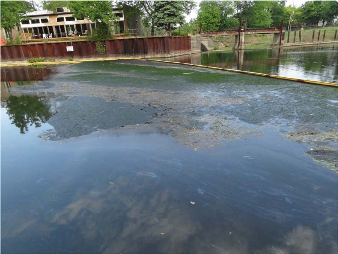
3. Ceresco Dam Control Point sheen and debris collecting.
