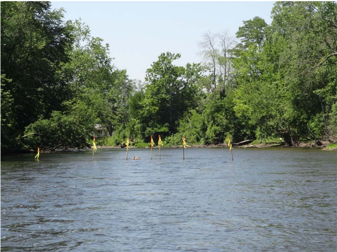
18. MP29.25 observed the navigational stakes reinstalled.
