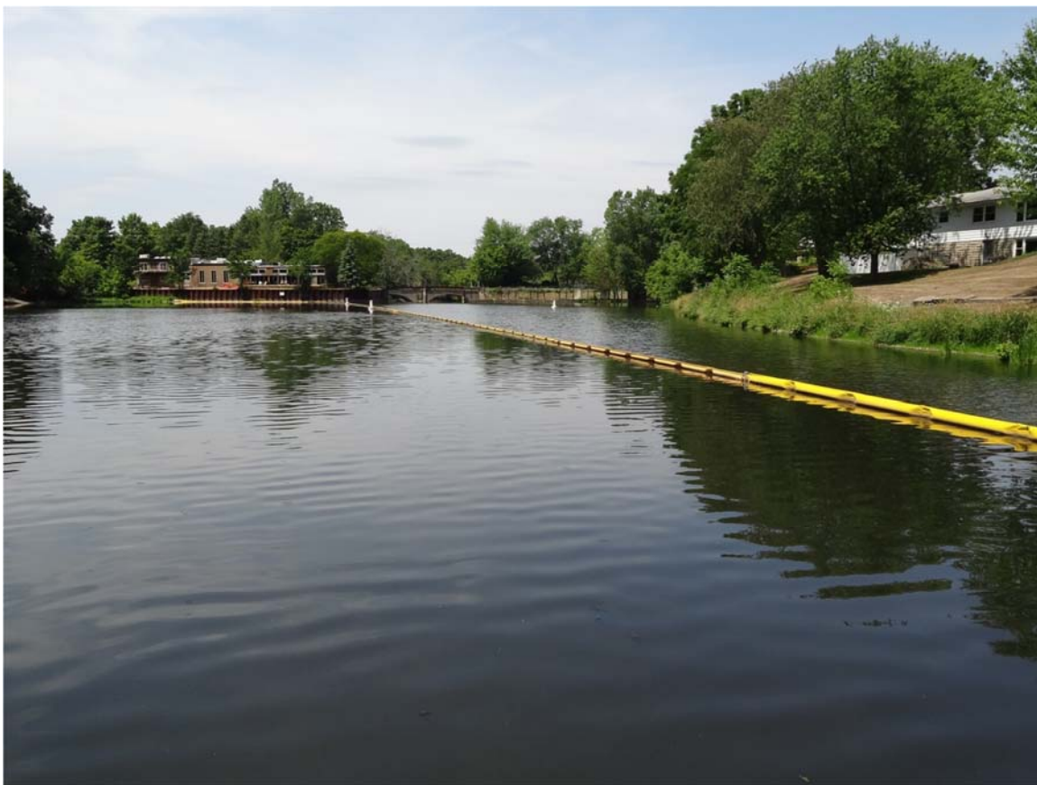
21. Ceresco Dam containment boom.
