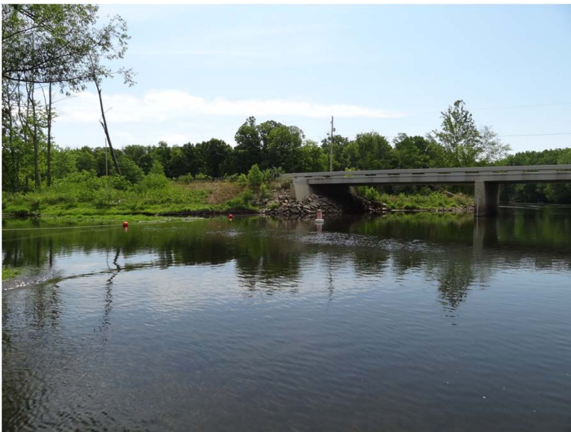
12. MP21.5 RDB no sheen observed.
