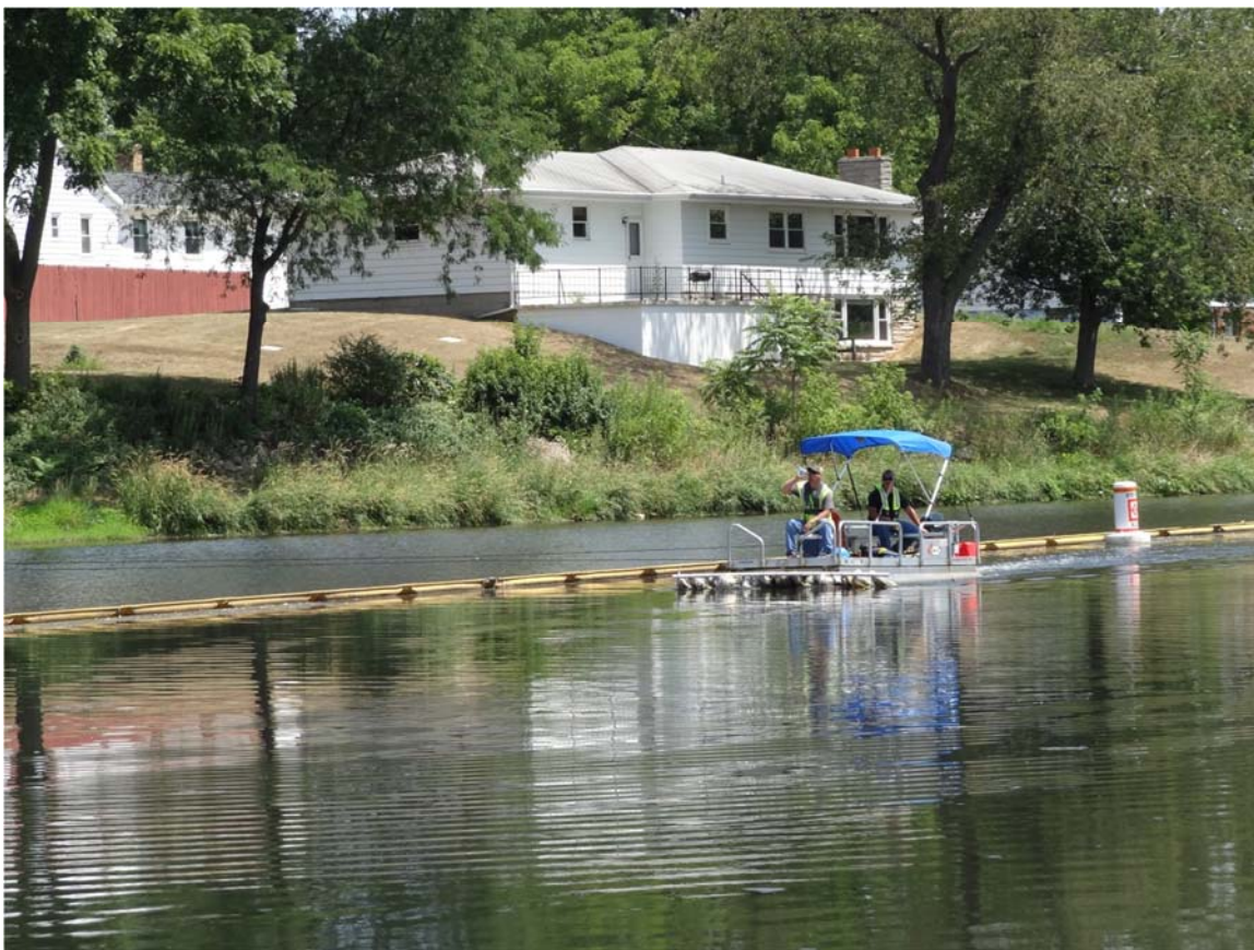
23. Ceresco Dam containment boom, observed the sweep boat operating.
