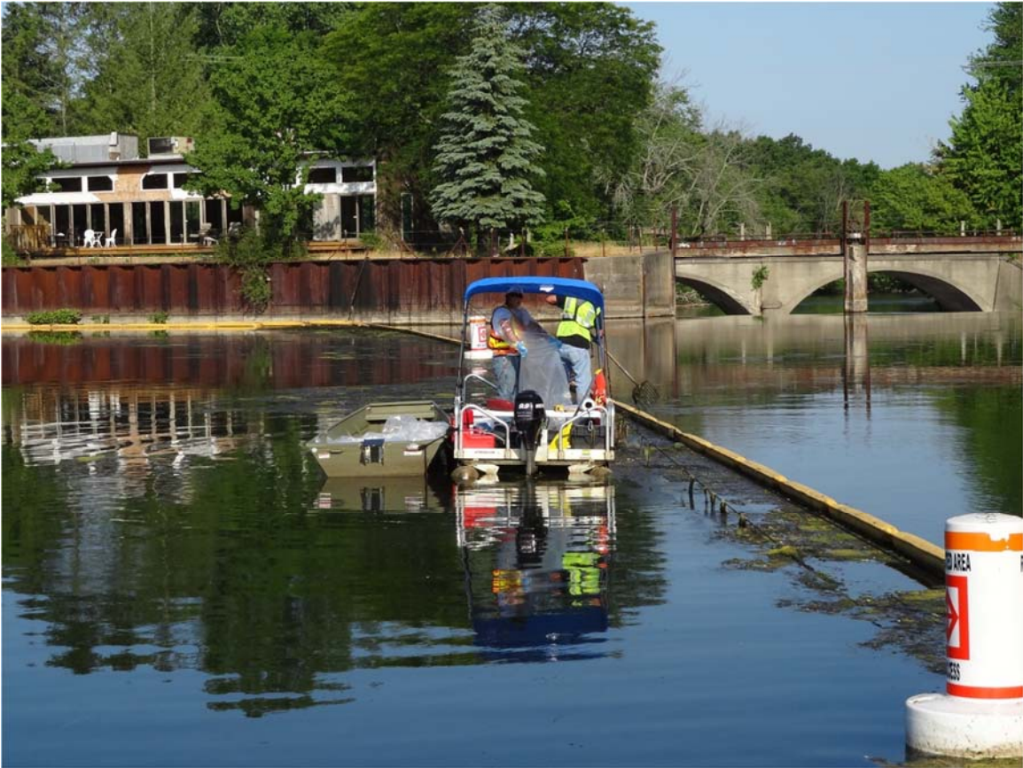
9. Ceresco Dam observed debris removal from the control point.
