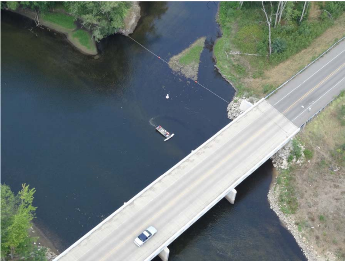
18. Sheen sweeper boat observed at MP 21.5.
