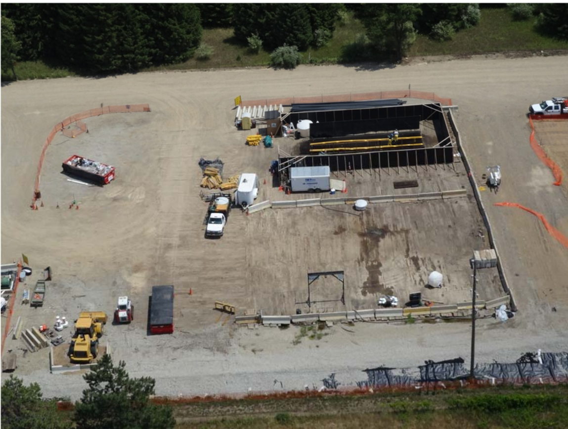
4. Frac-Tank City observed boom being decontaminated.
