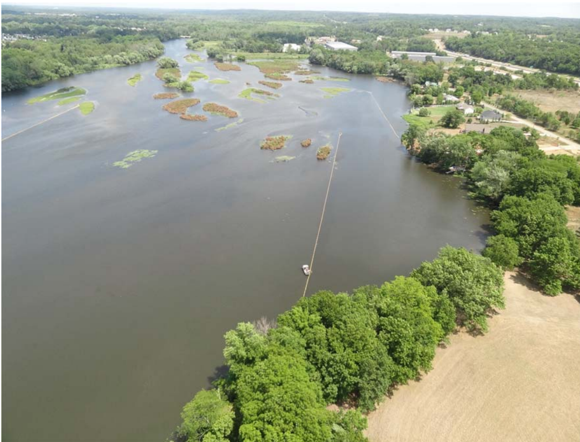
22. Morrow Lake Delta, observed boom maintenance along Boom B.
