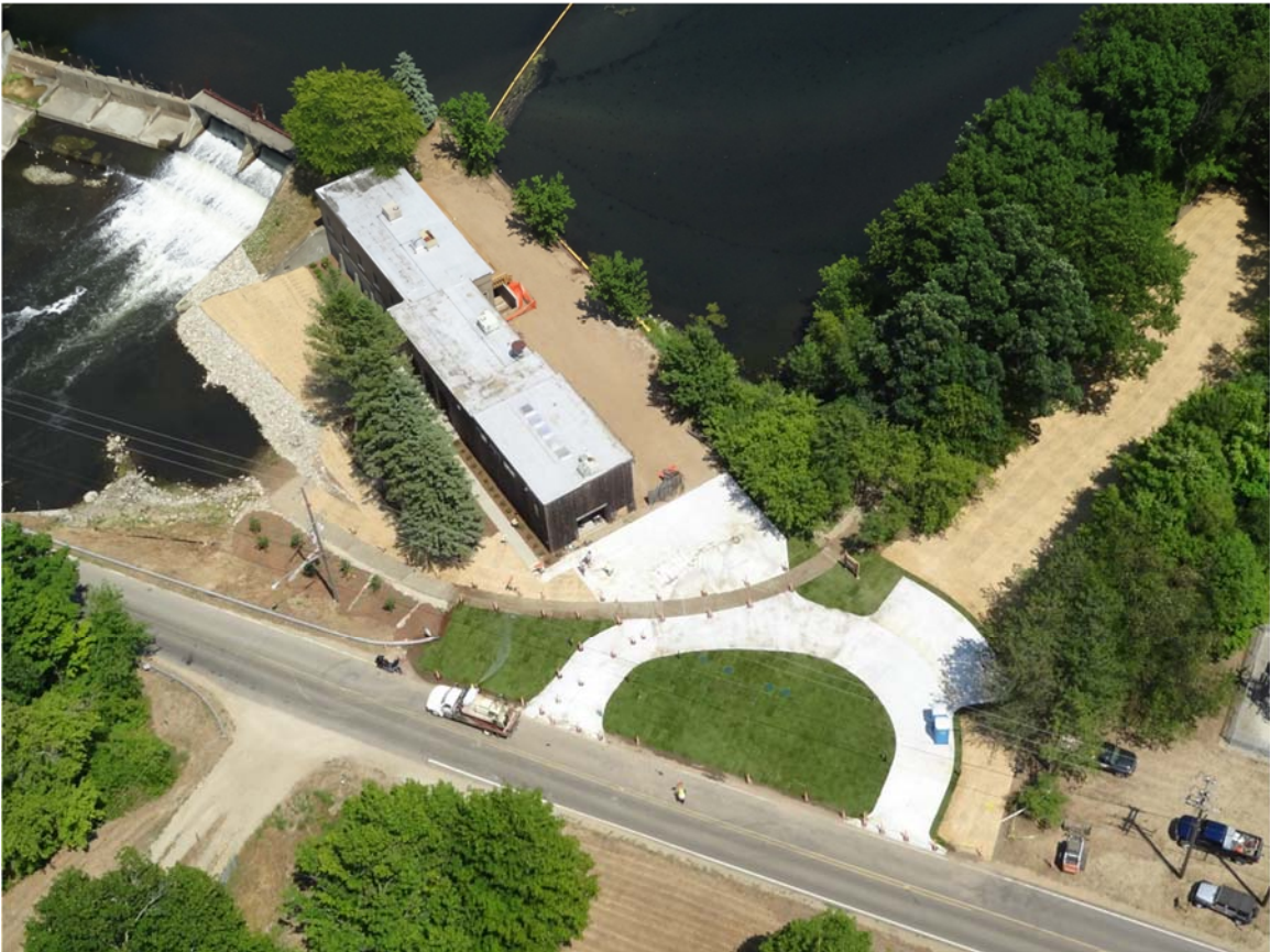
8. Ceresco Dam portage work.
