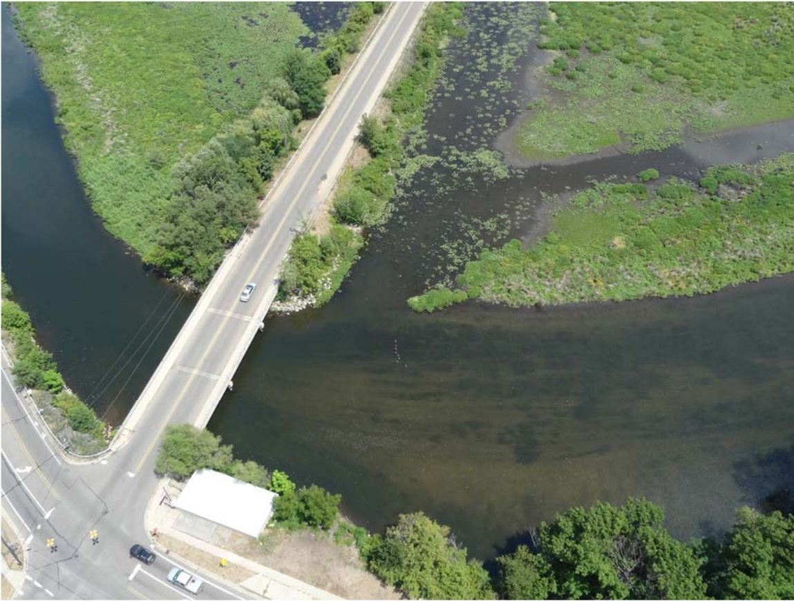
17. MP15.5 South Mill Pond, no sheen observed.
