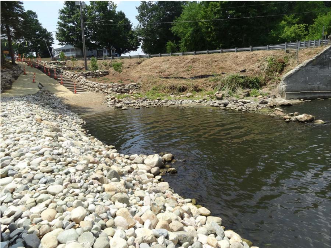
16. Ceresco Dam Portage work continued.
