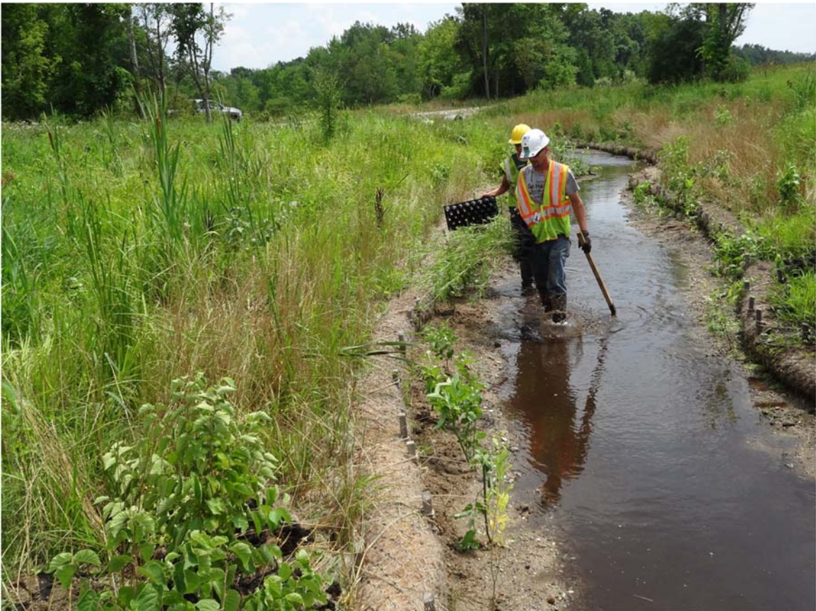
28. Talmadge Creek restoration work observed.
