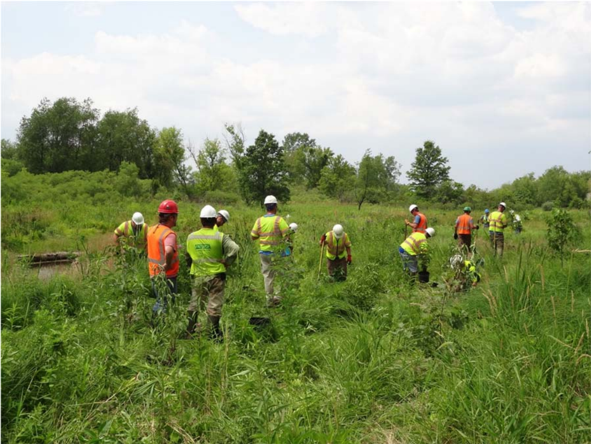
27. Talmadge Creek restoration work observed.
