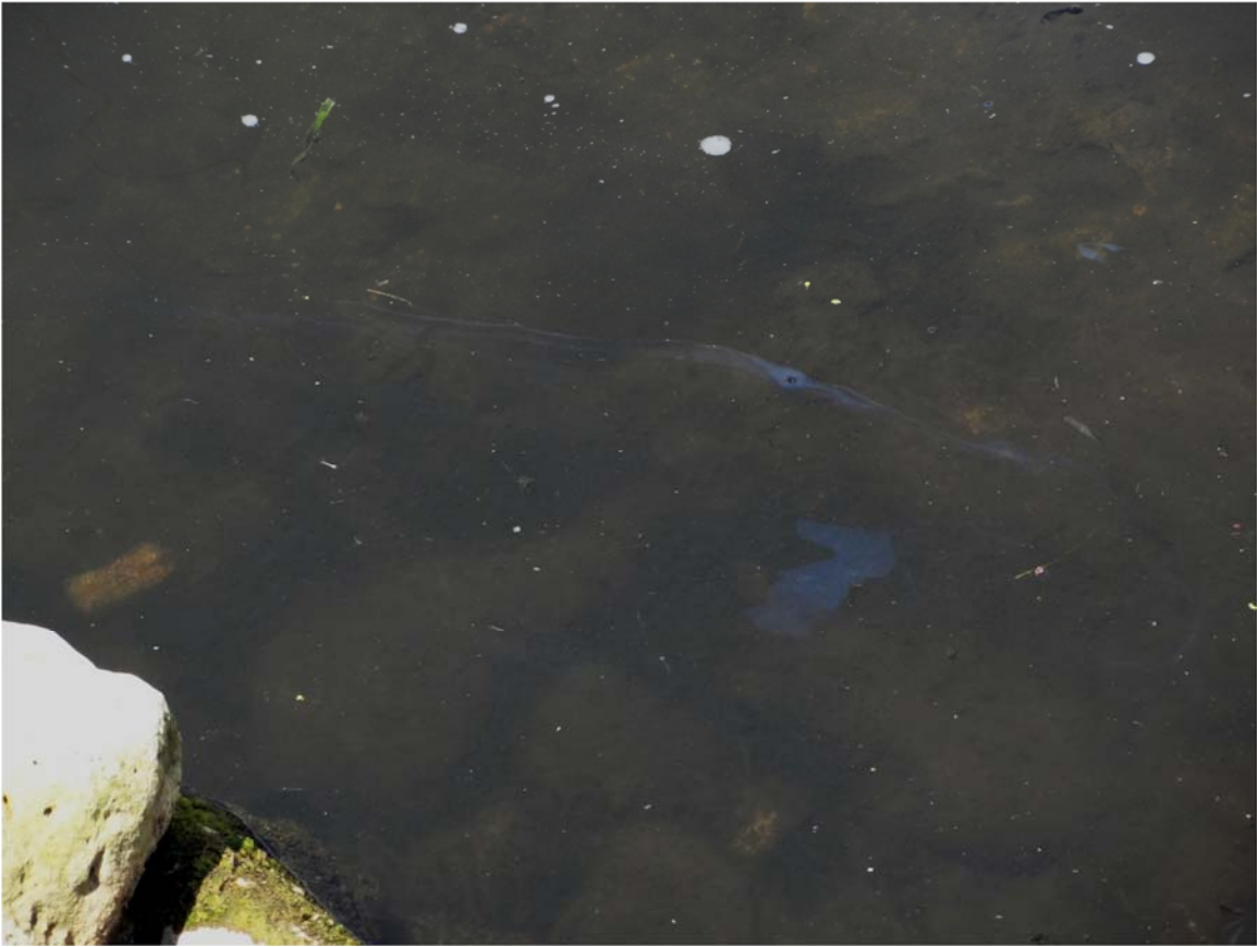
17. Ceresco Dam sheen observed within the downstream Portage cove.
