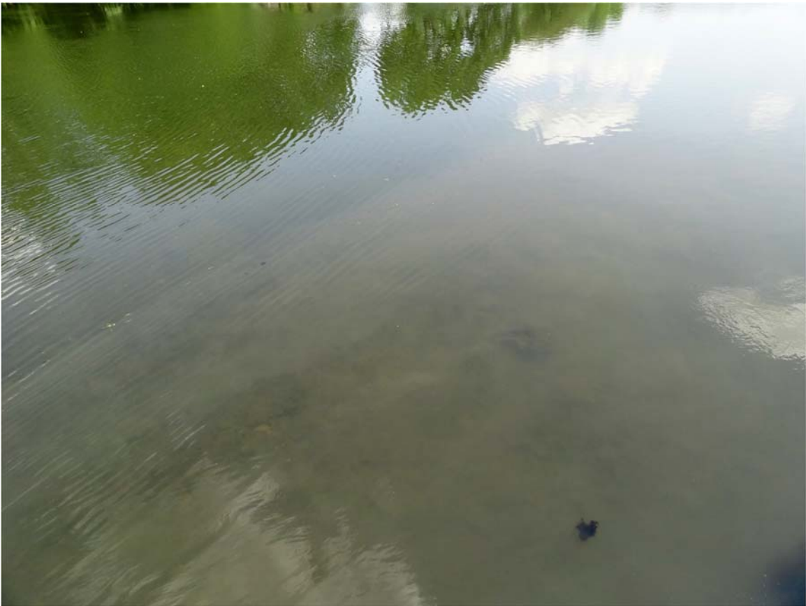
20. Ceresco Dam sediment plume observed going over the dam.
