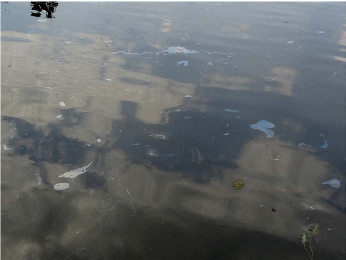
24. MP5.63 LDB Railroad Crossing sheen observed.
