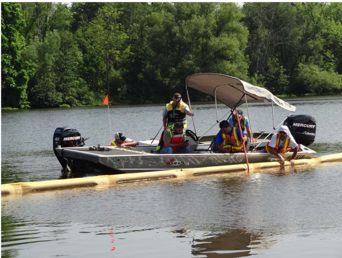
8. Morrow Lake Delta observed crew performing a video inspection of the containment curtain.
