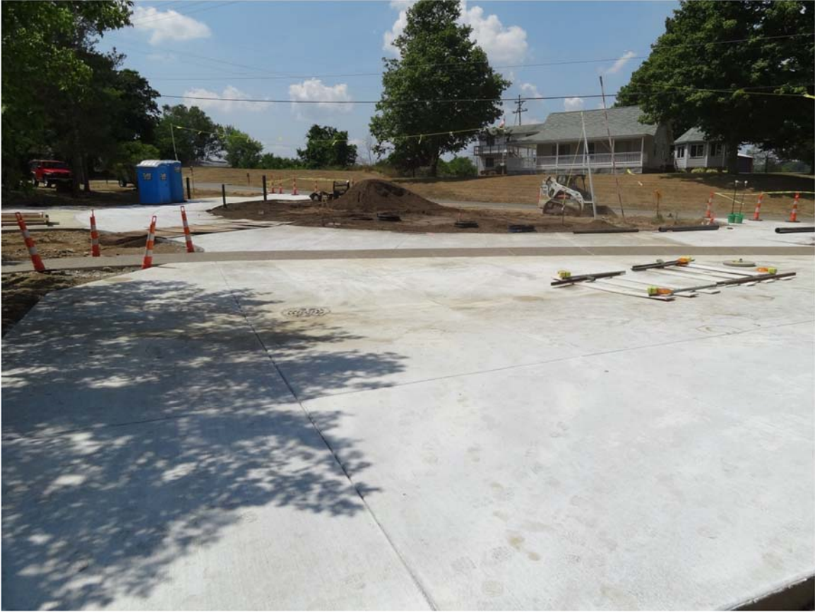
15. Ceresco Dam Portage work continued.
