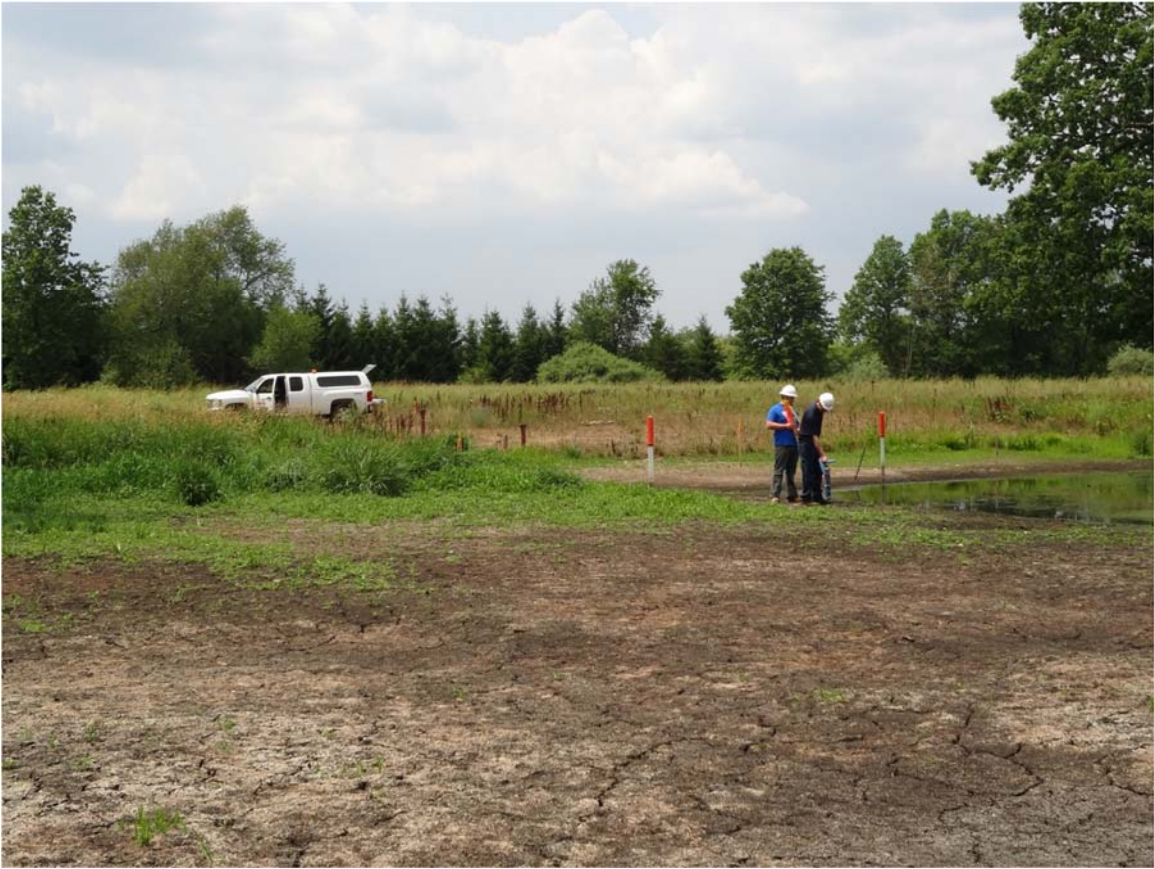
29. Source Area Pond observed crew locating and staking the pipeline.
