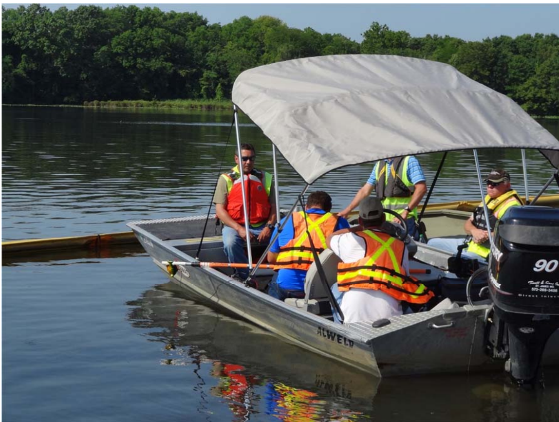
7. Morrow Lake Delta observed crew preparing to perform a video inspection of the containment curtain.
