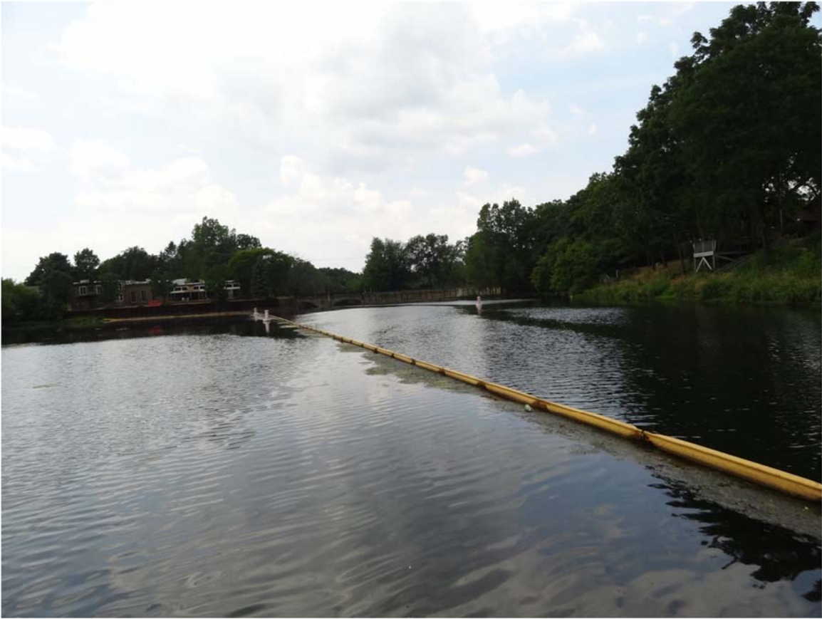
21. Ceresco Dam containment boom.
