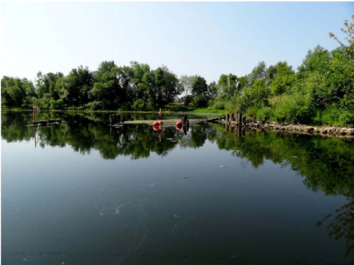
4. Sheen and vegetation observed at former trestle above Ceresco Dam.
