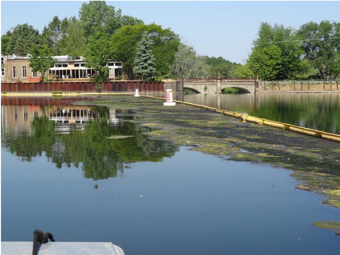
5. Vegetation and sheen observed along containment boom above Ceresco Dam.
