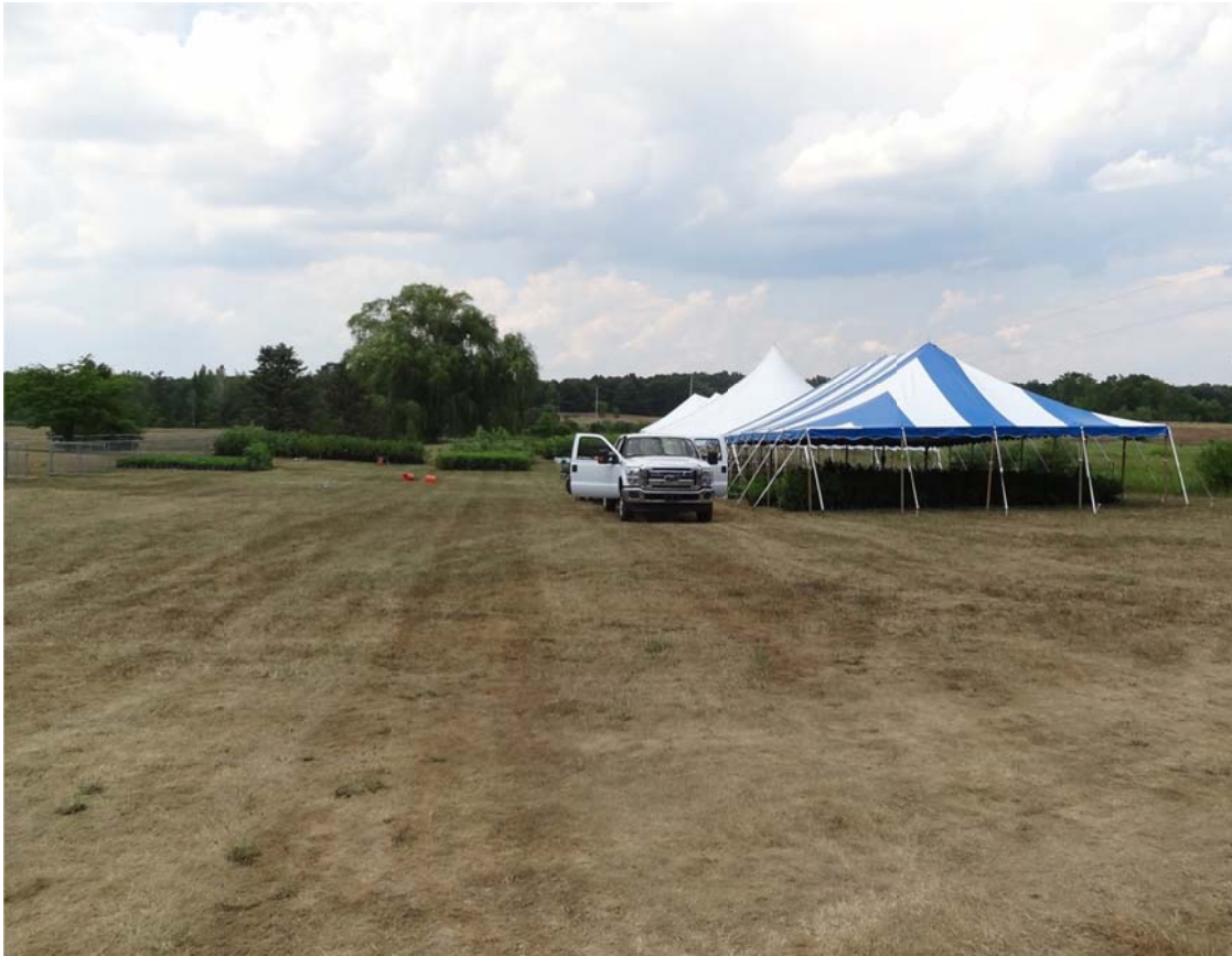
1. Plant staging area set up along Division Drive for Talmadge Creek tree planting activities.
