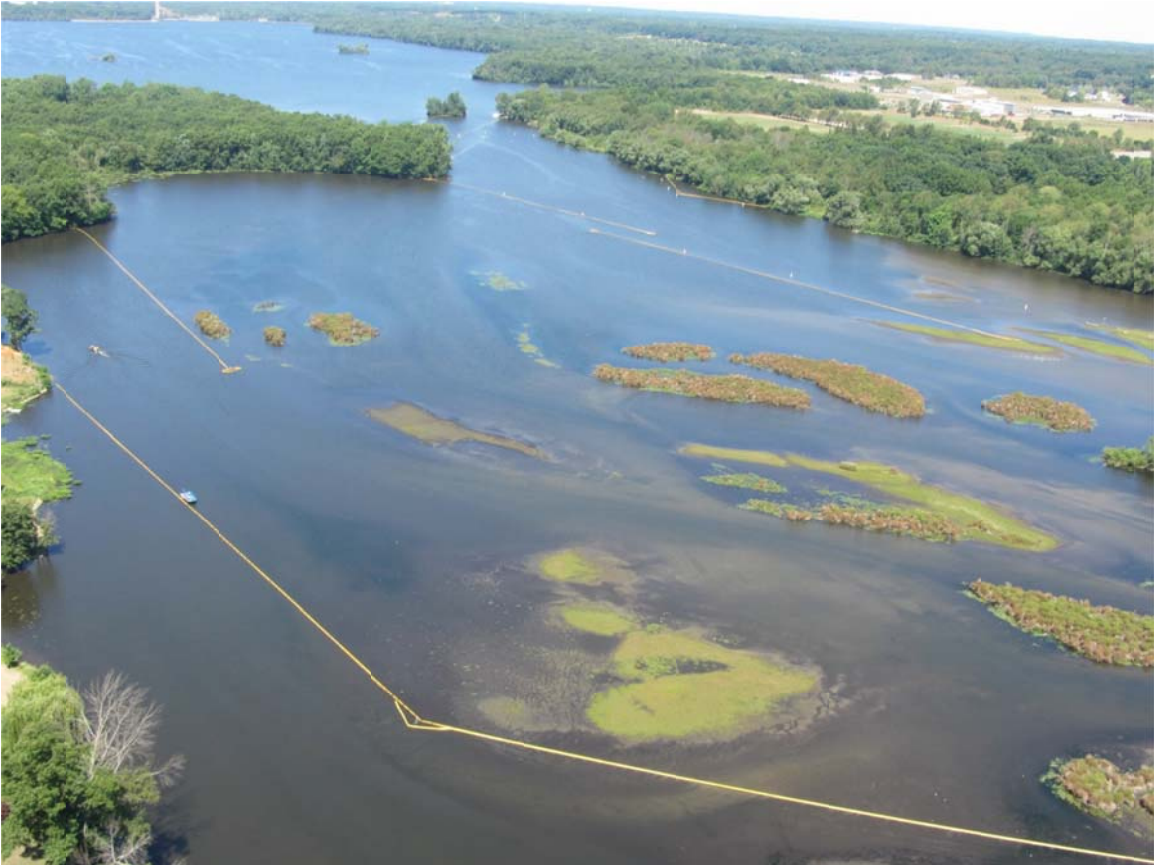
19. E 3.5 containment boom installed in southern end of Morrow Lake Delta.
