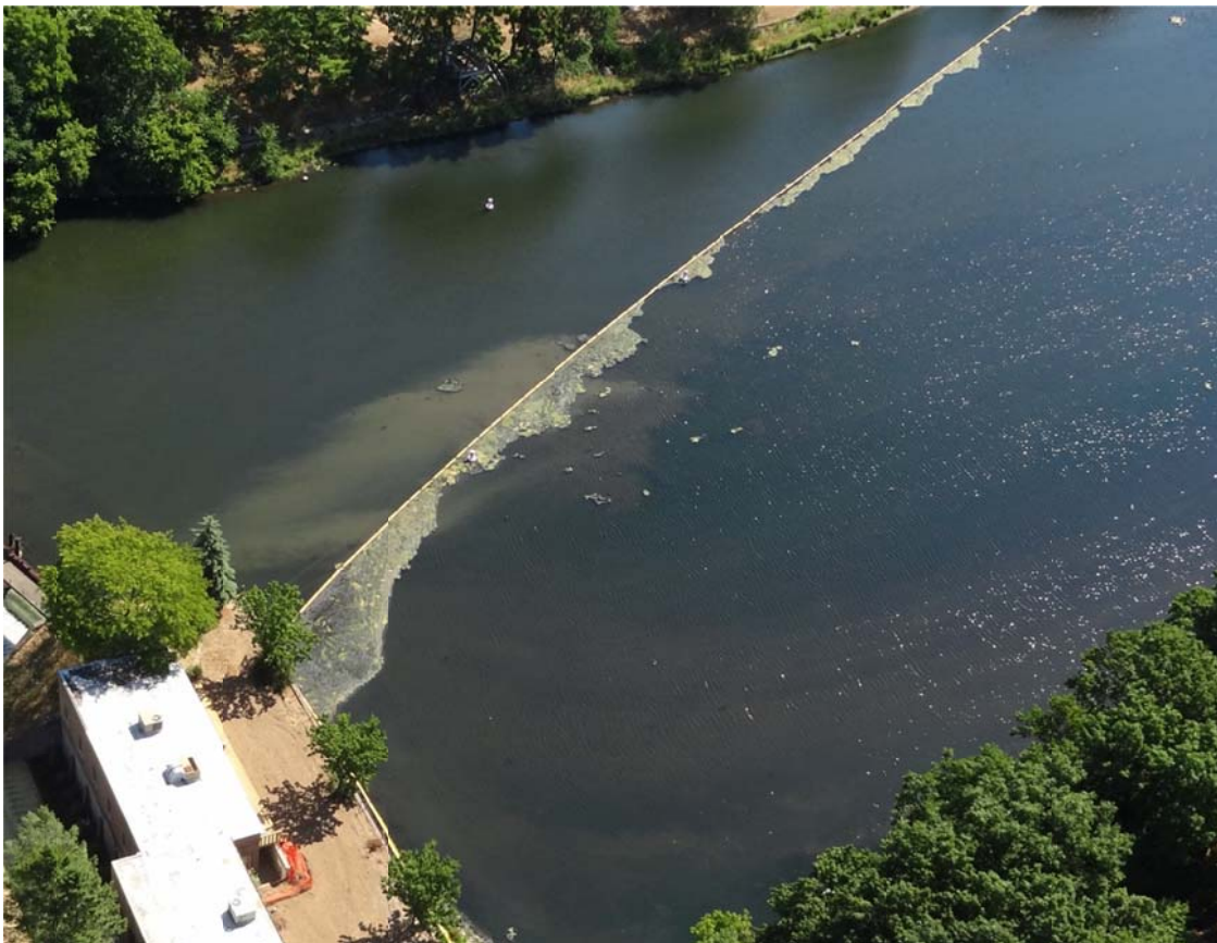
8. Vegetation and turbidity observed in vicinity of Ceresco Dam control point.
