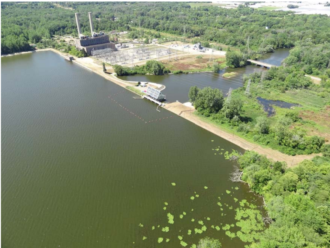
24. Morrow Lake Dam, no sheen or activity observed.
