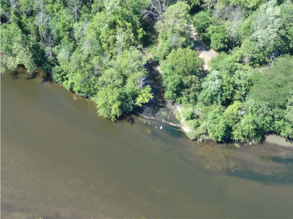
15. Downstream side of MP19.25 sediment trap, no sheen observed.
