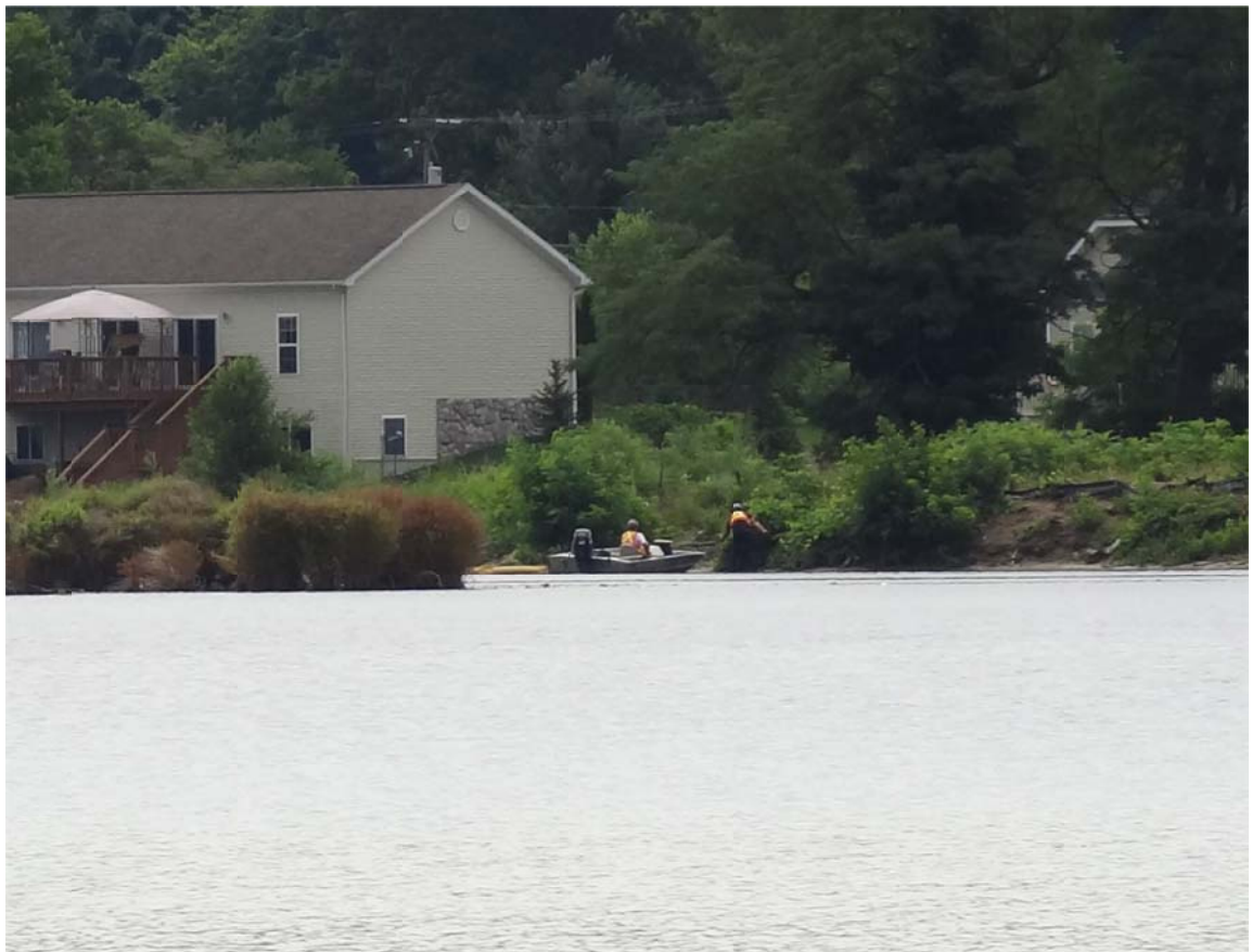
8. Crews installing containment boom in southern end of Morrow Lake Delta.
