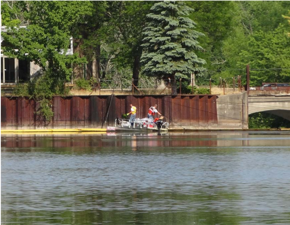
3. Crew maintaining containment boom above Ceresco Dam.
