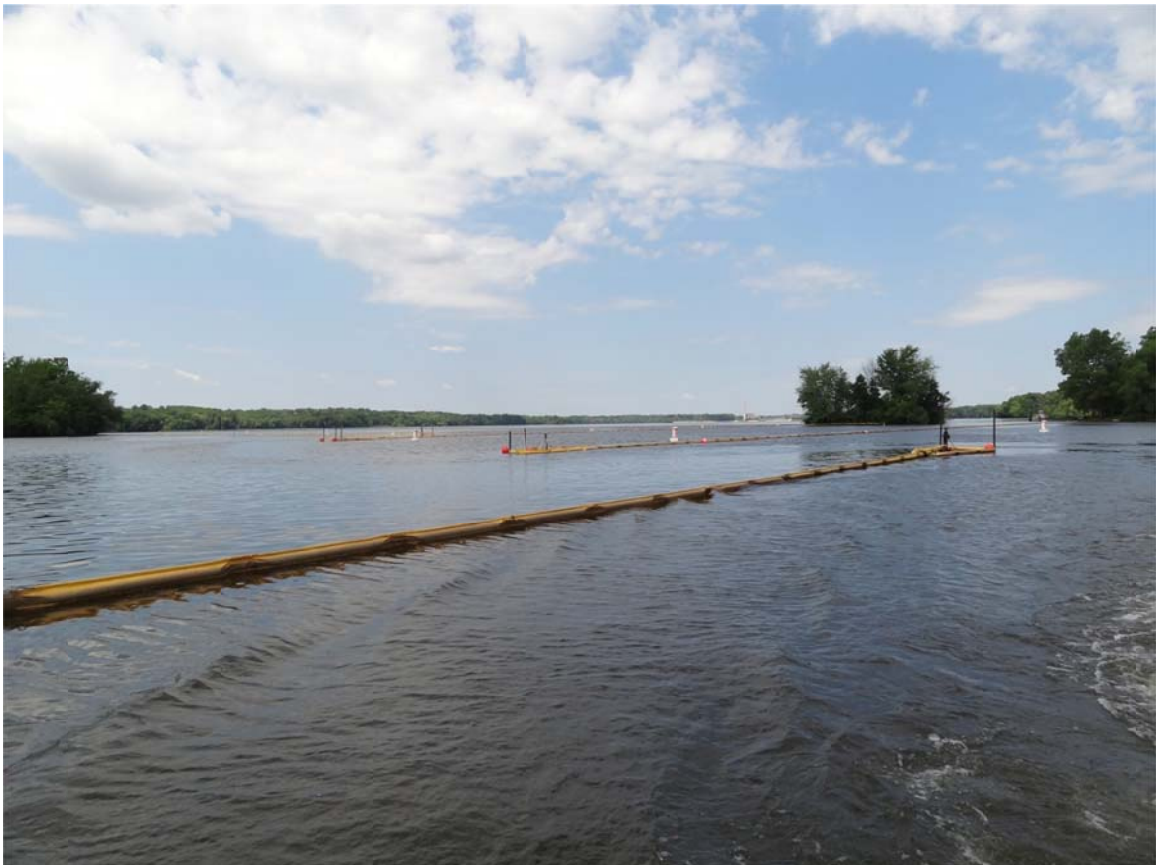
10. Control Point E4 gate boom configuration, looking west into mouth of Morrow Lake.
