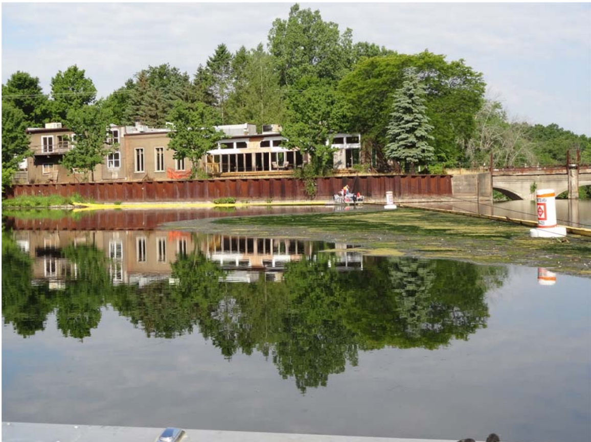
2. Crew removing vegetation from control point above Ceresco Dam.
