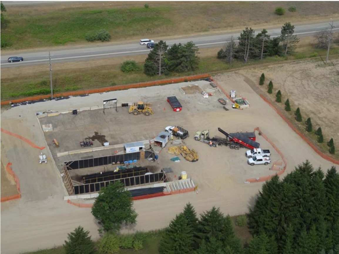
2. Frac-City, observed crews cleaning boom in the decon pad.
