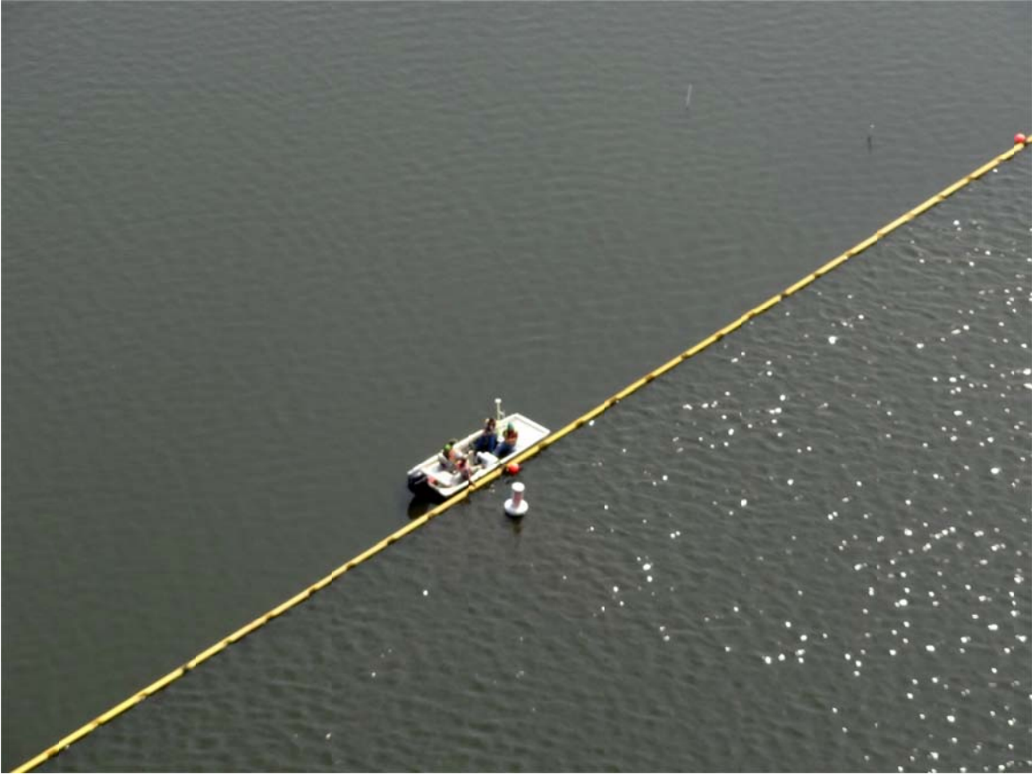
17. Crews inspecting the curtain along the E4 Boom System.
