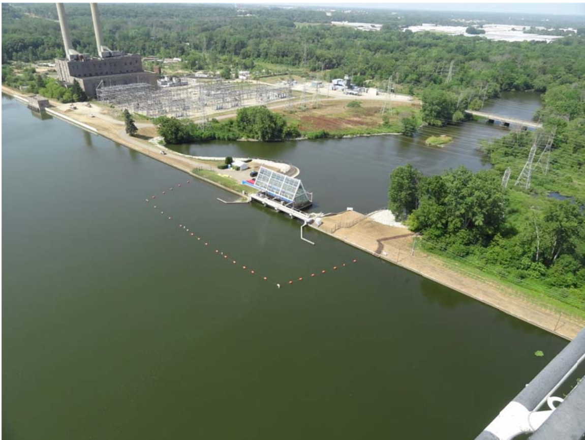
22. Morrow Lake Dam, no sheen observed.
