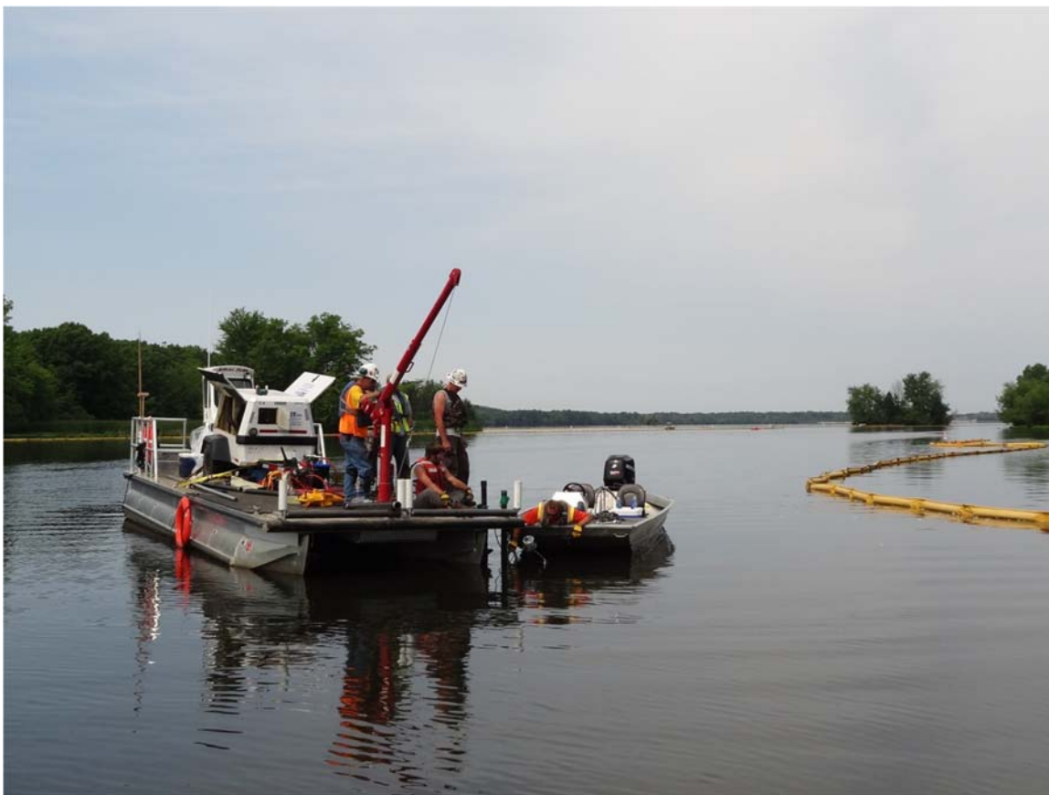
15. Morrow Lake Delta E4 boom system anchor installation.
