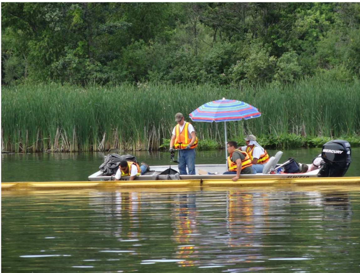
19. Morrow Lake Delta E4 boom system, observed crew installing curtain.
