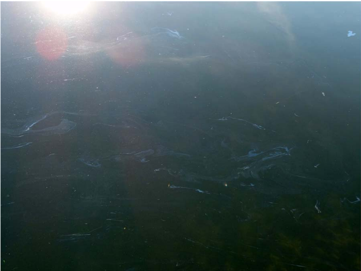
2. Ceresco Dam sheen observed above the dam. Operations was notified.
