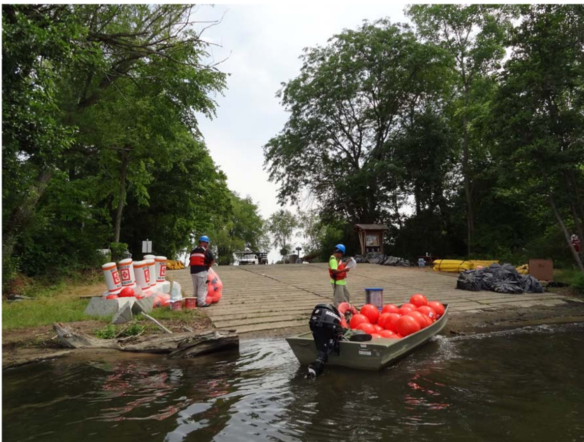
20. Morrow Lake Delta E4 boom system, observed crew deploying buoys.
