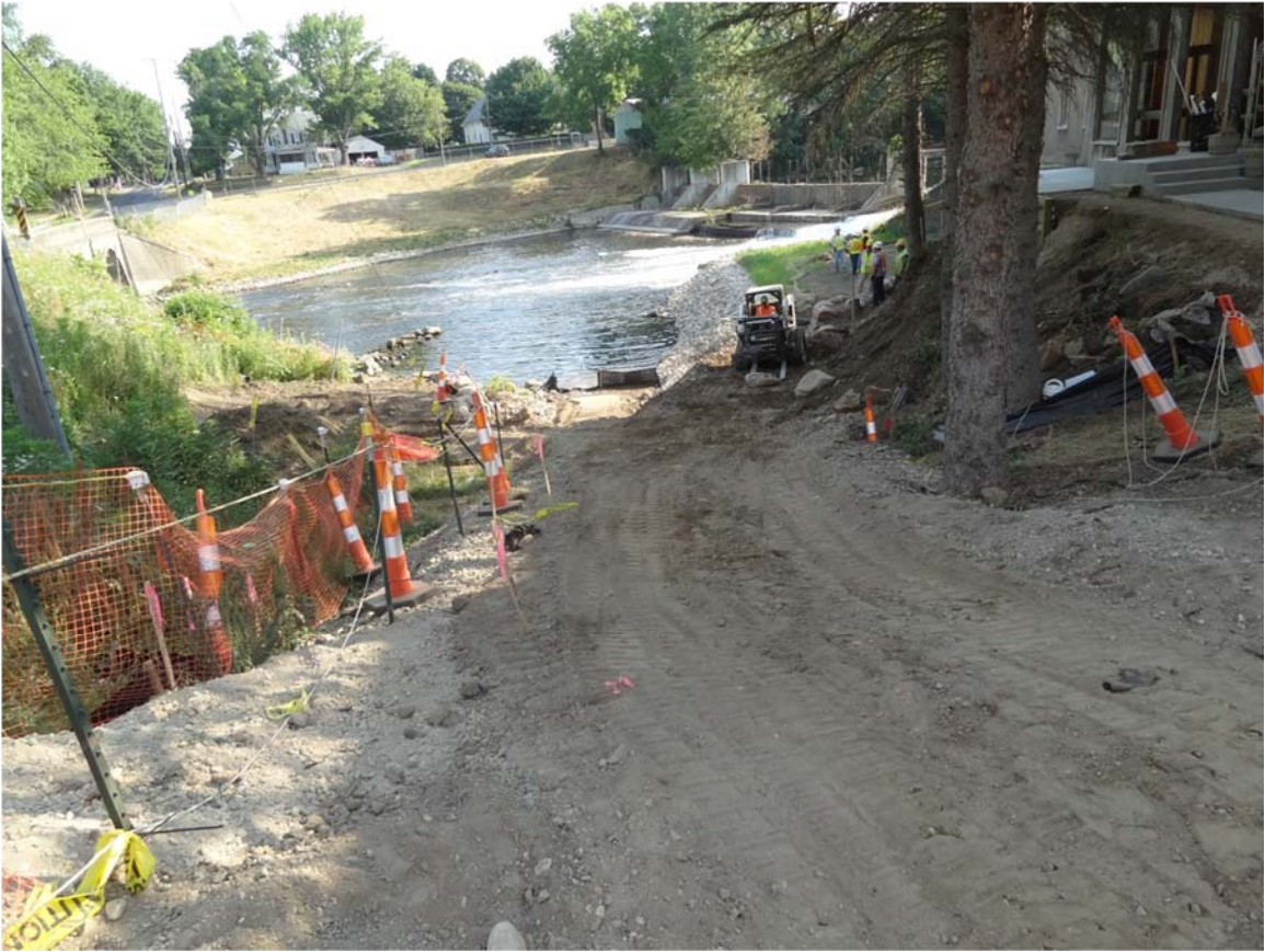
1. Ceresco Dam portage work continued below the dam.
