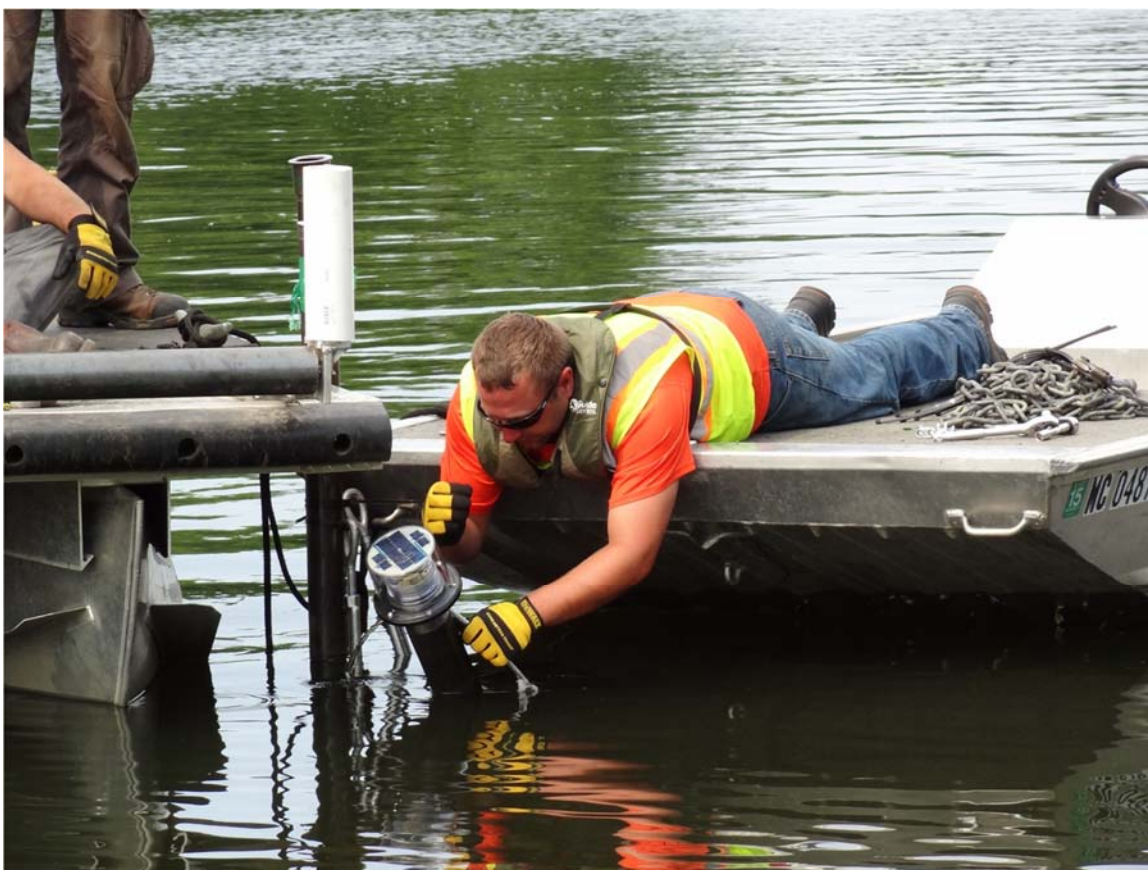
16. Morrow Lake Delta E4 boom system anchor installation, observed crew fixing broken anchor.
