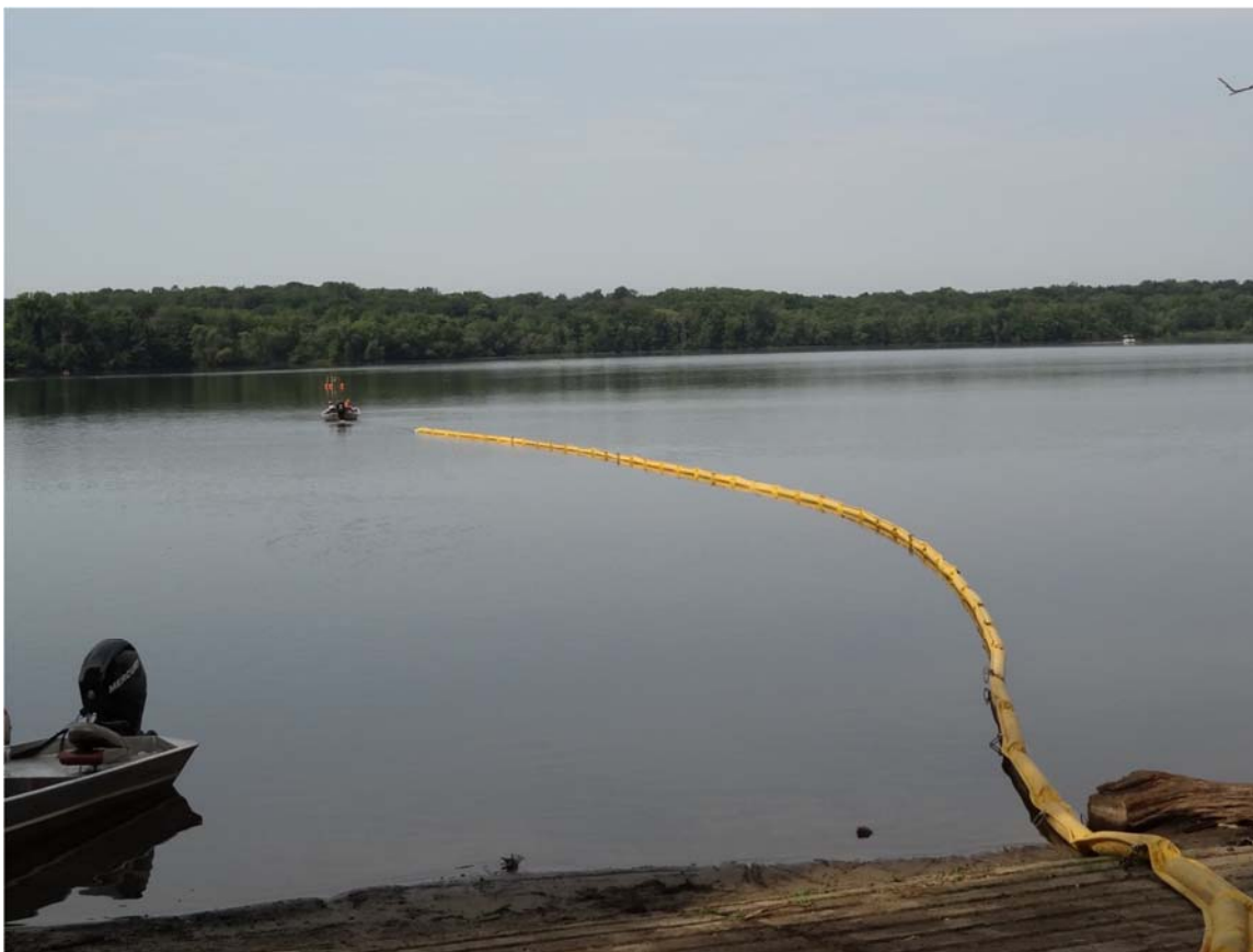
12. MP37.75 Observed crews deploying boom from E4 boat launch.
