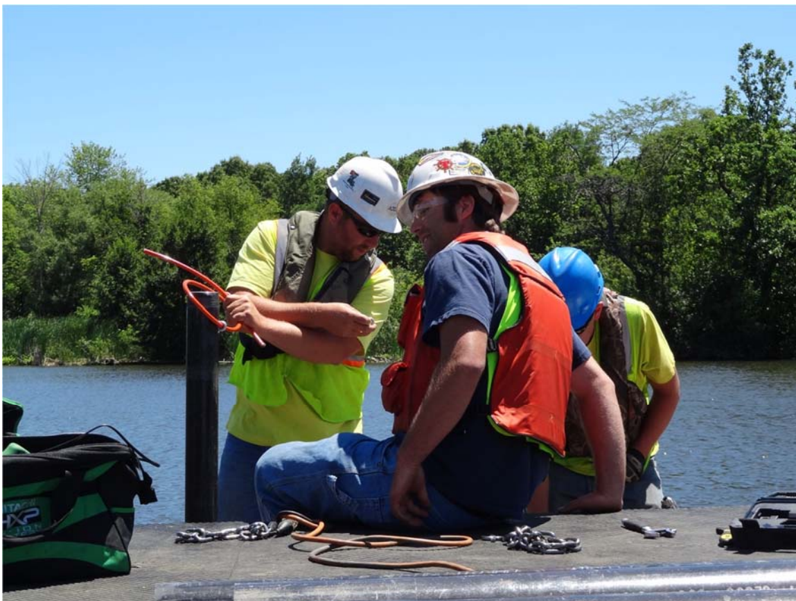
5. Observed installation of anchors for the new containment structures within the Morrow Lake Delta.
