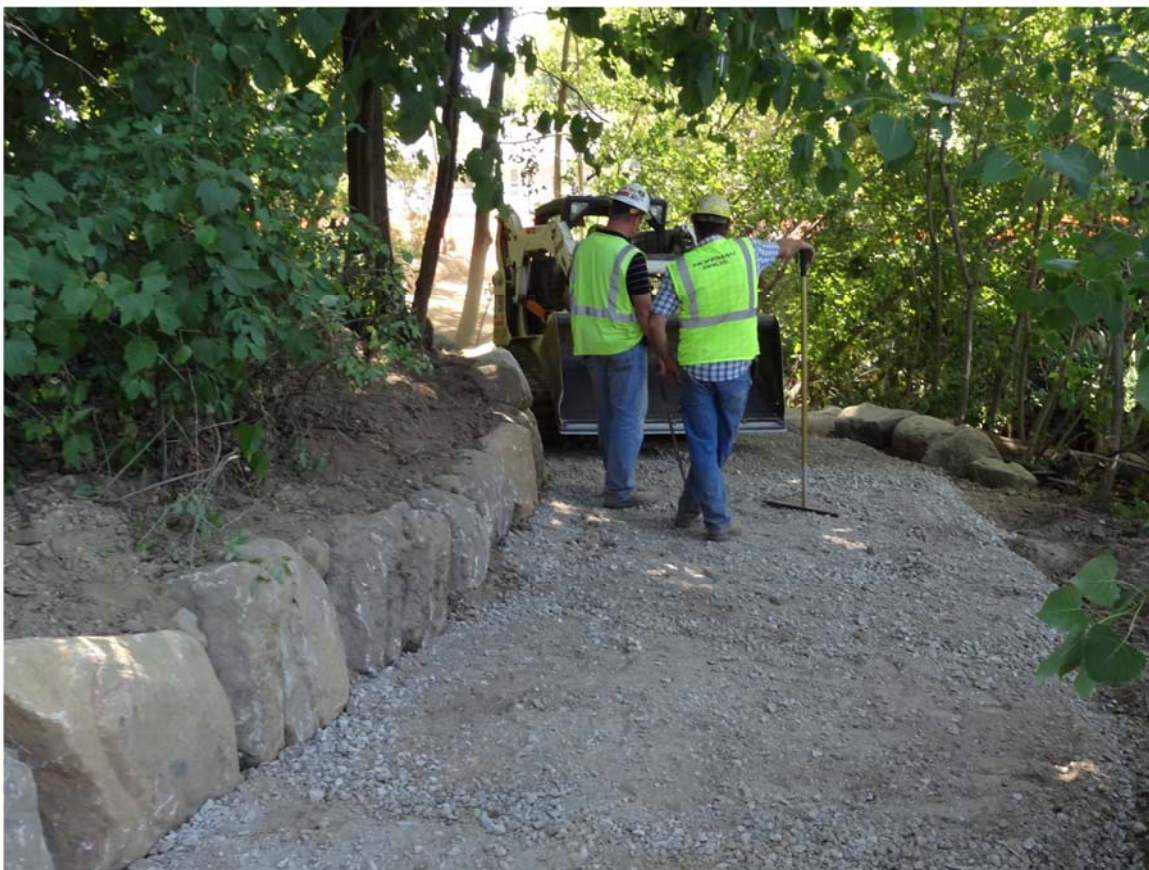
15. Ceresco Dam portage work continued.
