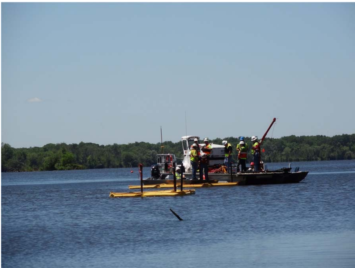
3. Observed installation of anchors for the new containment structures within the Morrow Lake Delta.
