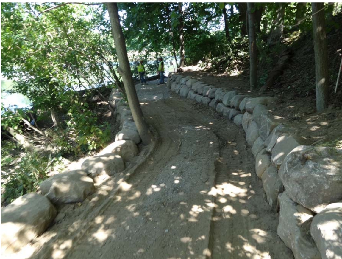
14. Ceresco Dam portage work continued.
