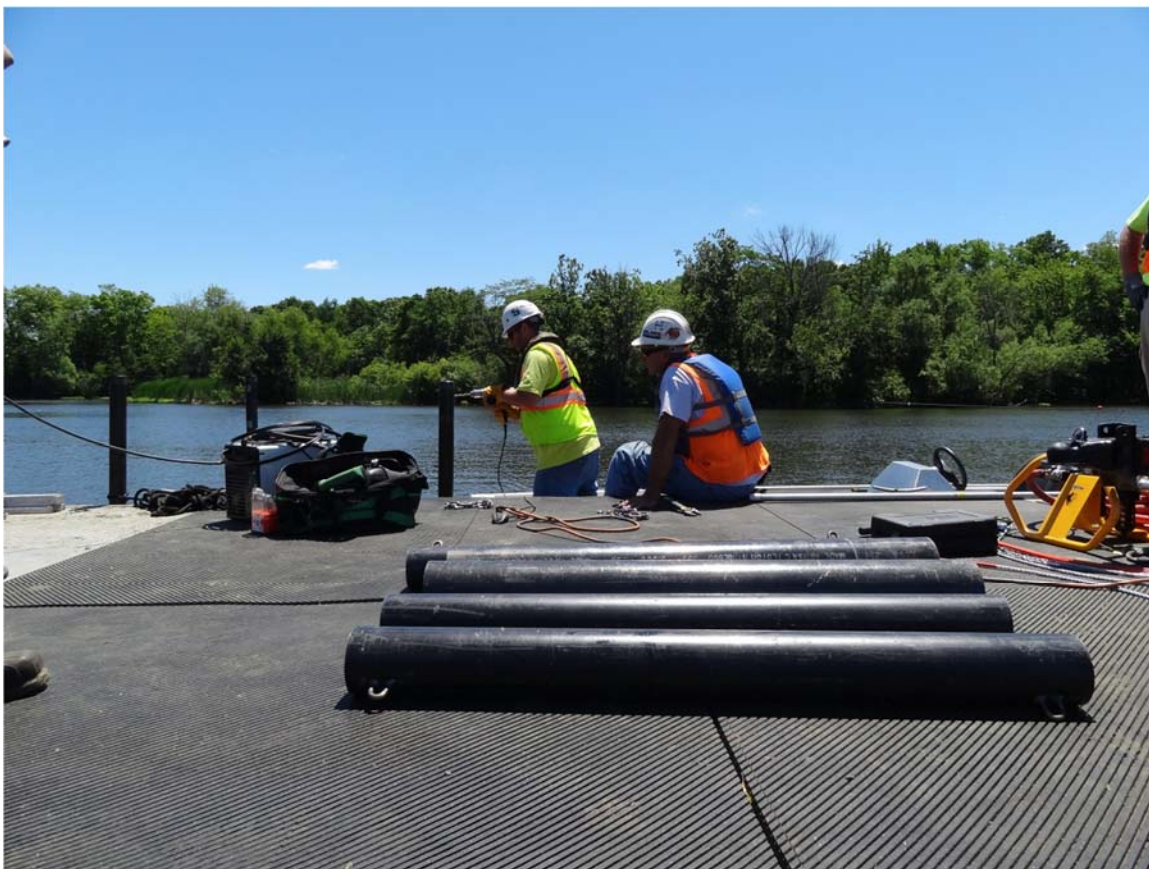
4. Observed installation of anchors for the new containment structures within the Morrow Lake Delta.
