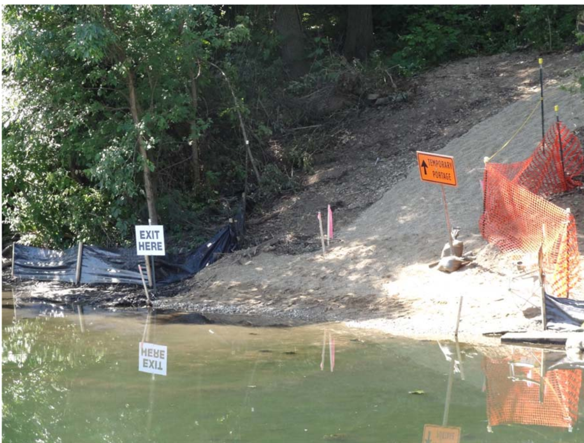
3. Ceresco Dam temporary portage.
