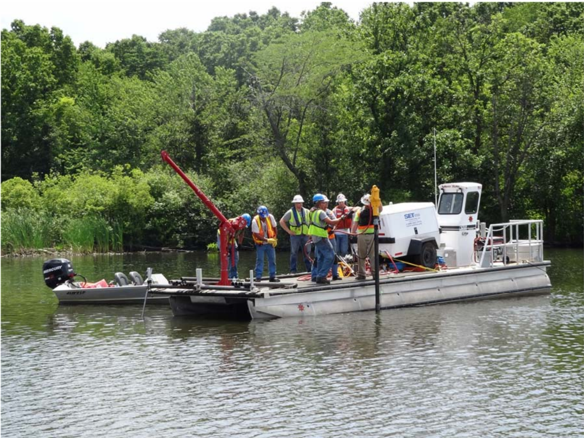
14. Morrow Lake Delta observed crew installing boom anchors.
