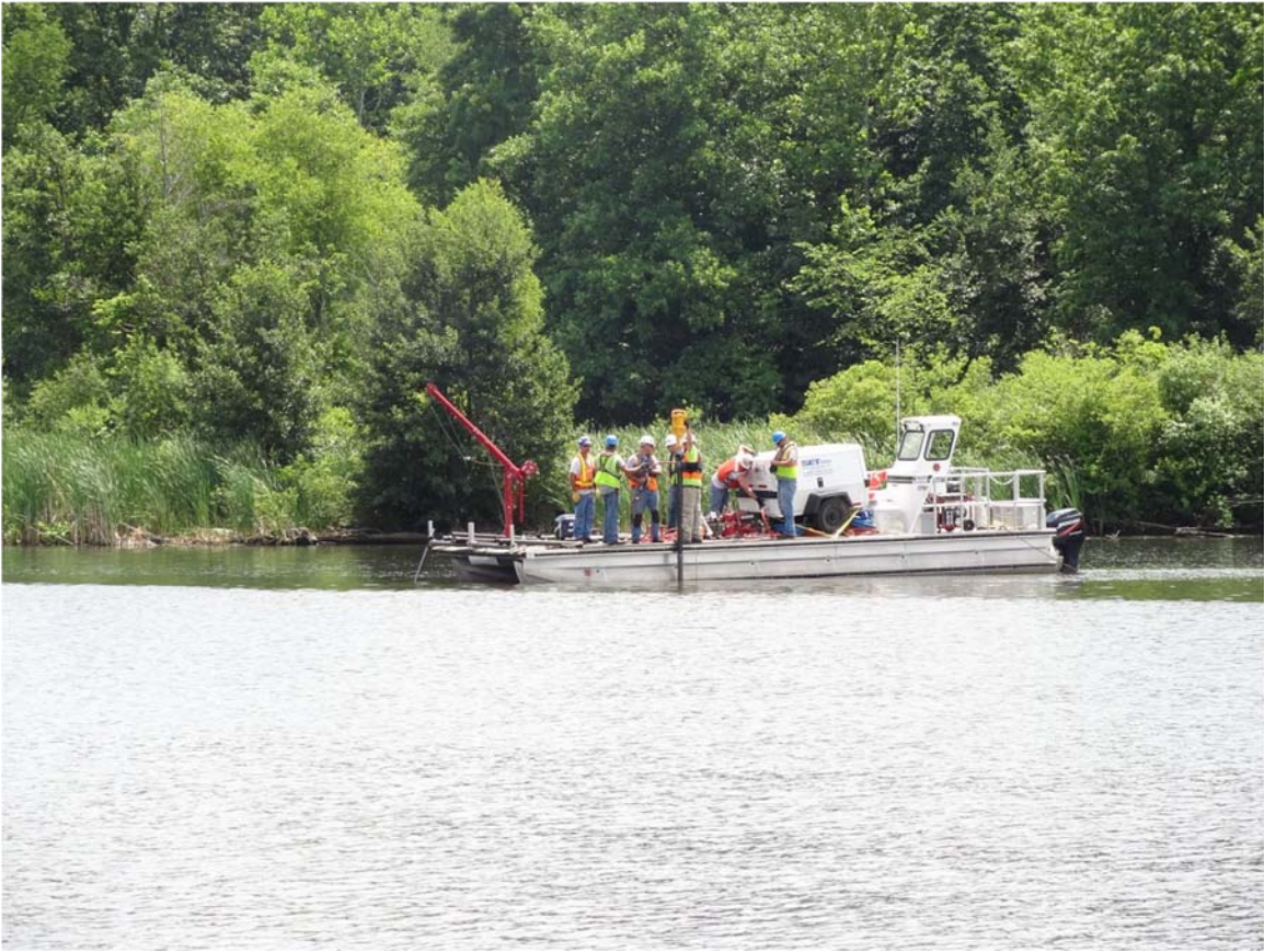
13. Morrow Lake Delta observed crew installing boom anchors.
