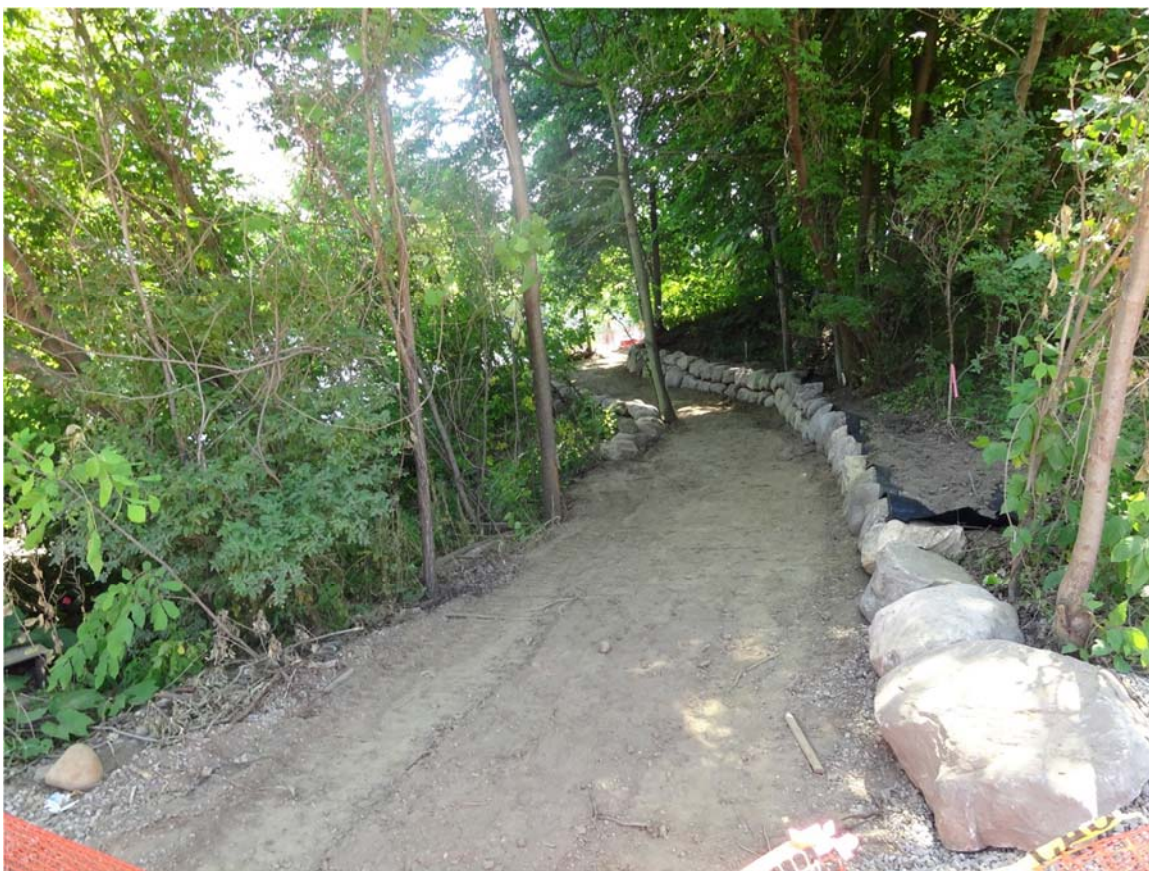
4. Ceresco Dam Portage under construction.
