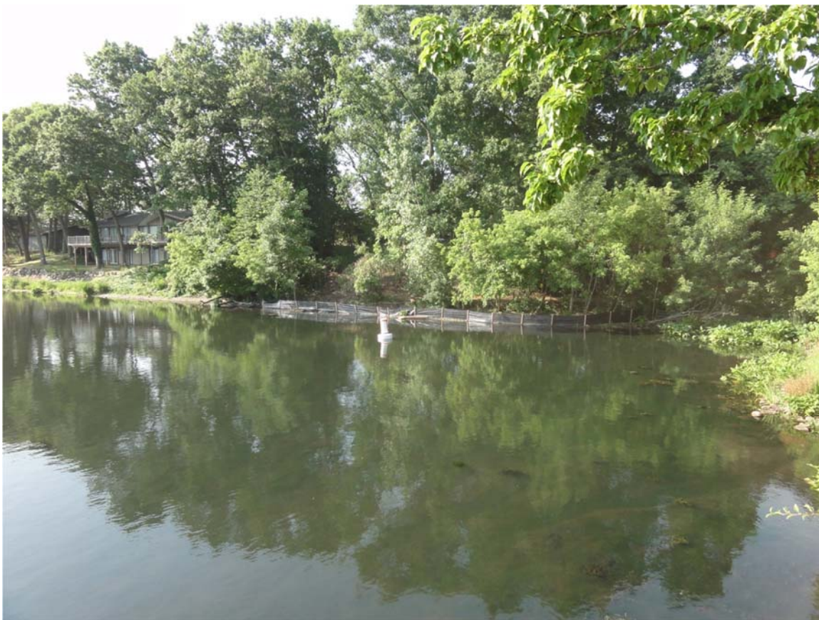
11. Ceresco Dam portage work continued.
