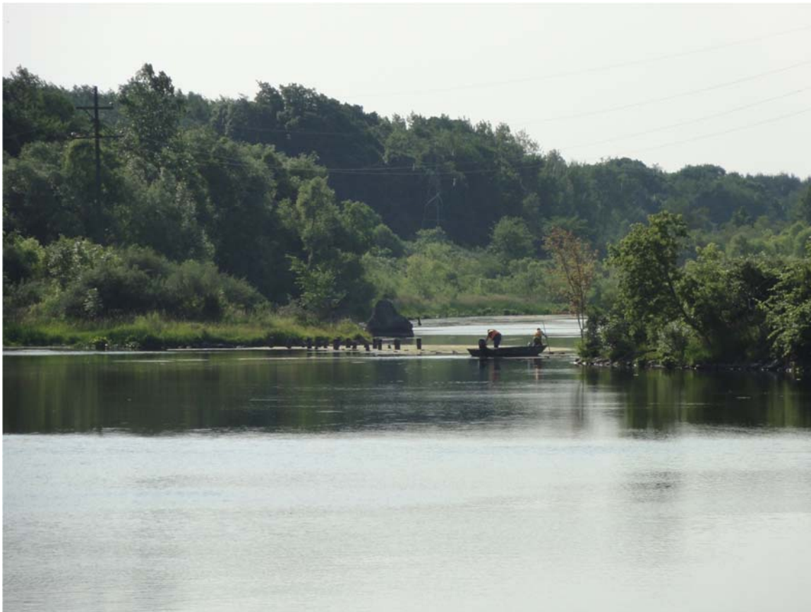
7. MP5.63 Observed crew removing vegetation.
