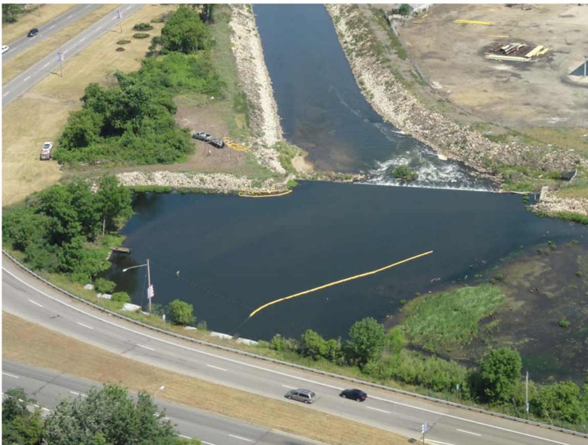
21. MP15.75 Boom observed being removed.
