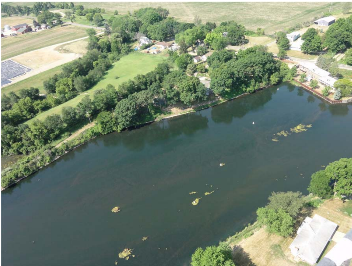
6. Ceresco Dam boom has been removed.
