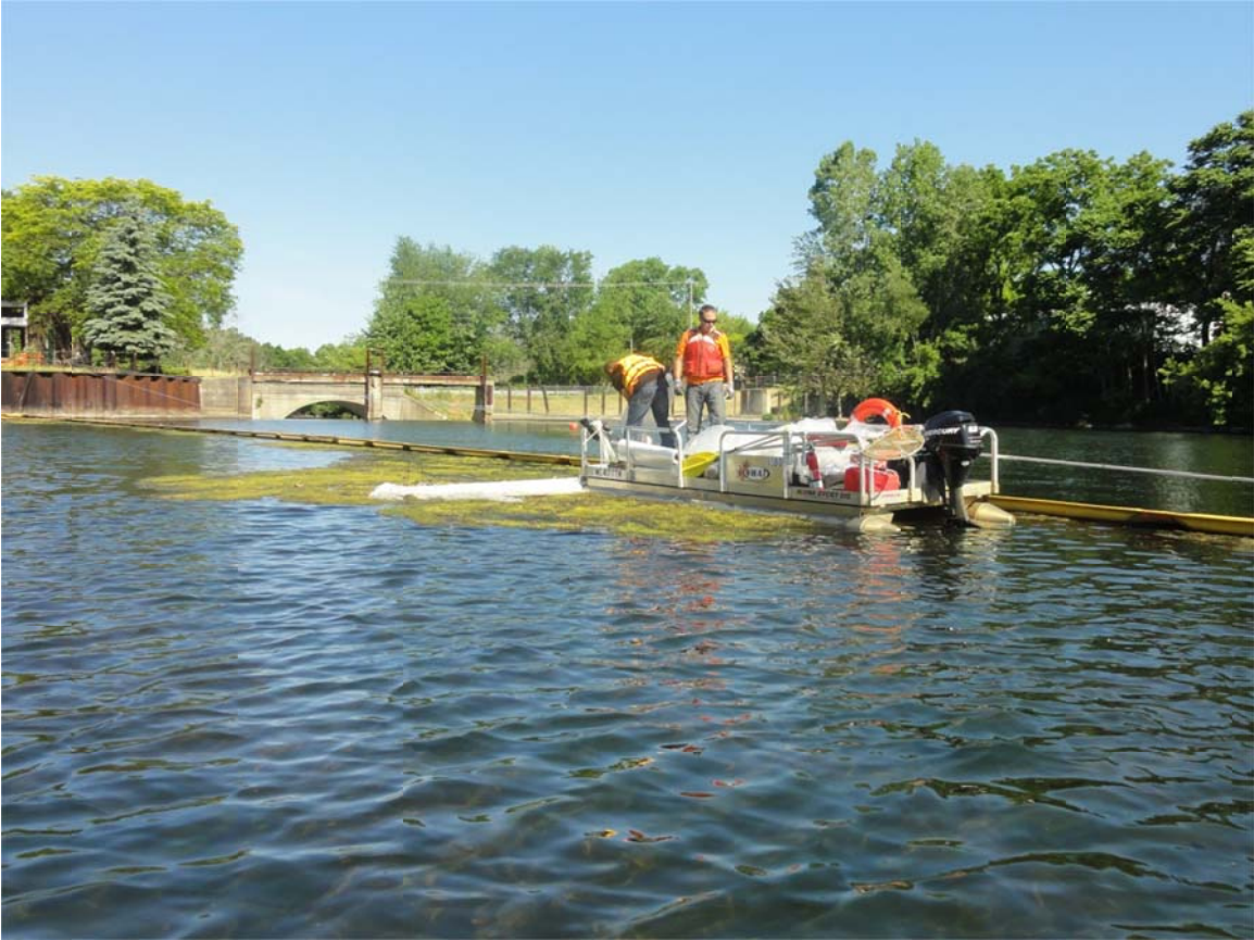
7. Debris removal along control point above Ceresco Dam.
