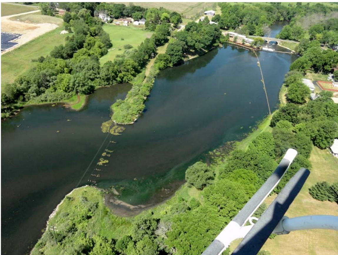
6. Ceresco Dam, boom maintenance crew observed.
