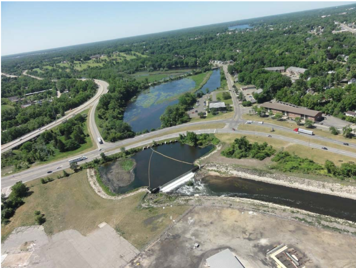
13. Battle Creek Spillway and Mill Ponds. No sheen observed.
