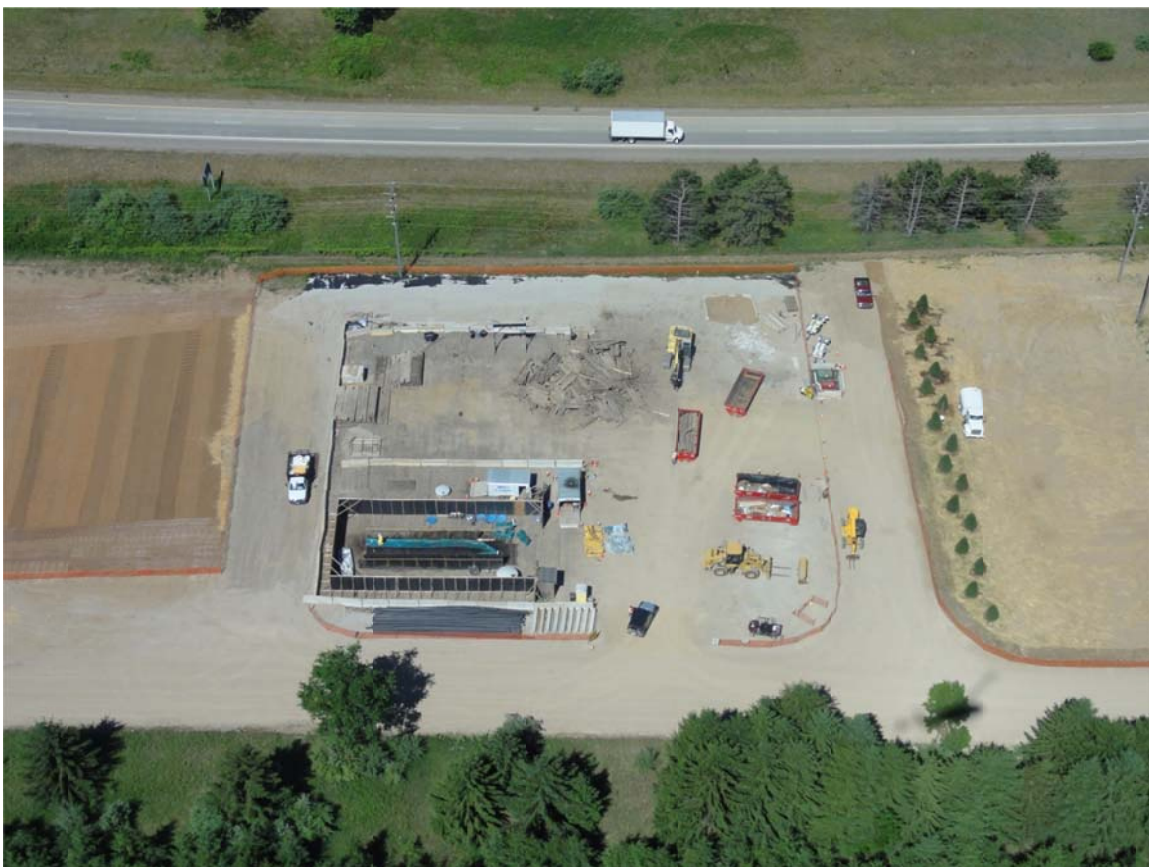
2. Frac-Tank City, observed the timber mats being disposed of.
