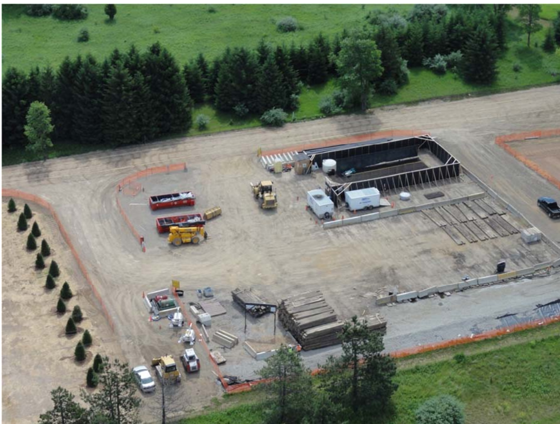
4. Frac-Tank City, no decontamination activities observed.
