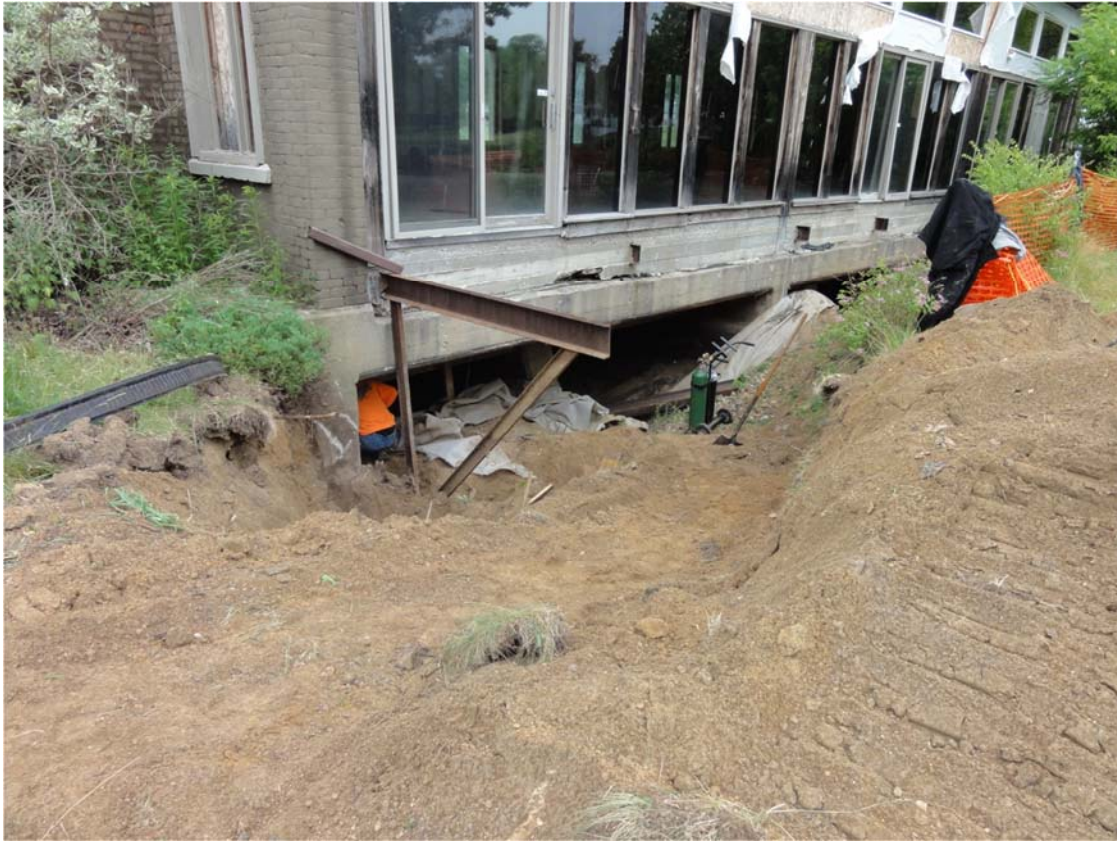
21. Ceresco Dam, owner is having turbines removed.
