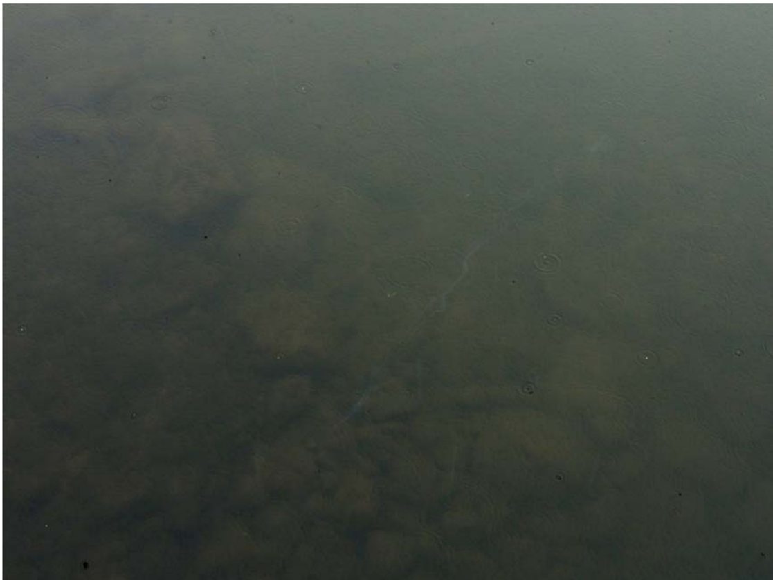
20. Ceresco Dam sheen observed flow over dam.
