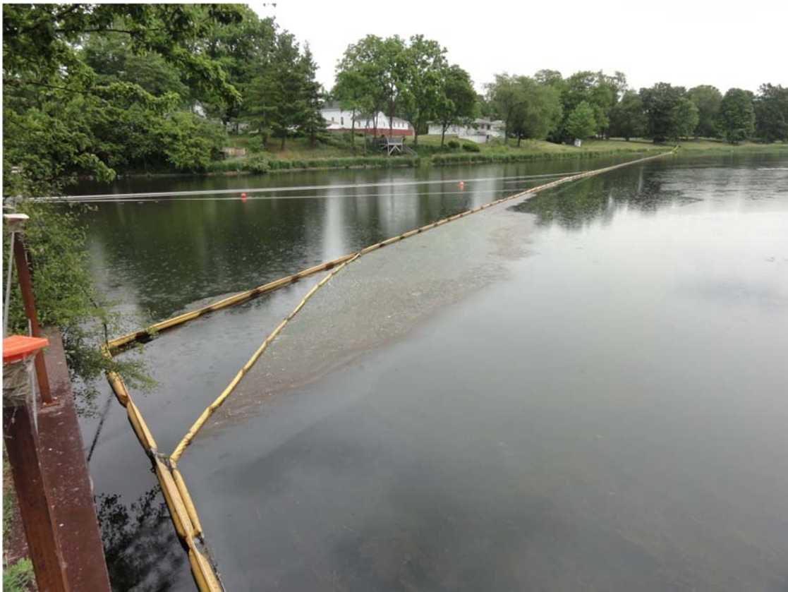
14. Ceresco Dam sheen and debris collecting at boom.
