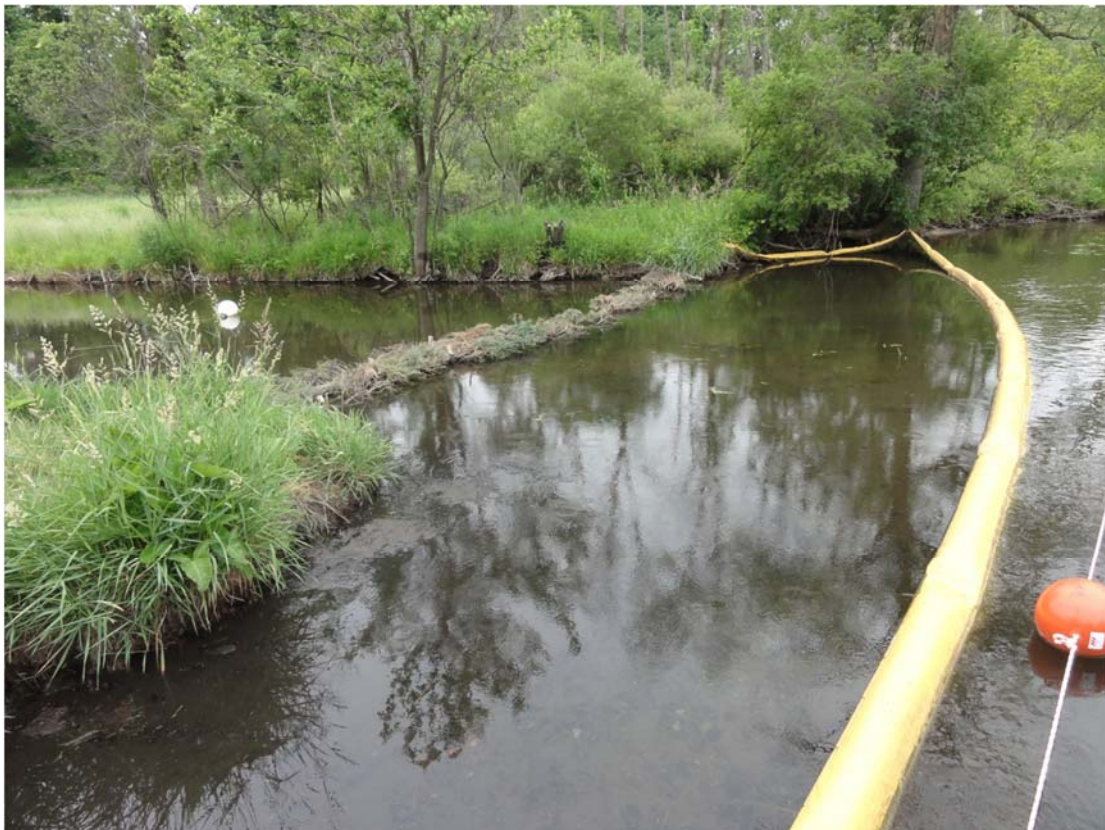
10. MP10.75 sediment control trap, water levels receding.
