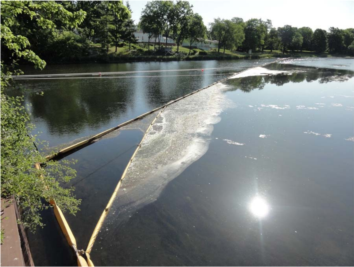
1. Ceresco Dam containment boom.
