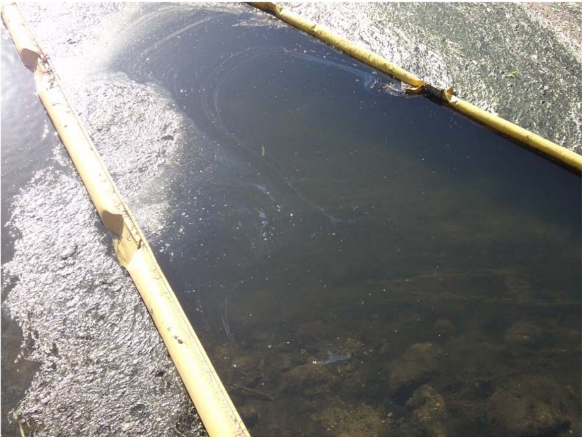
2. Sheen observed between booms at Ceresco Dam.
