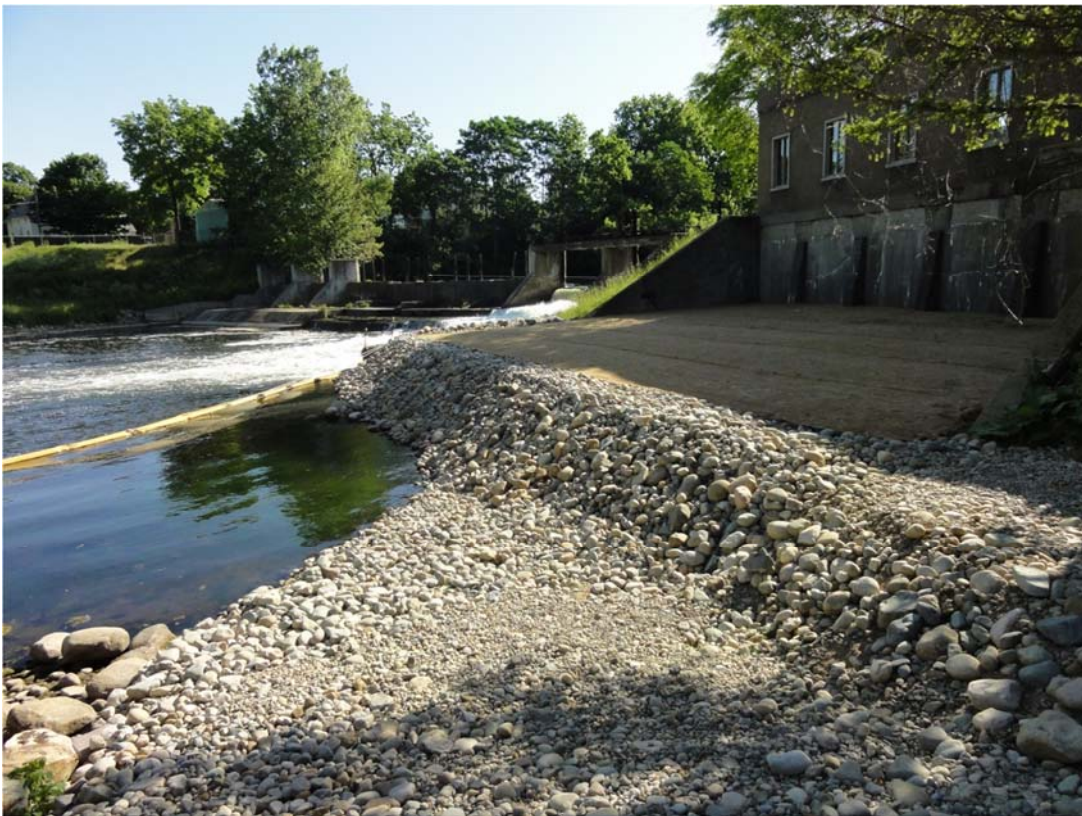
6. Legacy work below Ceresco Dam.
