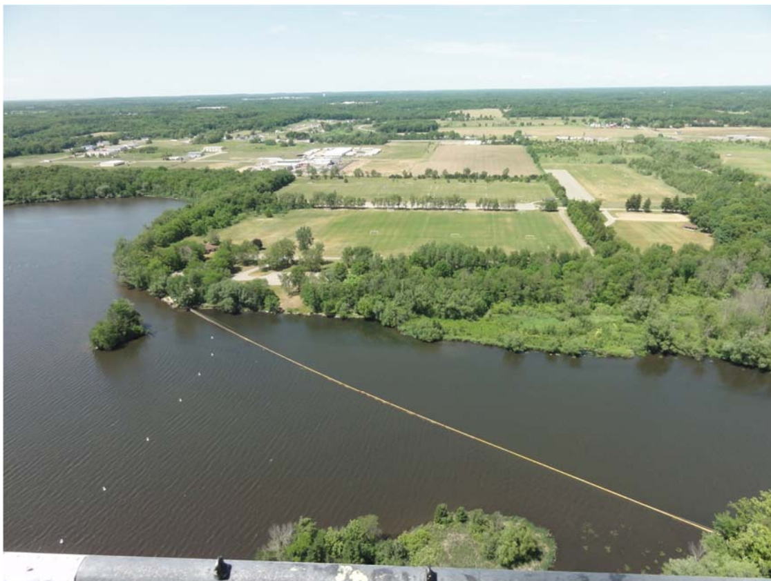
19. Control Point E4 no sheen observed.
