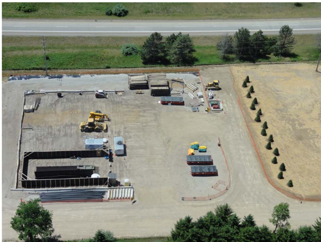
2. Frac-Tank City decon pad and soil cells. Boat observed in decon area.
