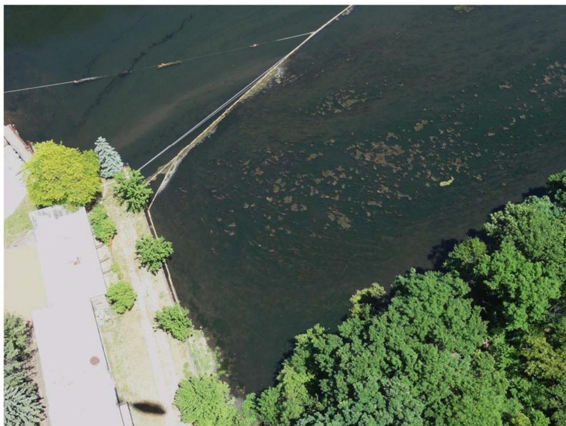
8. Control point above Ceresco Dam, some debris observed within containment.
