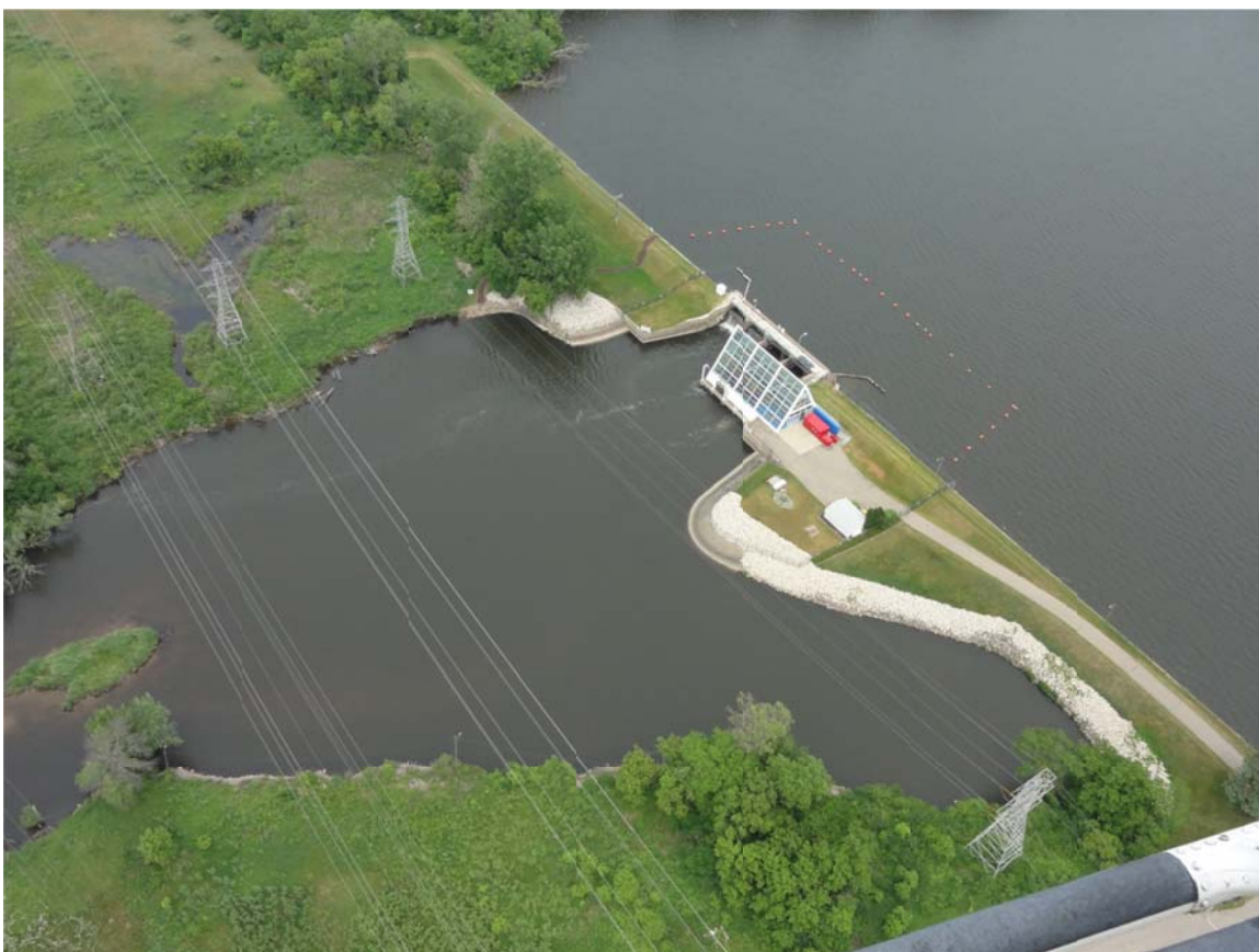
17. Morrow Lake Dam, no sheen or activity observed.
