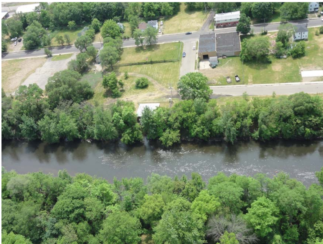
11. Rock Tenn inlet, no activity observed.
