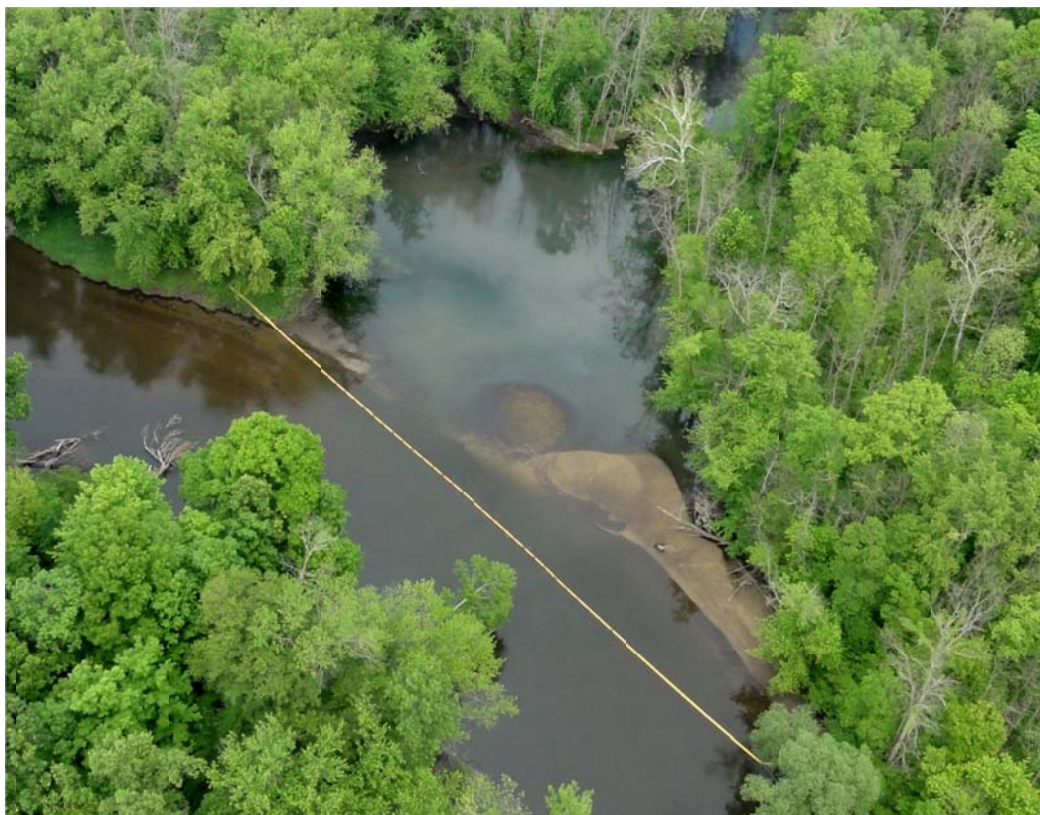
13. MP 30.8 LDB containment. Sheen observed within containment. Operations crew notified to conduct inspection.
