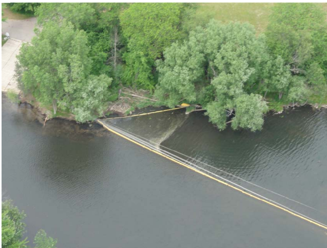
14. E4.0 control point. Debris observed within containment. No sheen observed.
