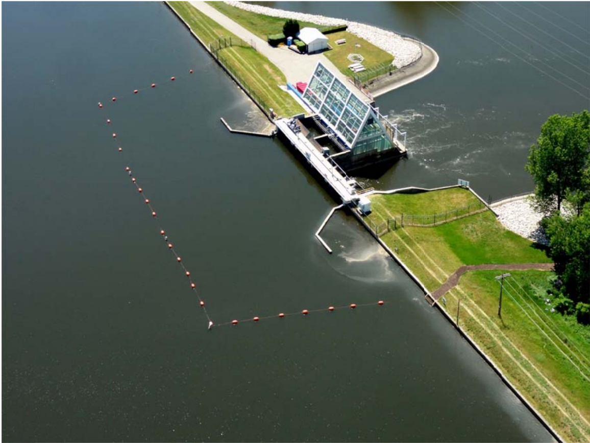
23. Morrow Lake Dam. Sheen observed along shoreline north of spillway. Operations crew notified.
