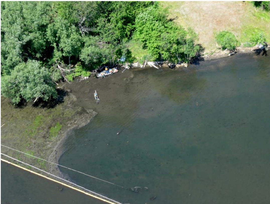
20. Crews removing vegetation and debris from E4.0 control point.
