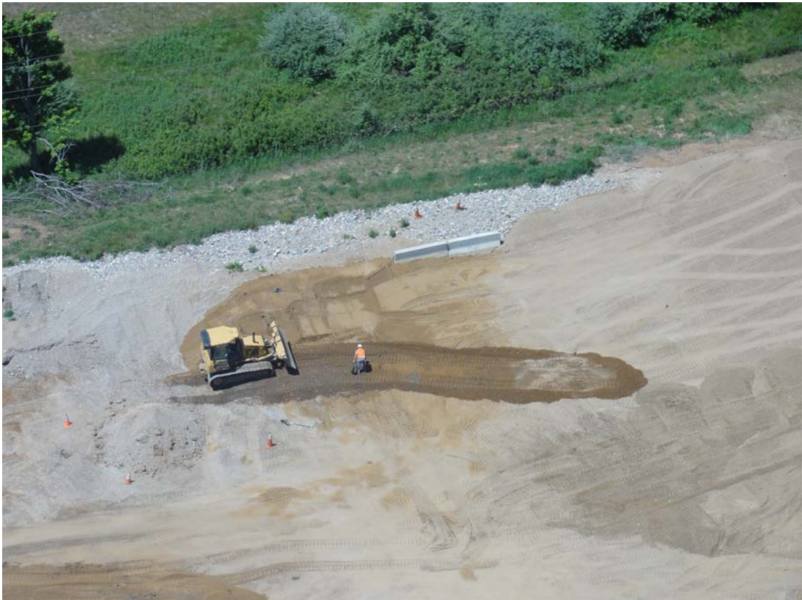
4. Frac-Tank City, footprint reduction continues.
