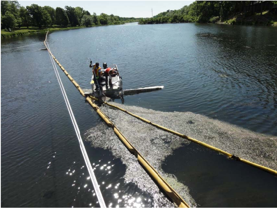
9. Ceresco Dam, crews removing debris from containment above dam.
