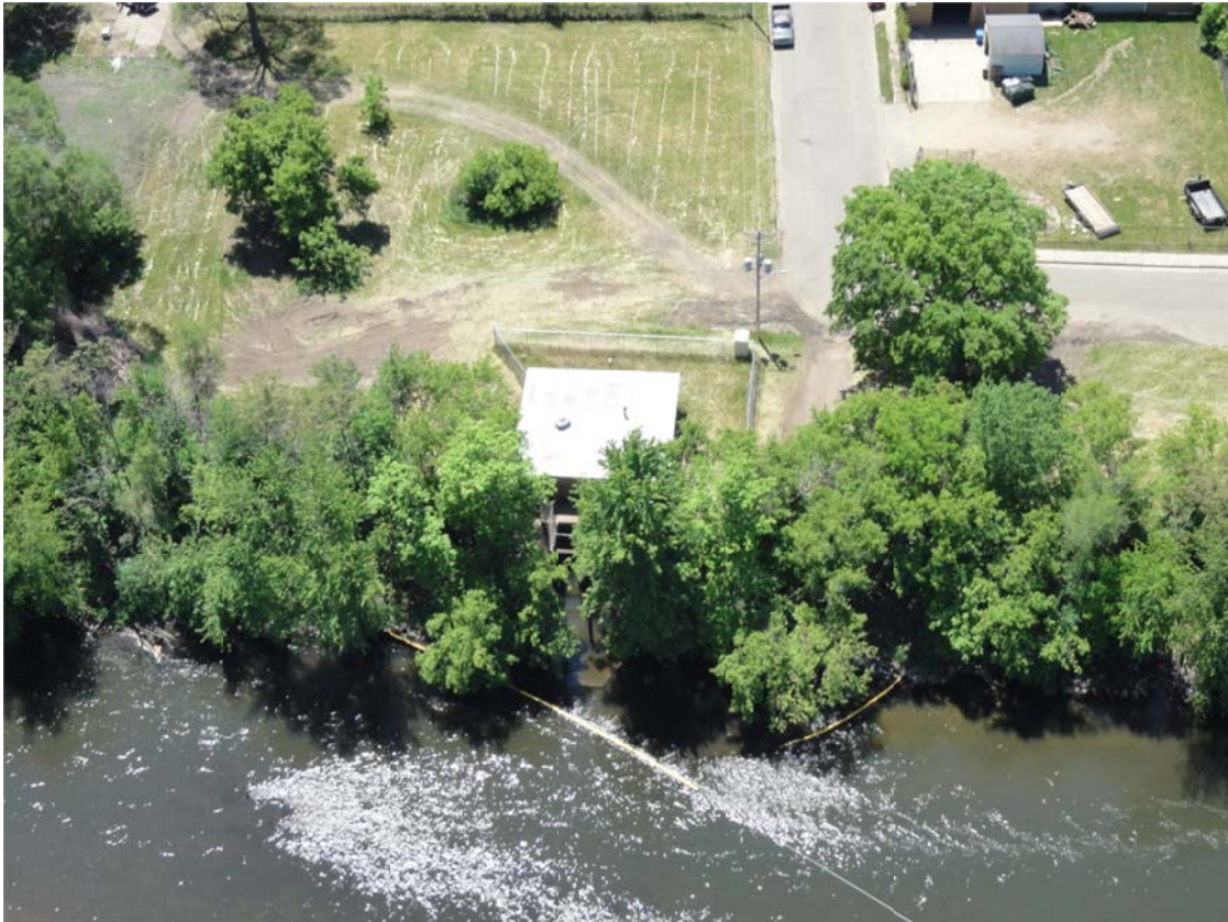
17. Rock Tenn inlet, no activity observed.
