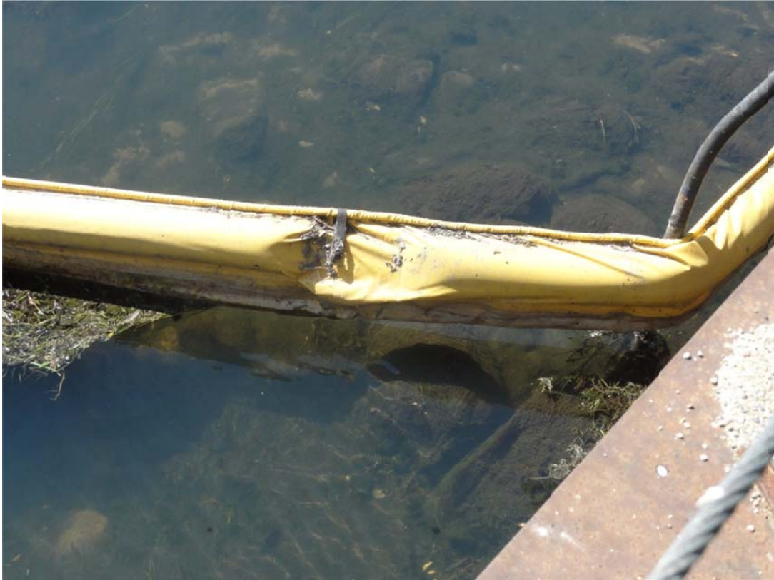
10. Ceresco Dam. Water level has dropped below containment boom, containment crews notified of need to adjust boom height.
