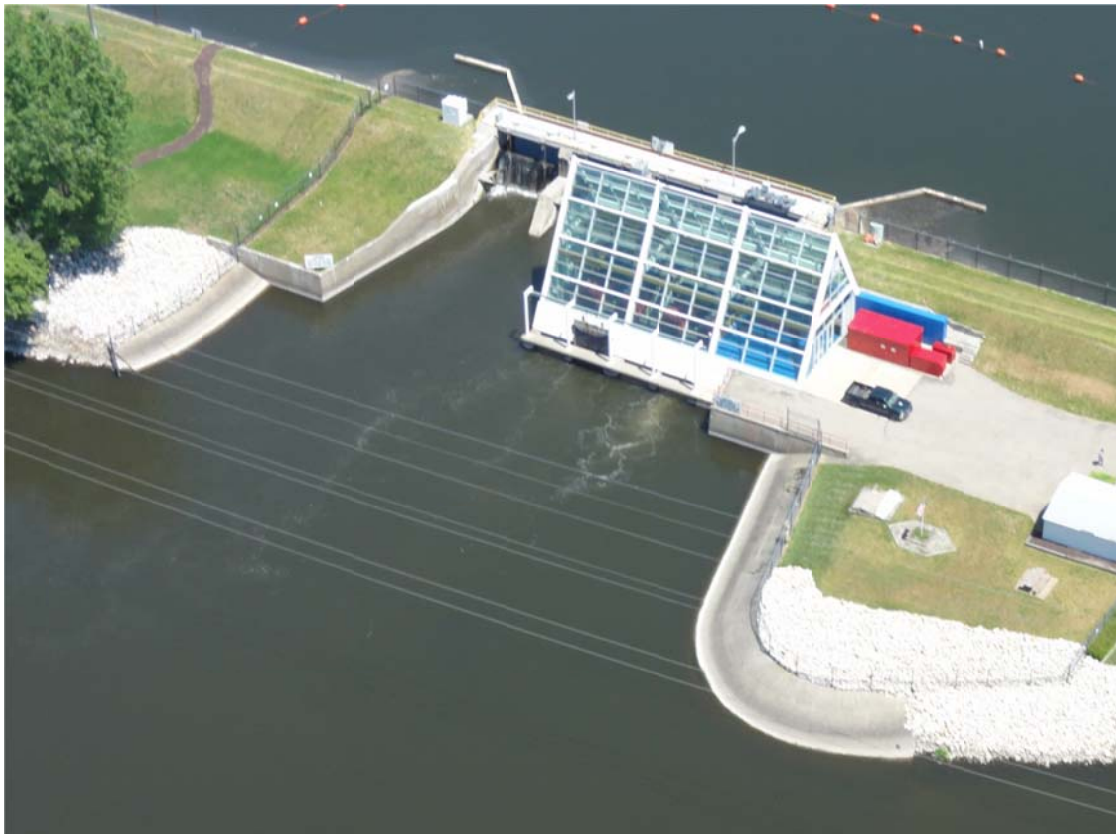
24. Close up of Morrow Dam discharge.
