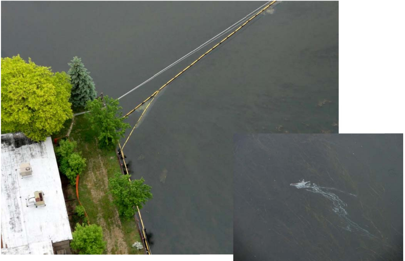
9. Control point above Ceresco Dam, sheen observed within containment.
