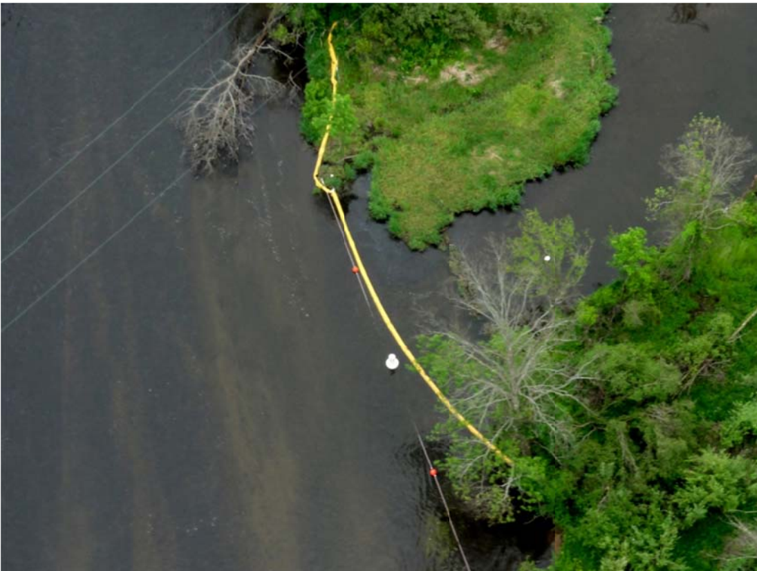
12. MP 10.75 LDB sediment trap, sheen observed within containment.
