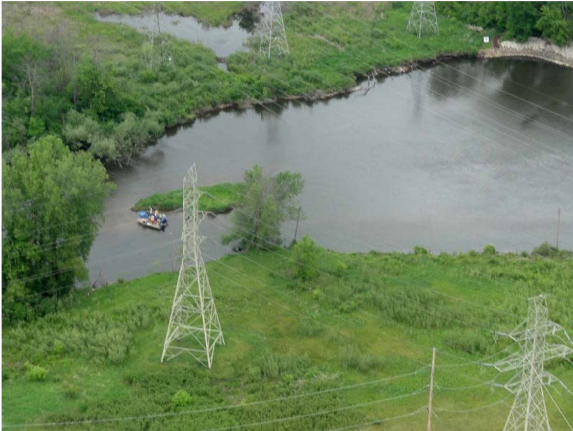
27. Poling crew operating below Morrow Lake Dam.
