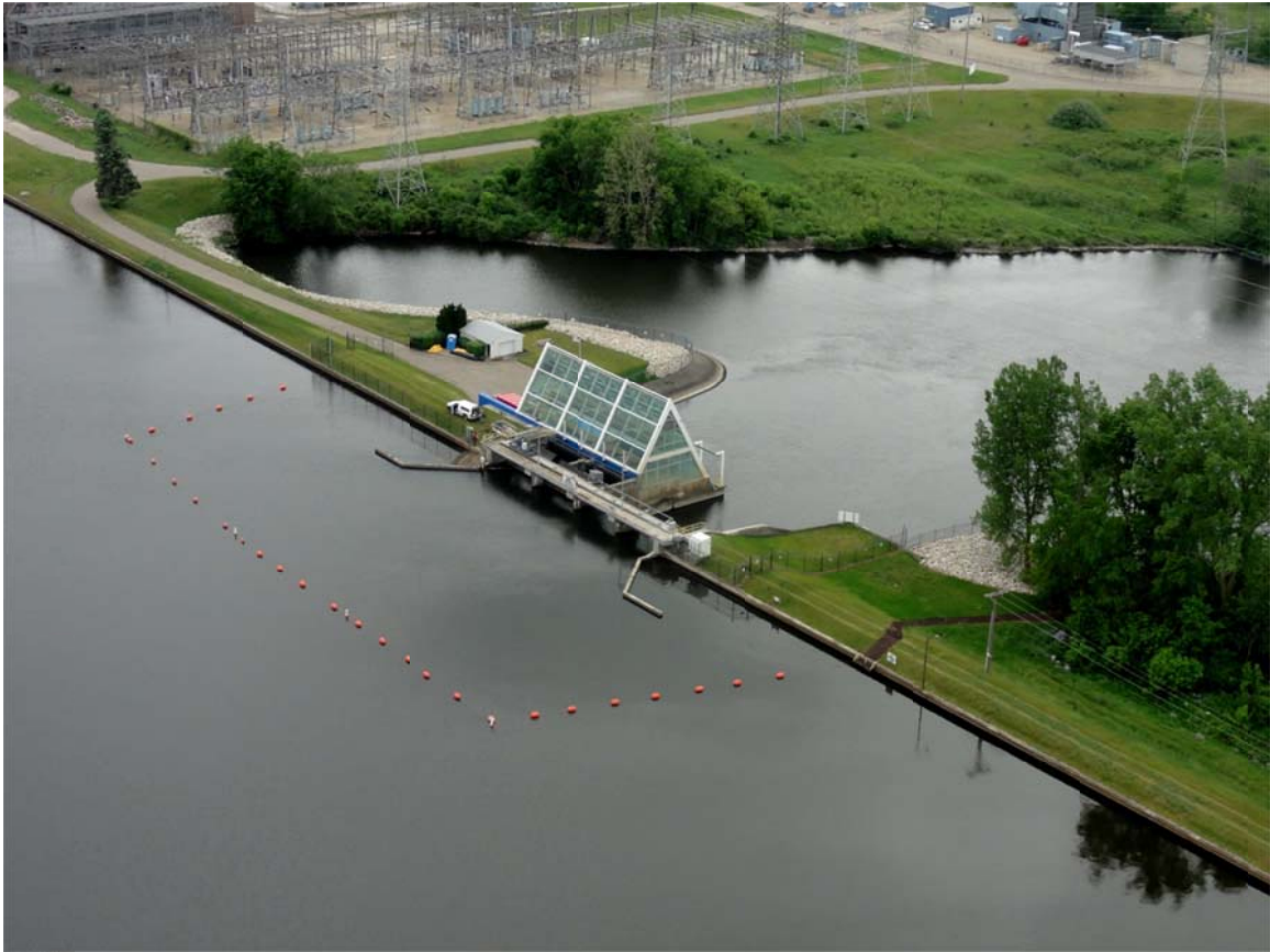
23. Morrow Lake Dam. One poling crew observed upstream from dam.
