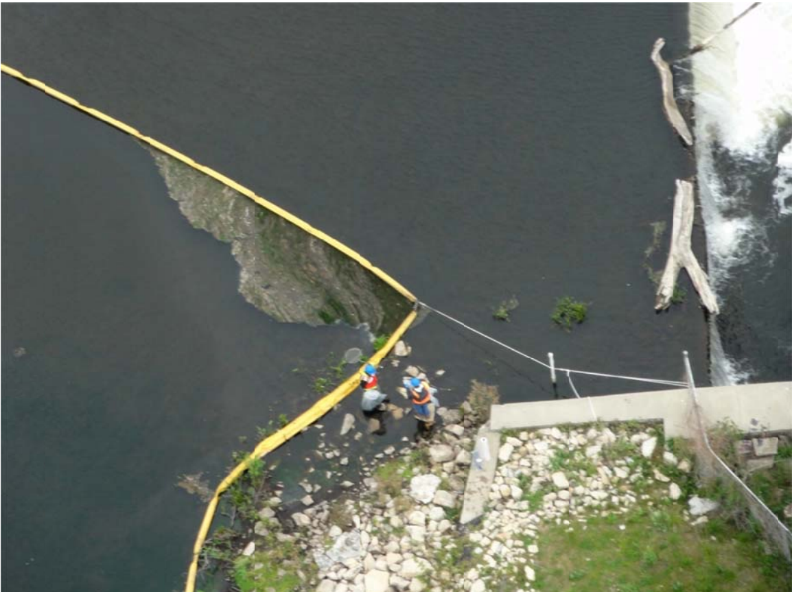
16. Control point at Battle Creek spillway. Crews observed removing debris from boom.
