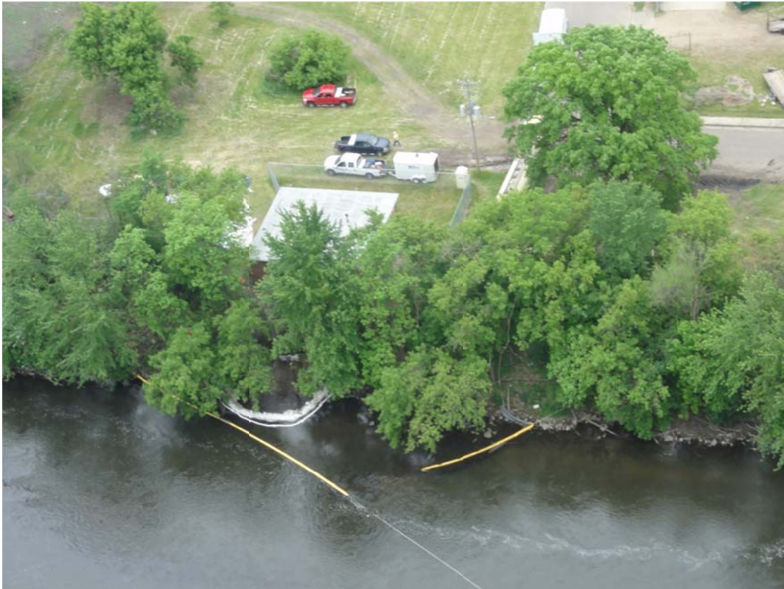
17. Rock Tenn inlet, crews observed cleaning inlet inside containment.
