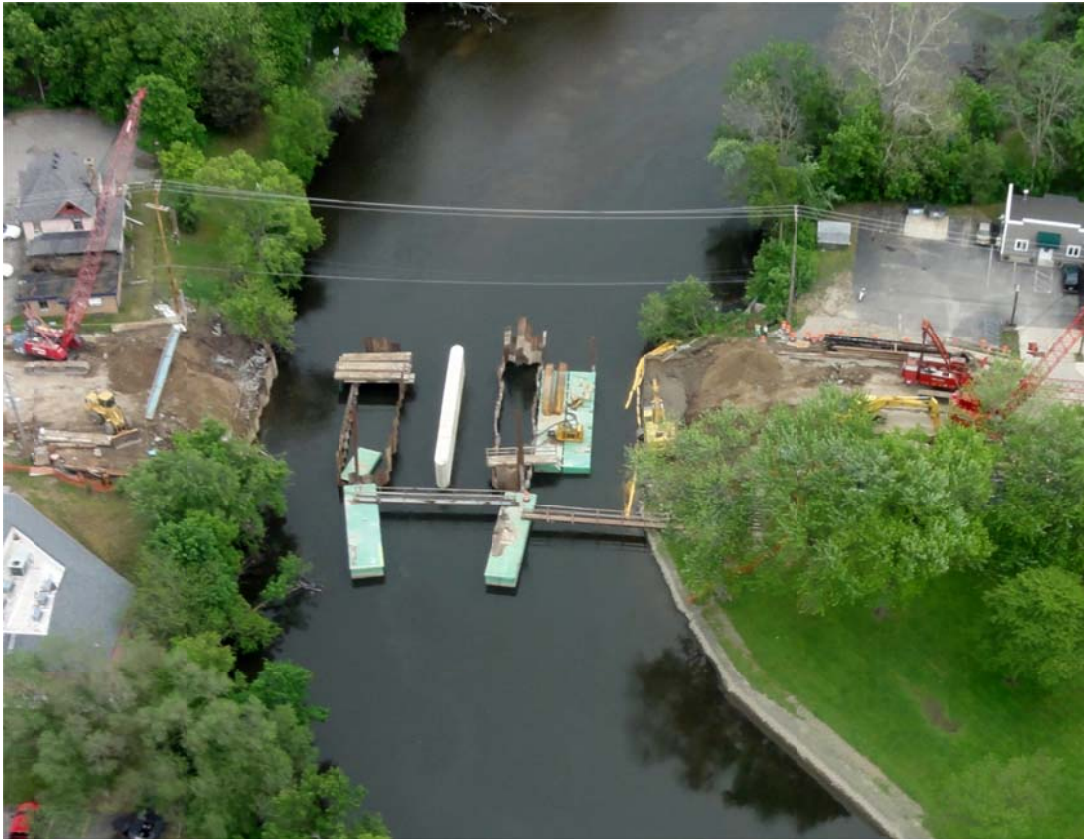
25. Bridge under construction downstream from Morrow Lake Dam.
