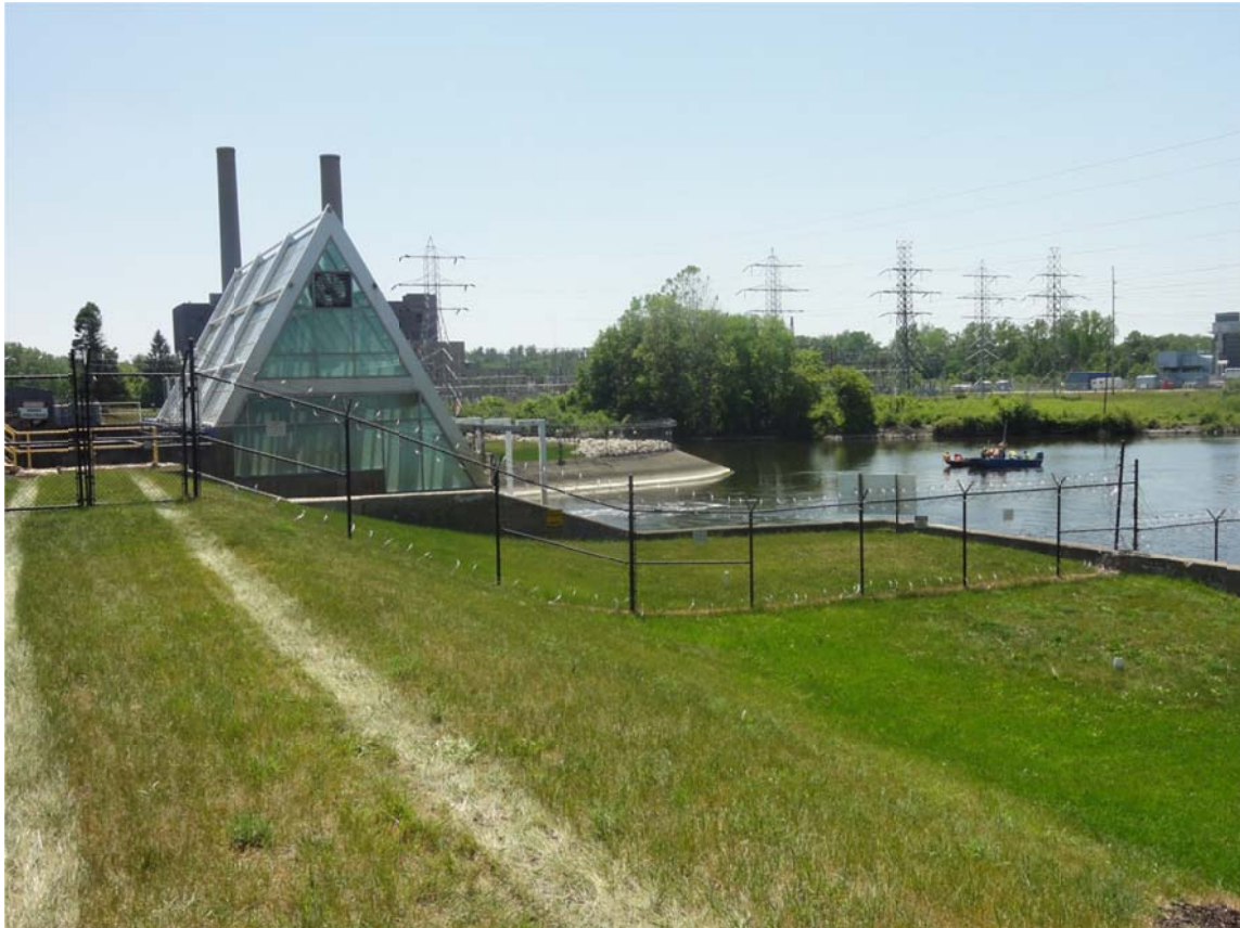
23. Poling crew observed downstream of Morrow Lake Dam.
