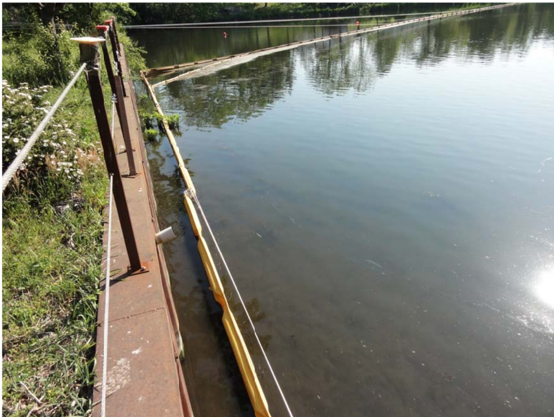
2. Sheen observed above Ceresco Dam within containment.
