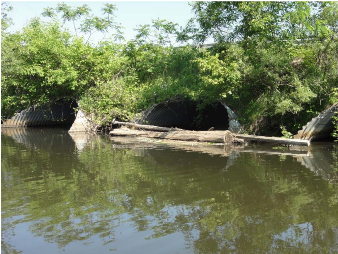
16. Culverts at MP 15.75, north end of Mill Ponds, no sheen observed.
