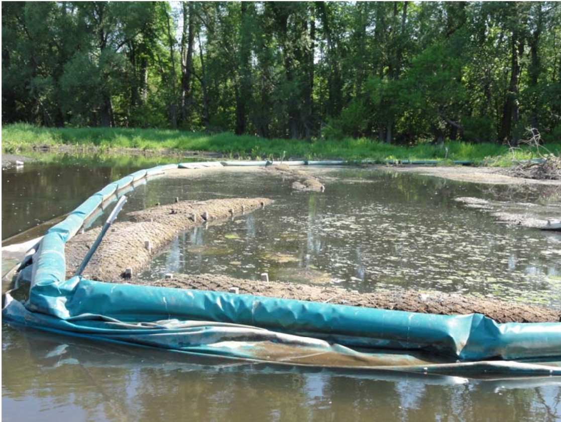
15. MP 14.98 Island. Containment boom remains in place around island.
