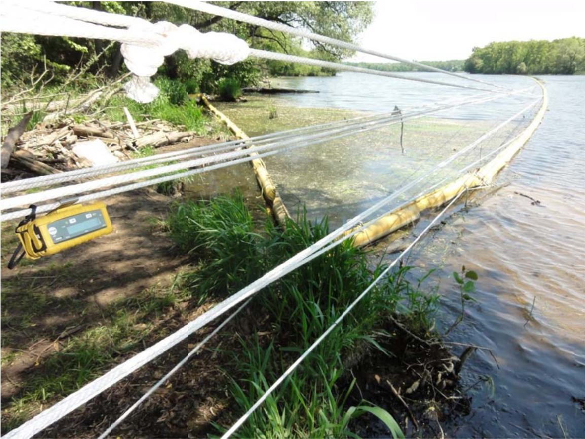
17. Control Point E4, crews observed removing debris within containment.
