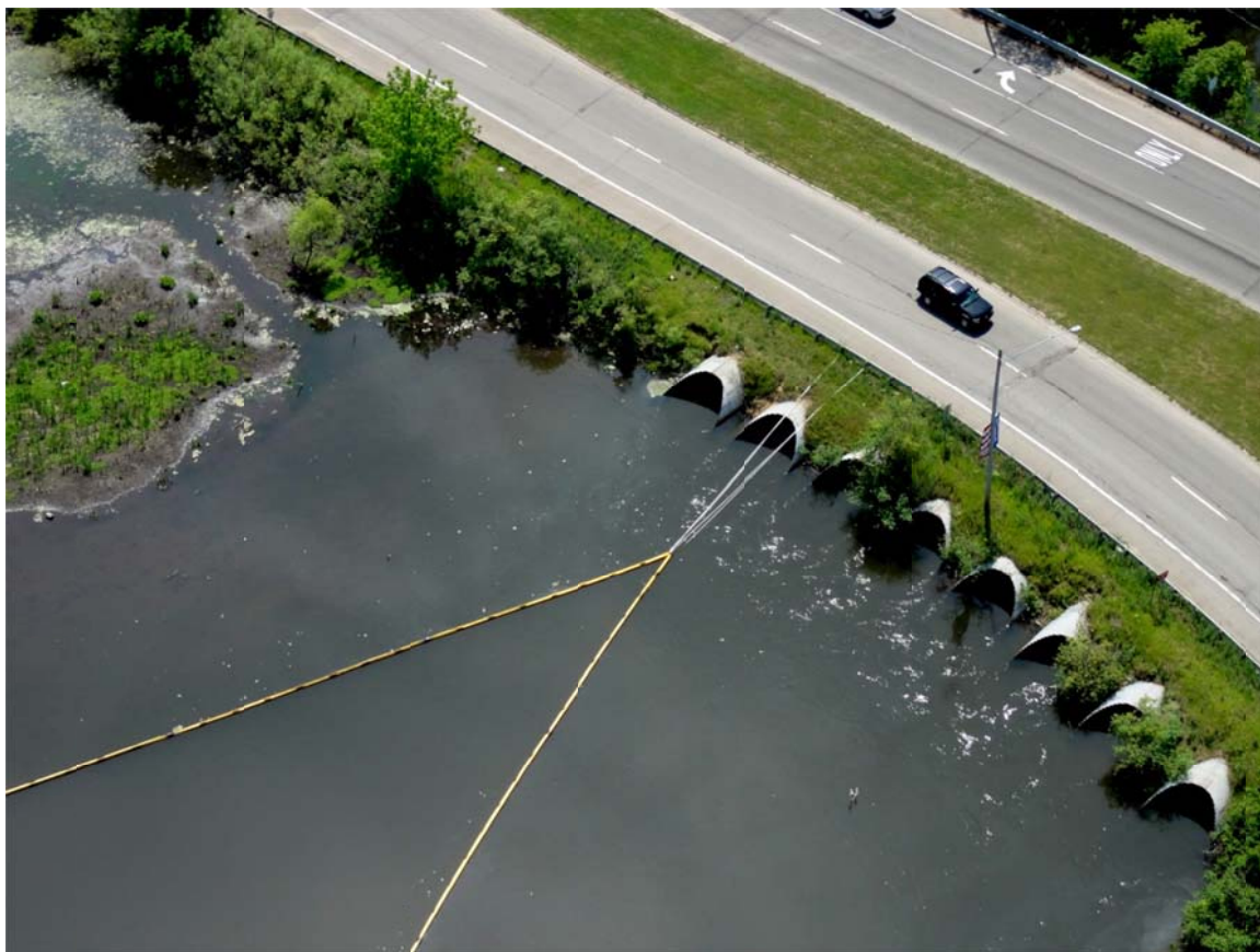
13. Control point at Battle Creek spillway. Sheen observed at culverts.
