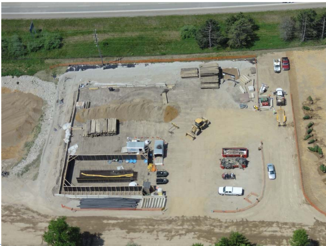
2. Frac-Tank City decon pad and soil cells. Boom observed in decon area.
