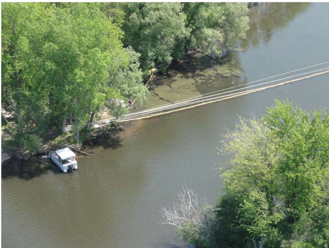
19. Crews removing debris from Control Point E4.
