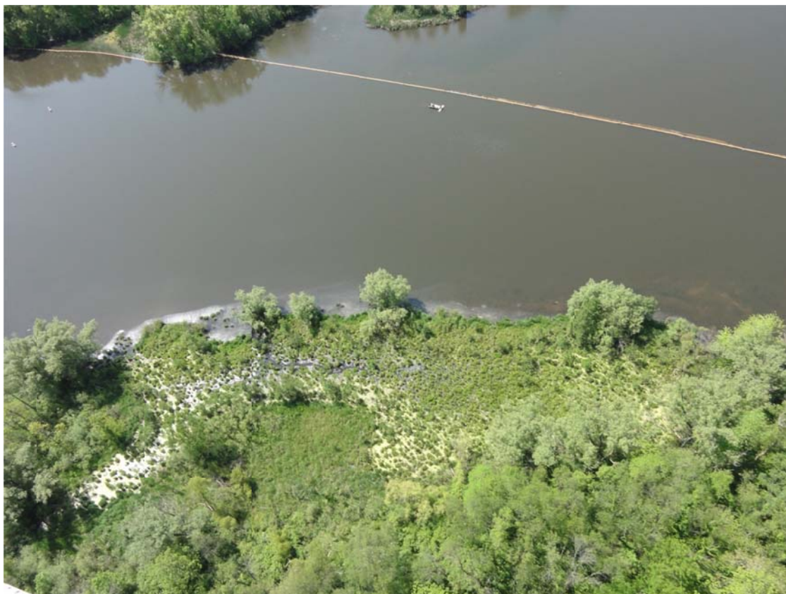
18. Control Point E4, sheen observed along northern shore.
