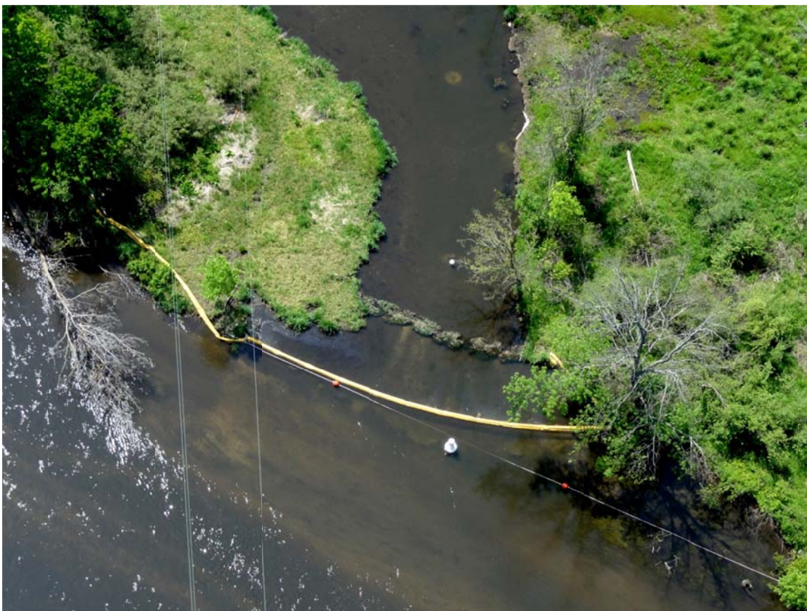
11. MP 10.75 LDB sediment trap, sheen observed within containment.
