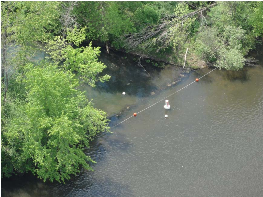
30. MP19.25 sediment control structure #2.
