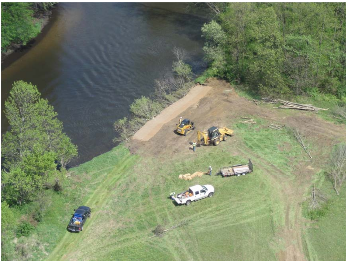
34. MP23.4 shoreline restoration work.
