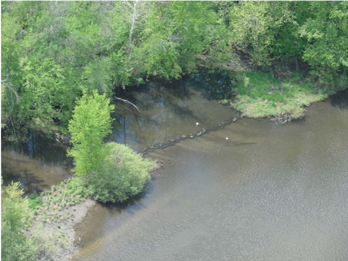
29. MP19.25 sediment control structure #1.
