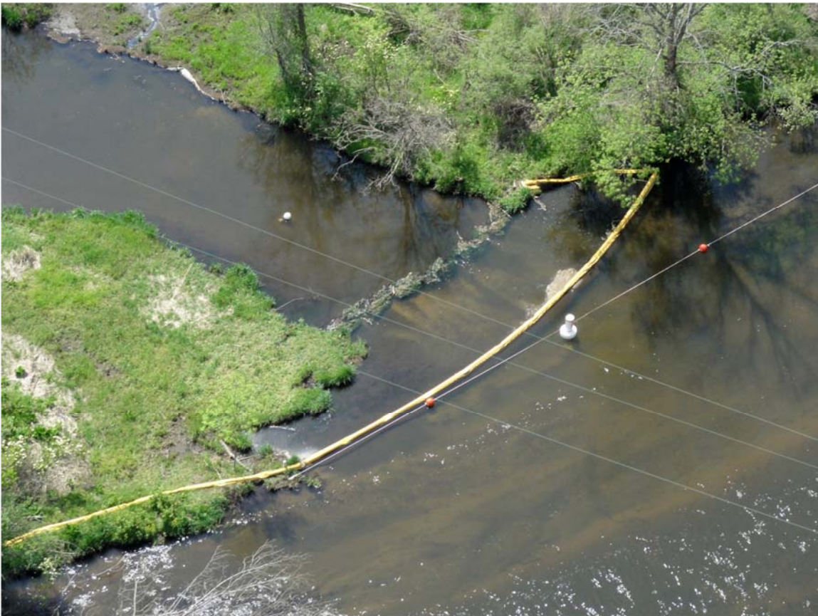
20. MP10.75 sediment trap location.
