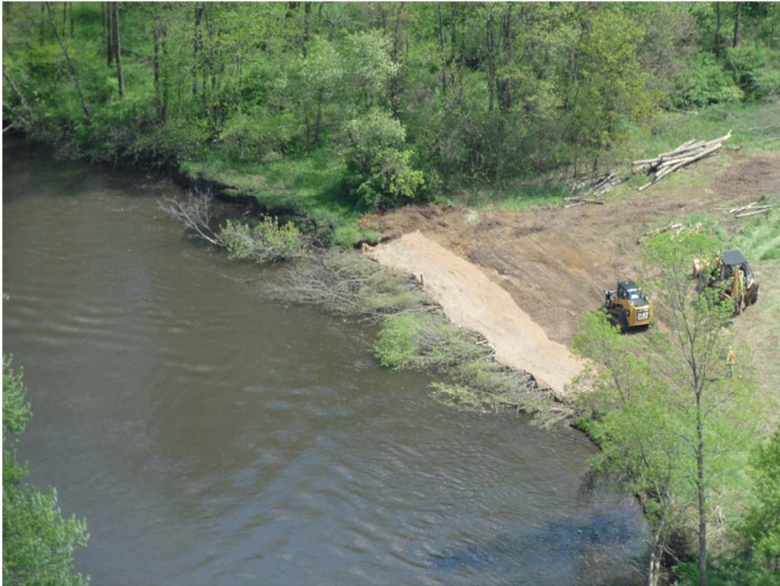
33. MP23.4 shoreline restoration work.
