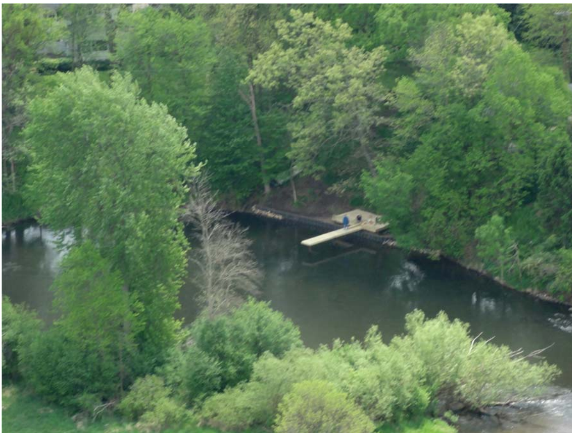
9. MP2.75 LDB new dock installed extending into the river.
