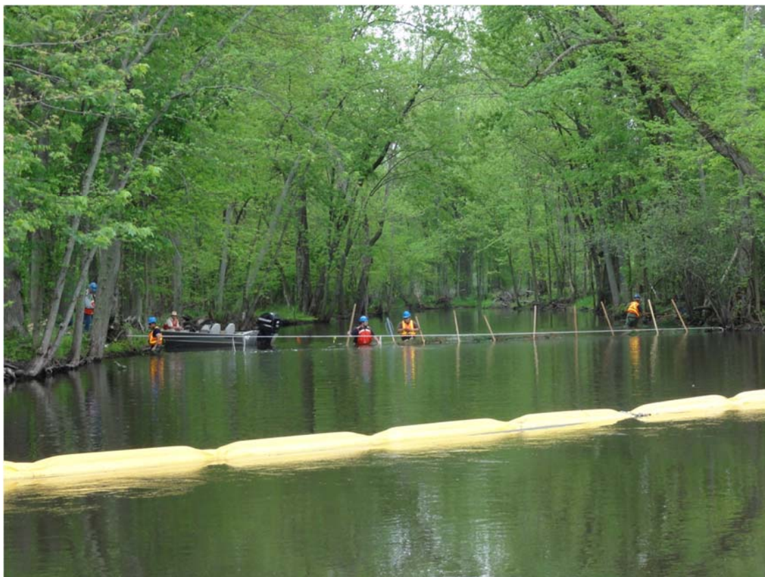
40. MP36.10 sediment trap installation.
