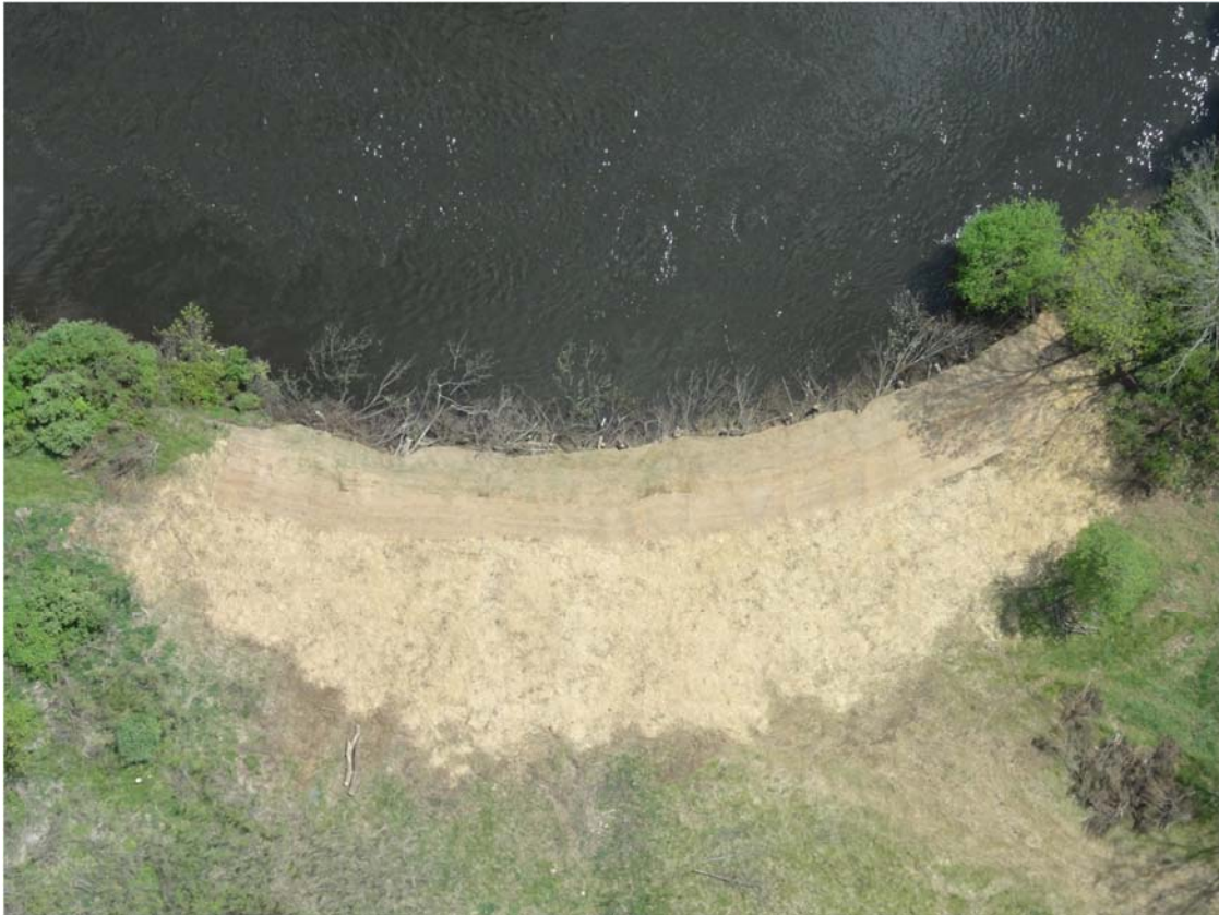
35. MP24.0 shoreline restoration work.
