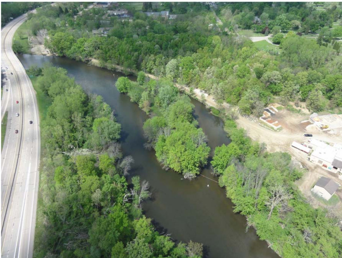
22. MP14.75 sediment trap location.
