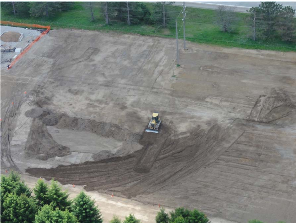
6. Frac-Tank City footprint reduction work continued.
