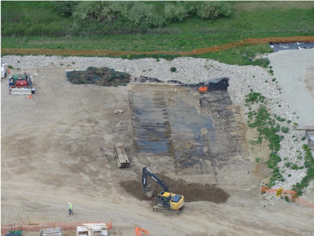
5. Frac-Tank City footprint reduction work continued.
