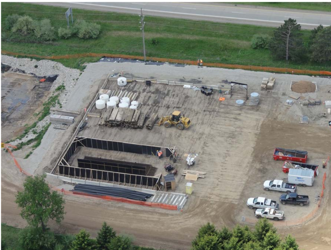
3. Frac-Tank City construction of the new decon pad.
