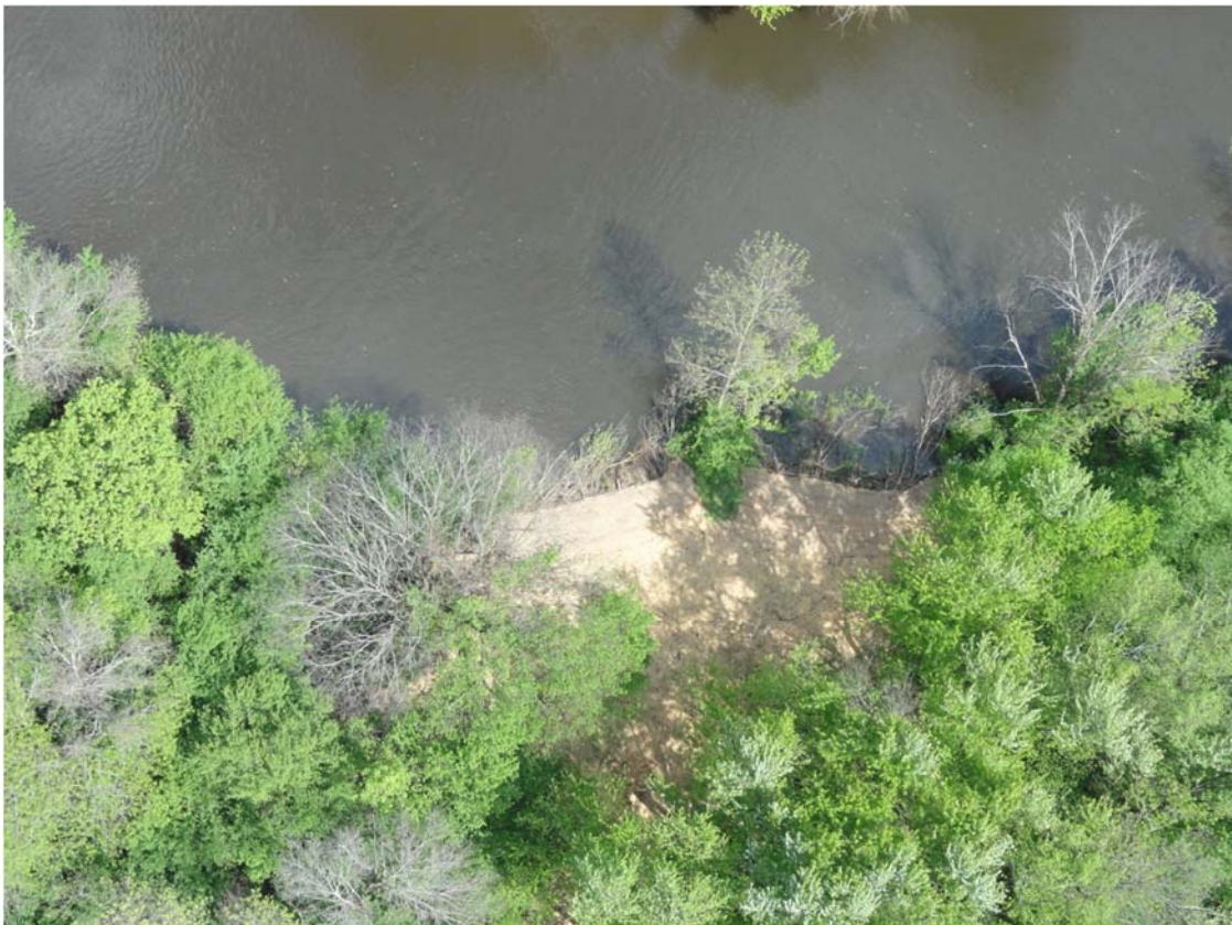
36. MP24.0 shoreline restoration work.
