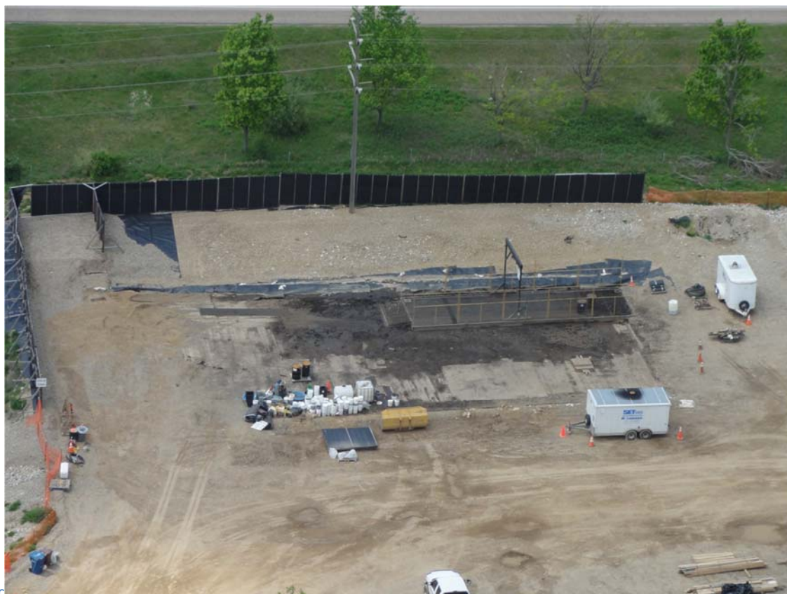
4. Frac-Tank City footprint reduction work continued.
