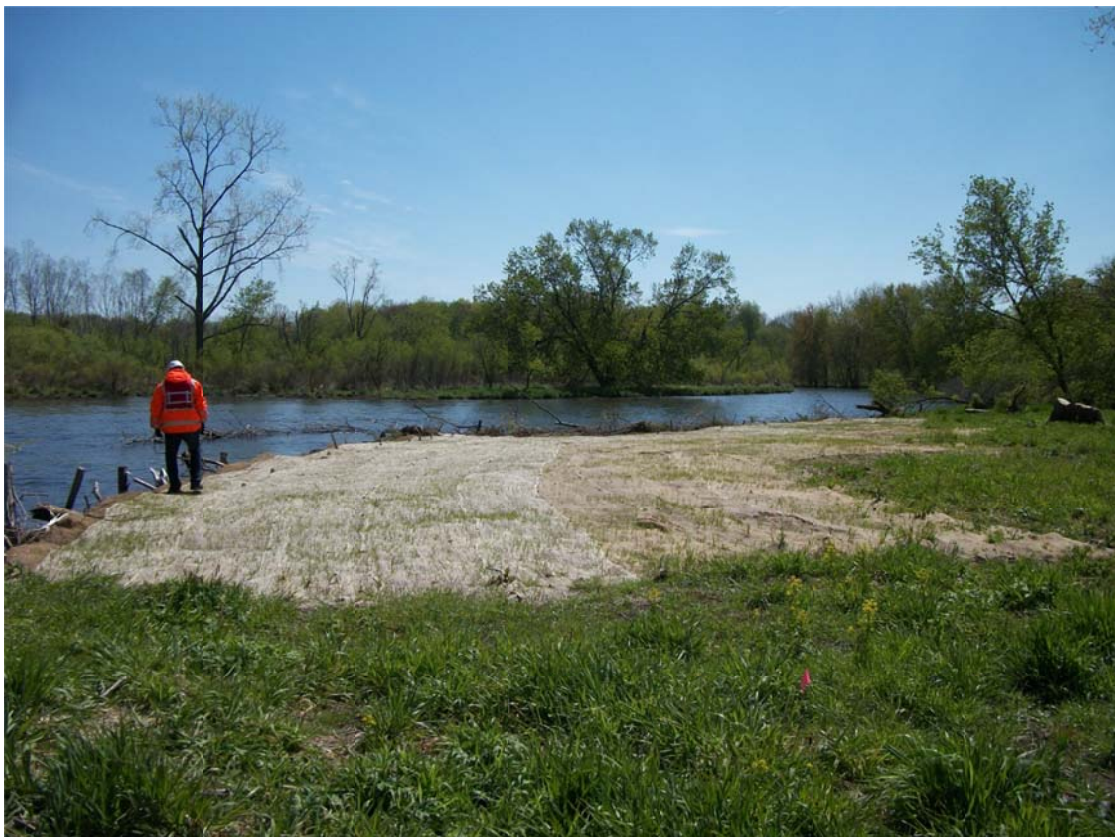
14. Operations personnel inspecting former excavation location at OB 13.40 RDB.
