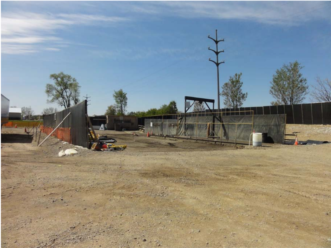
5. Southern decon pad at Frac Tank City. Boom and materials staged in pad.
