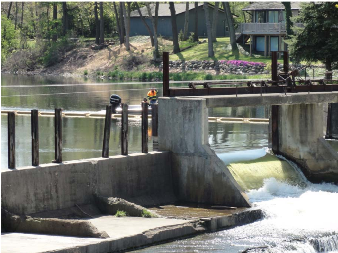
6. Crews conducting boom inspection and maintenance above Ceresco Dam.
