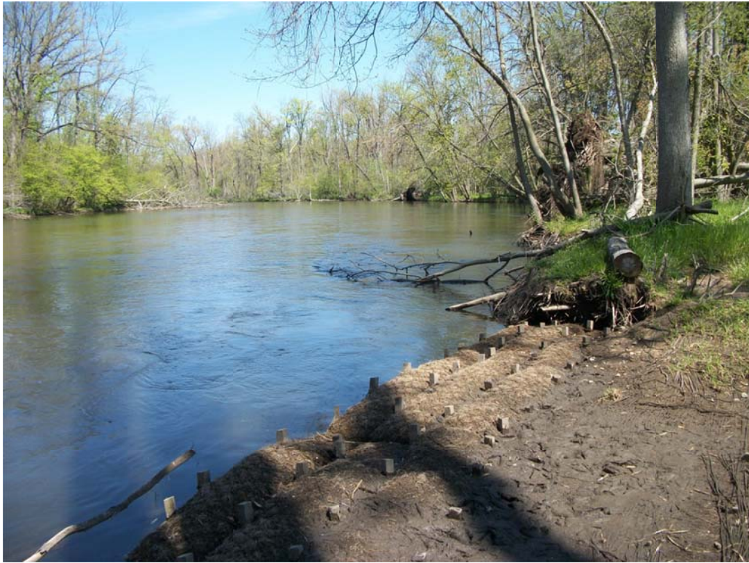
13. Restoration at former excavation area at MP 11.25 R2. Operations personnel inspected this location today.
