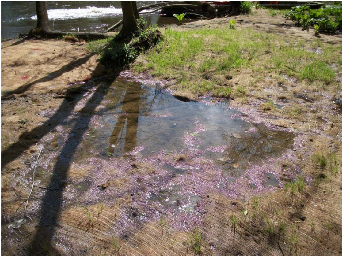
9. Former excavation site at MP 9.10. Area inspected by Operations today.
