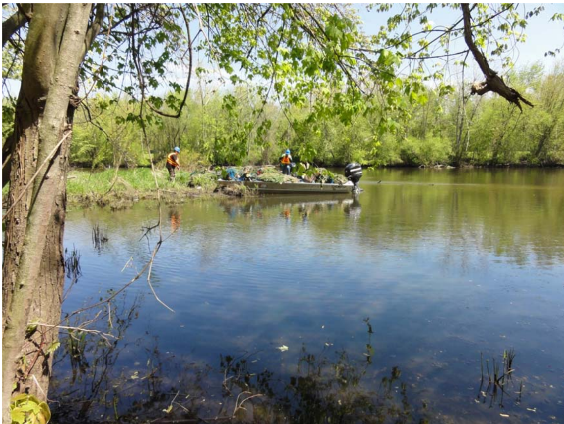
16. Crews off-loading materials for sediment trap installation at MP 19.25 LDB.
