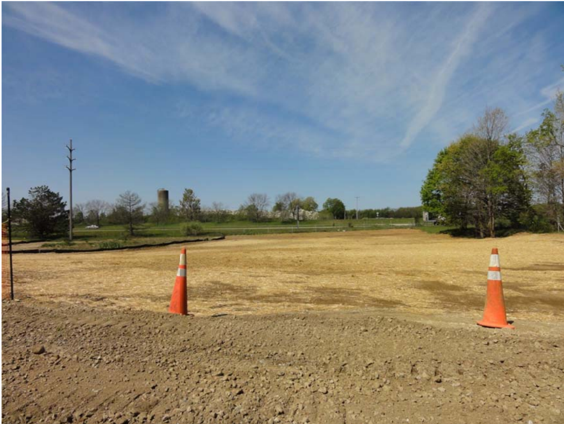
3. Crews continue footprint reduction at Frac Tank City.
