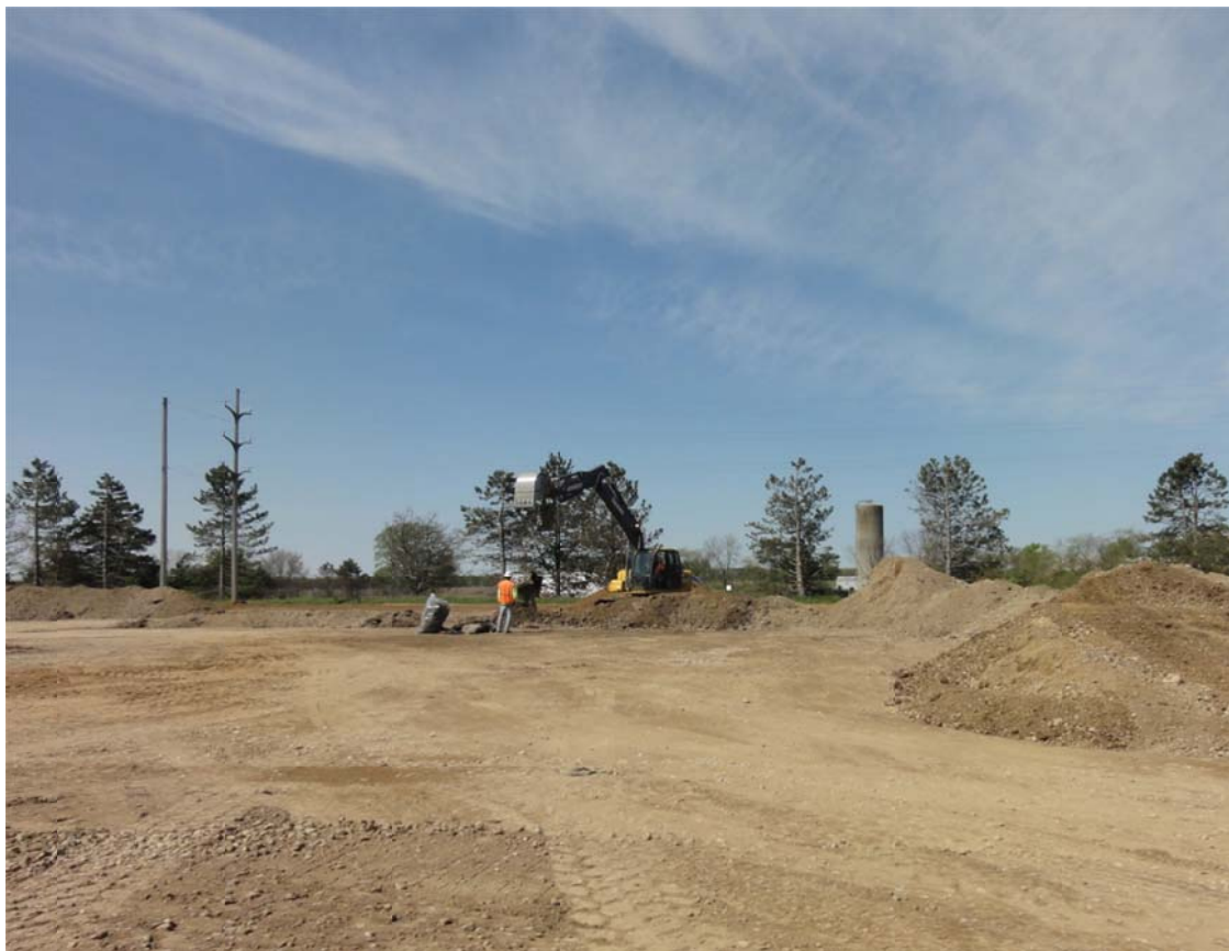
4. Gravel removal in northern end of Frac Tank City.
