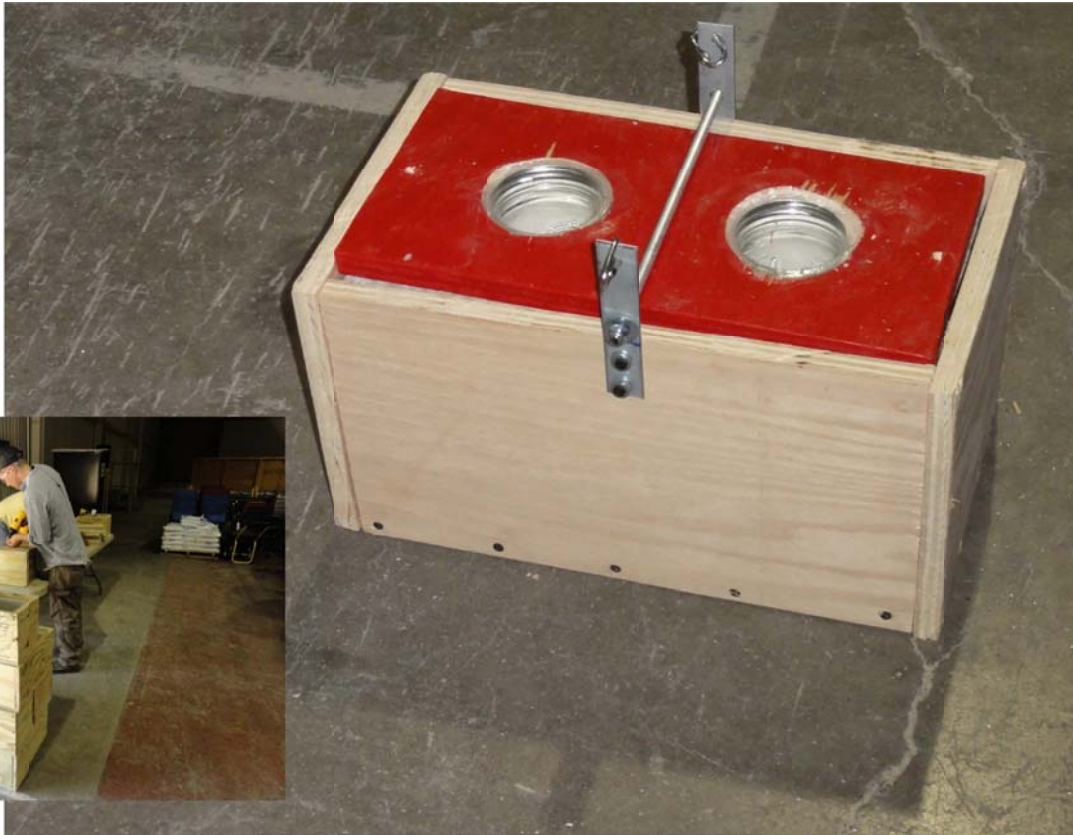
1. Crews building sediment collection devices for installation with sediment traps.
