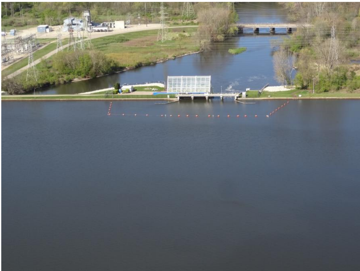
28. Morrow Lake Dam buoys reinstalled.
