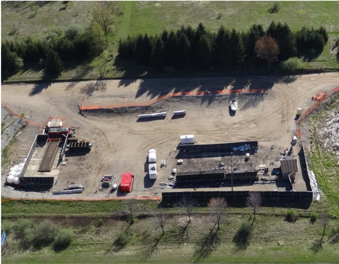
3. Frac-City decontamination pads.
