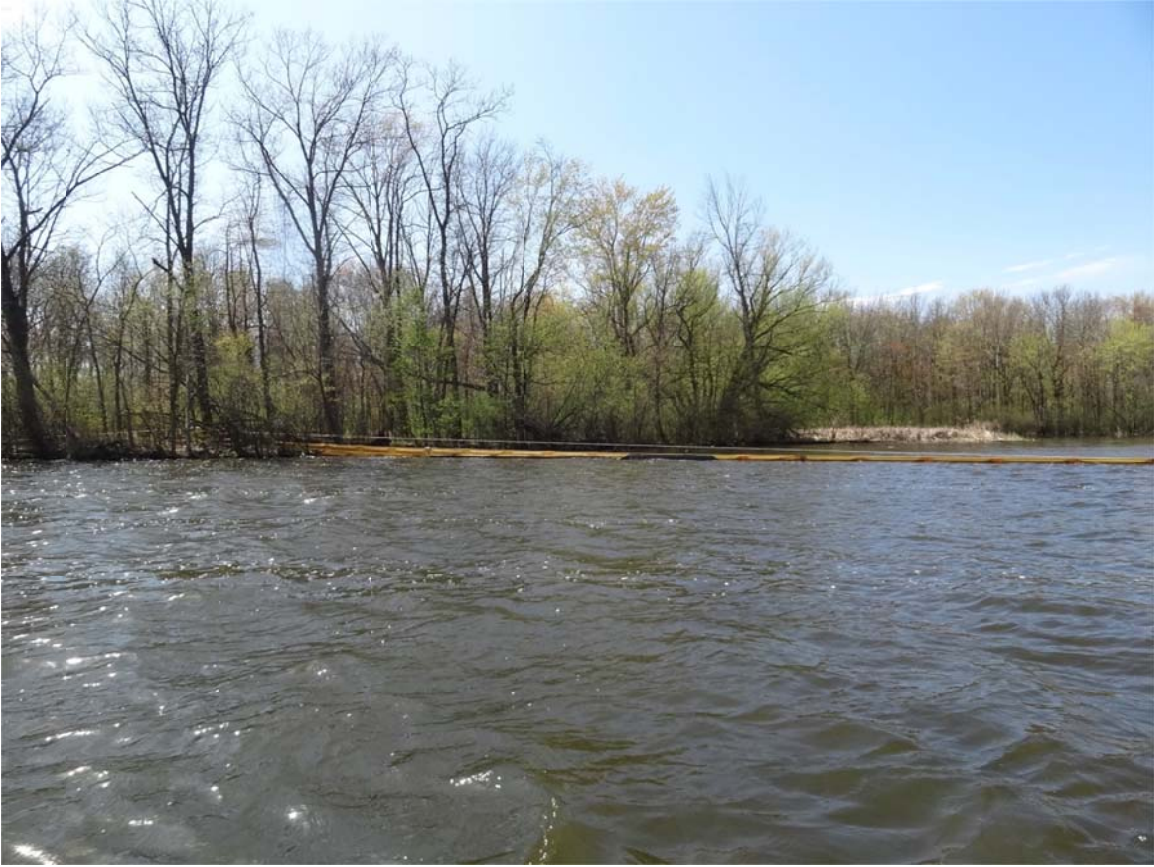
11. E4 Containment boom in place.
