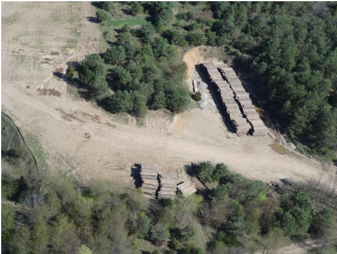
5. Timber mat staged off Talmadge Creek near MP1.5.
