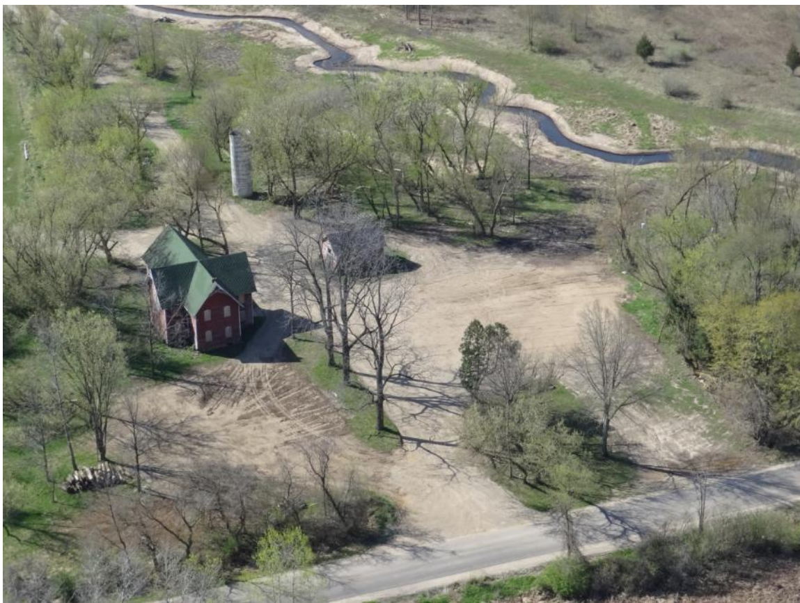
1. Demobilization of the staging area at the farmhouse on Division Drive appears complete.
