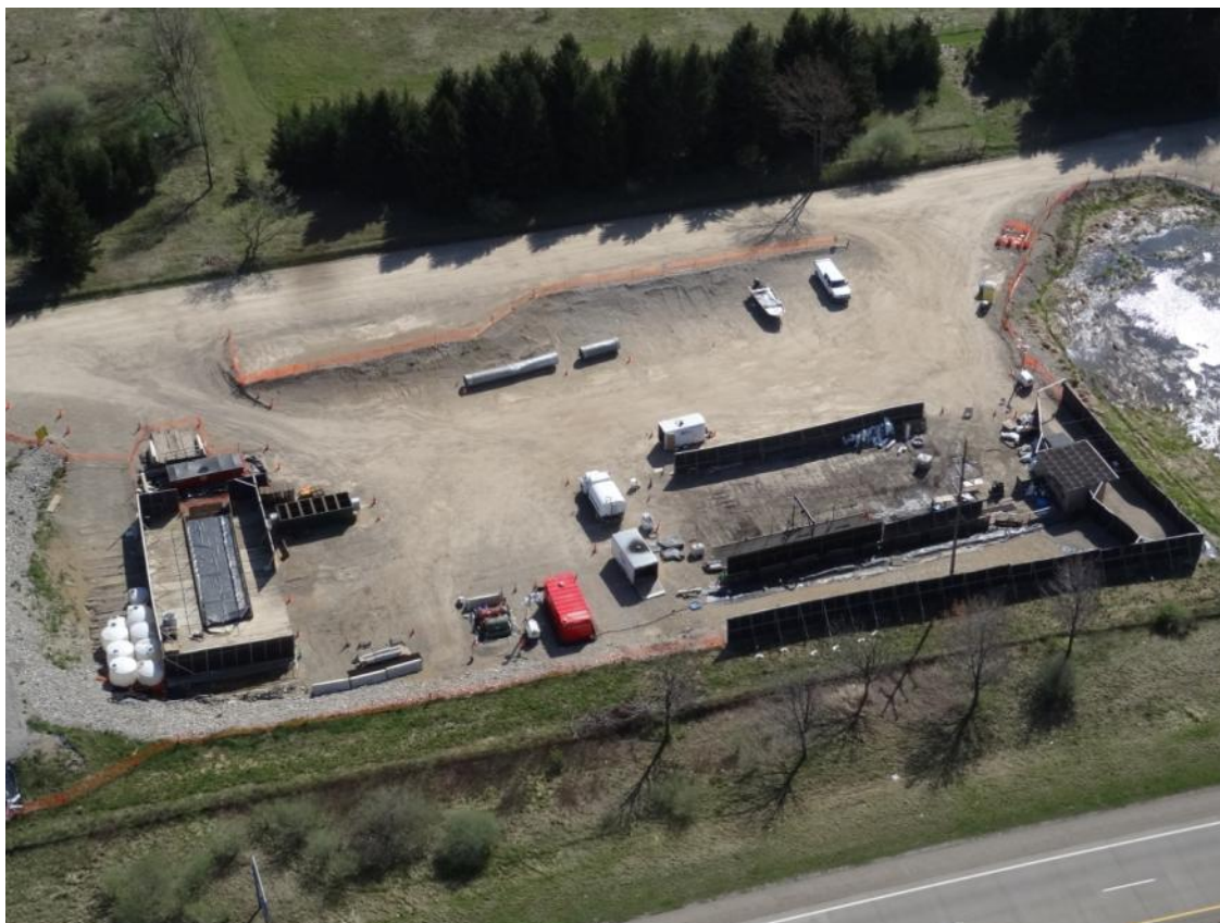
3. Frac-City no decontamination activities observed.
