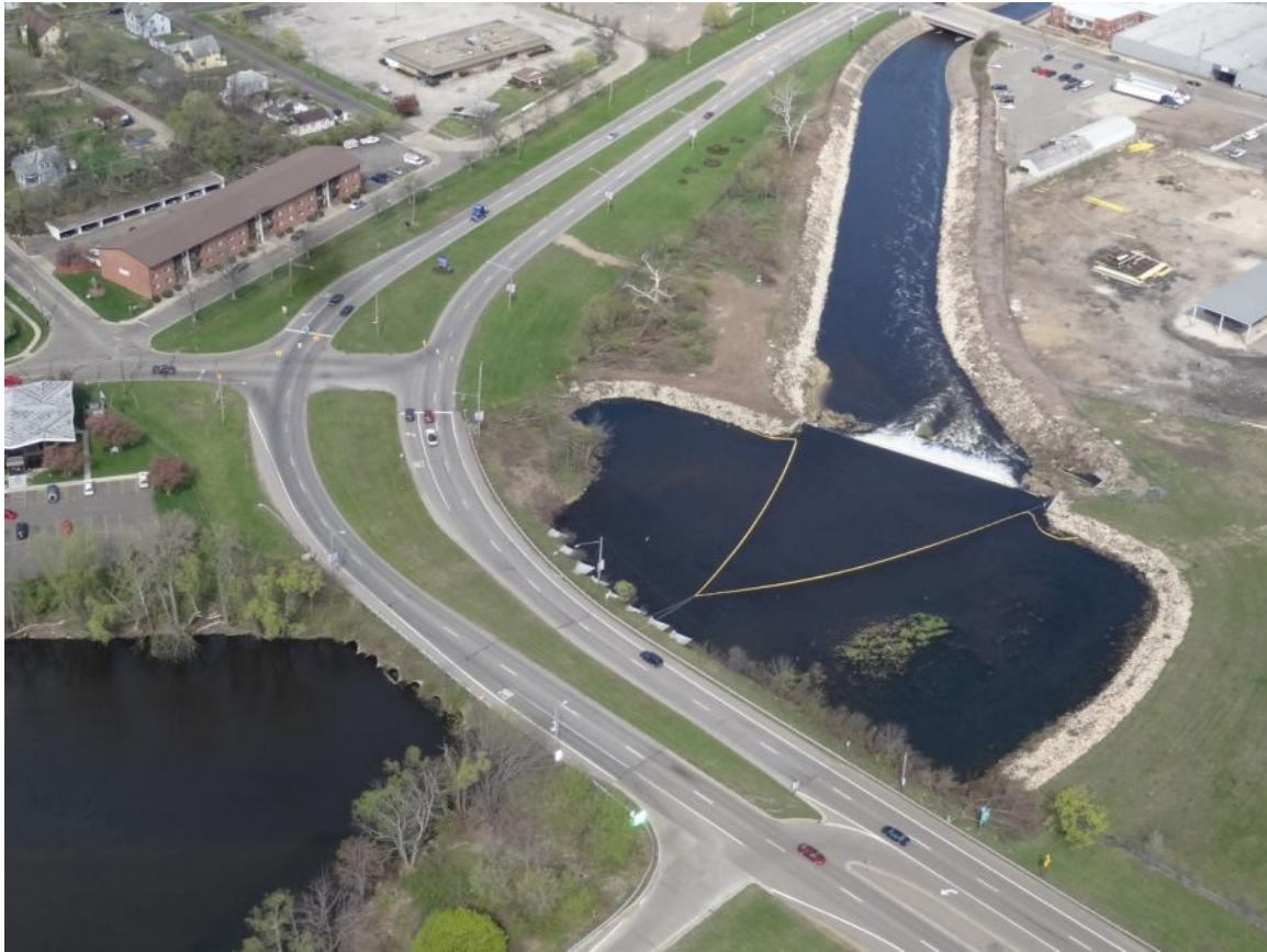
15. MP15.75 boom installed at the Battle Creek Spillway.
