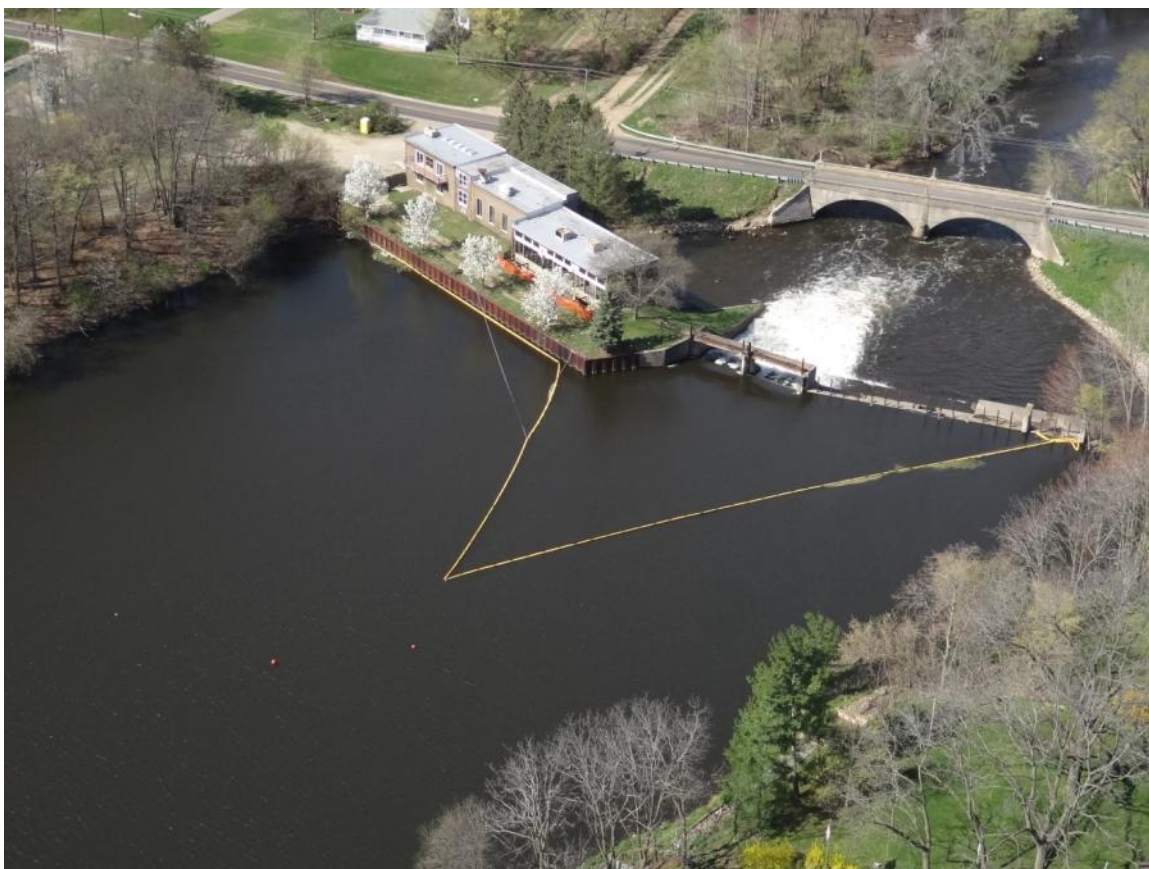
10. Ceresco Dam observed newly installed boom.
