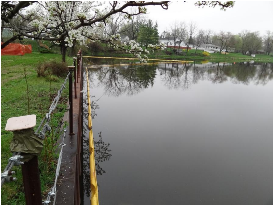
12. Ceresco Dam boom.
