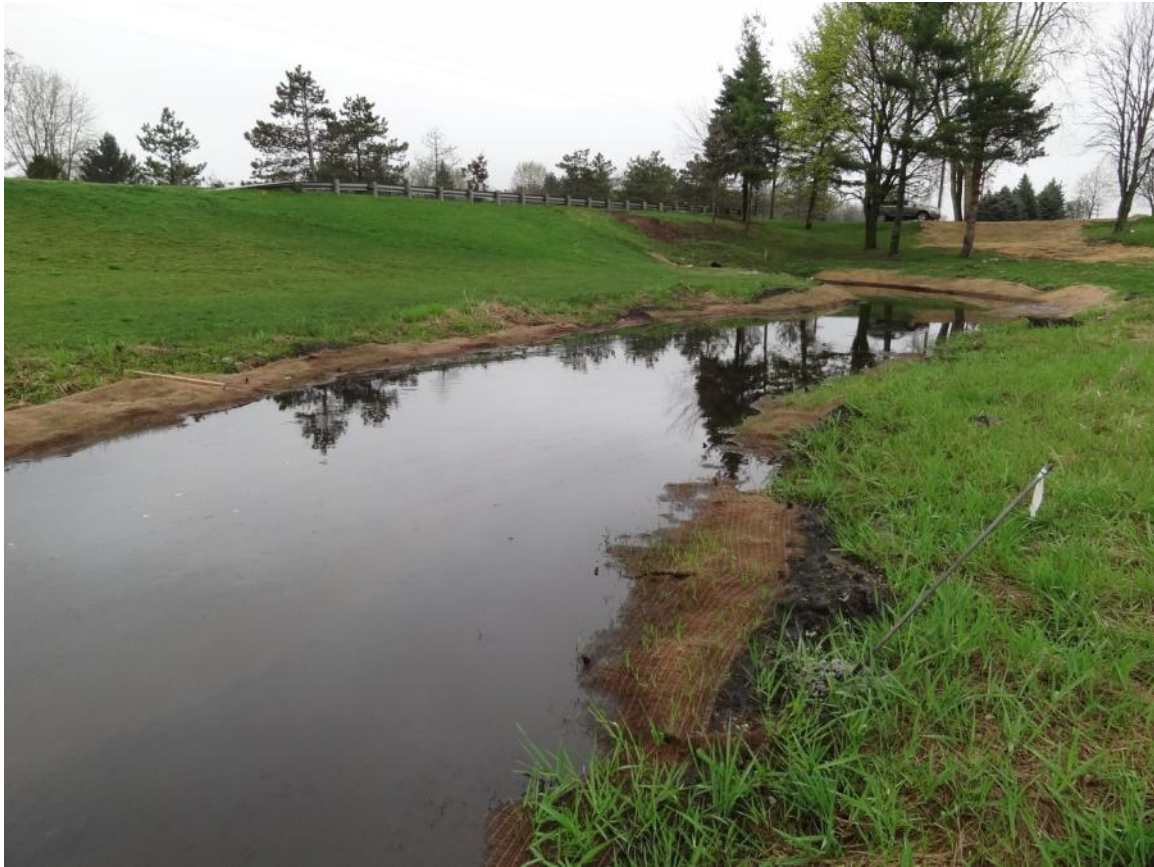
27. Talmadge Creek east of 16 Mile Rd, no turbidity or sheen observed.
