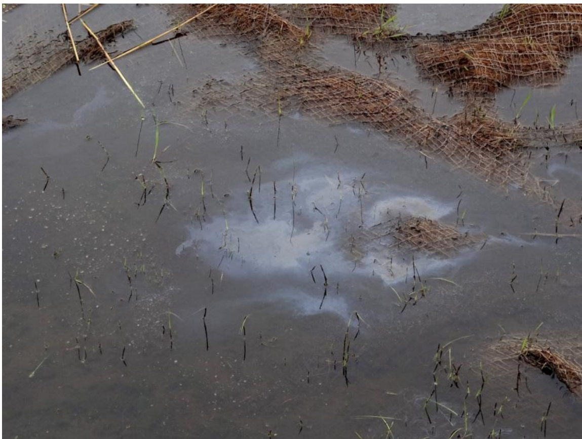
29. Talmadge Creek MP1.0 RDB overbank sheen observed.
