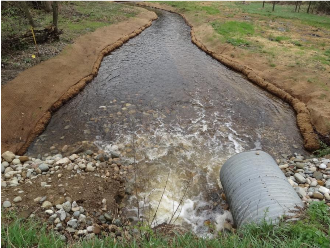
25. Talmadge Creek west of 15 ½ Mile Rd no turbidity or sheen observed.
