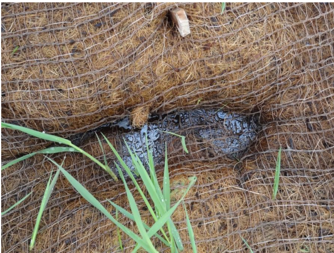
30. Talmadge Creek MP1.0 RDB overbank sheen observed.
