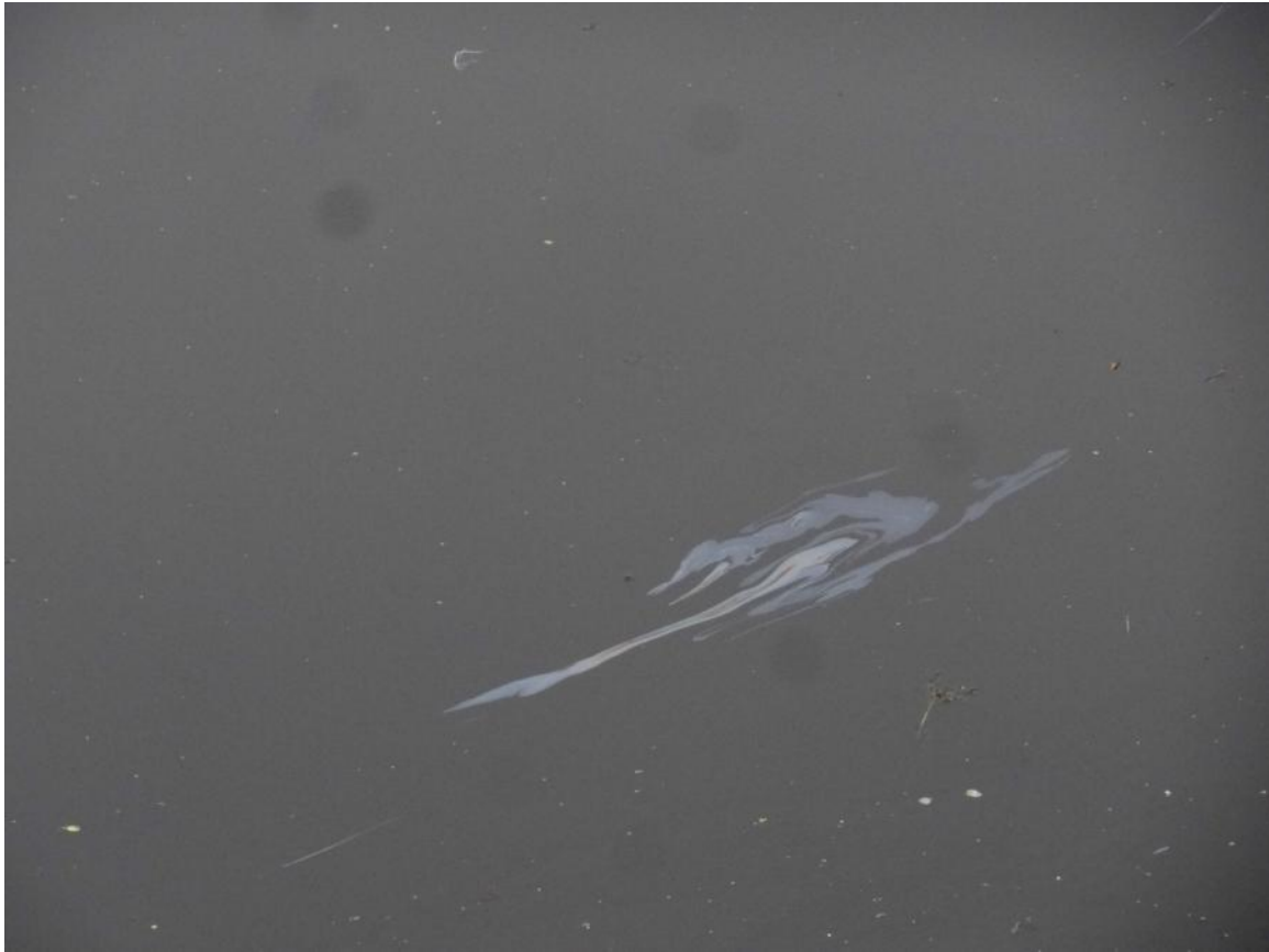
15. Ceresco Dam sheen observed.
