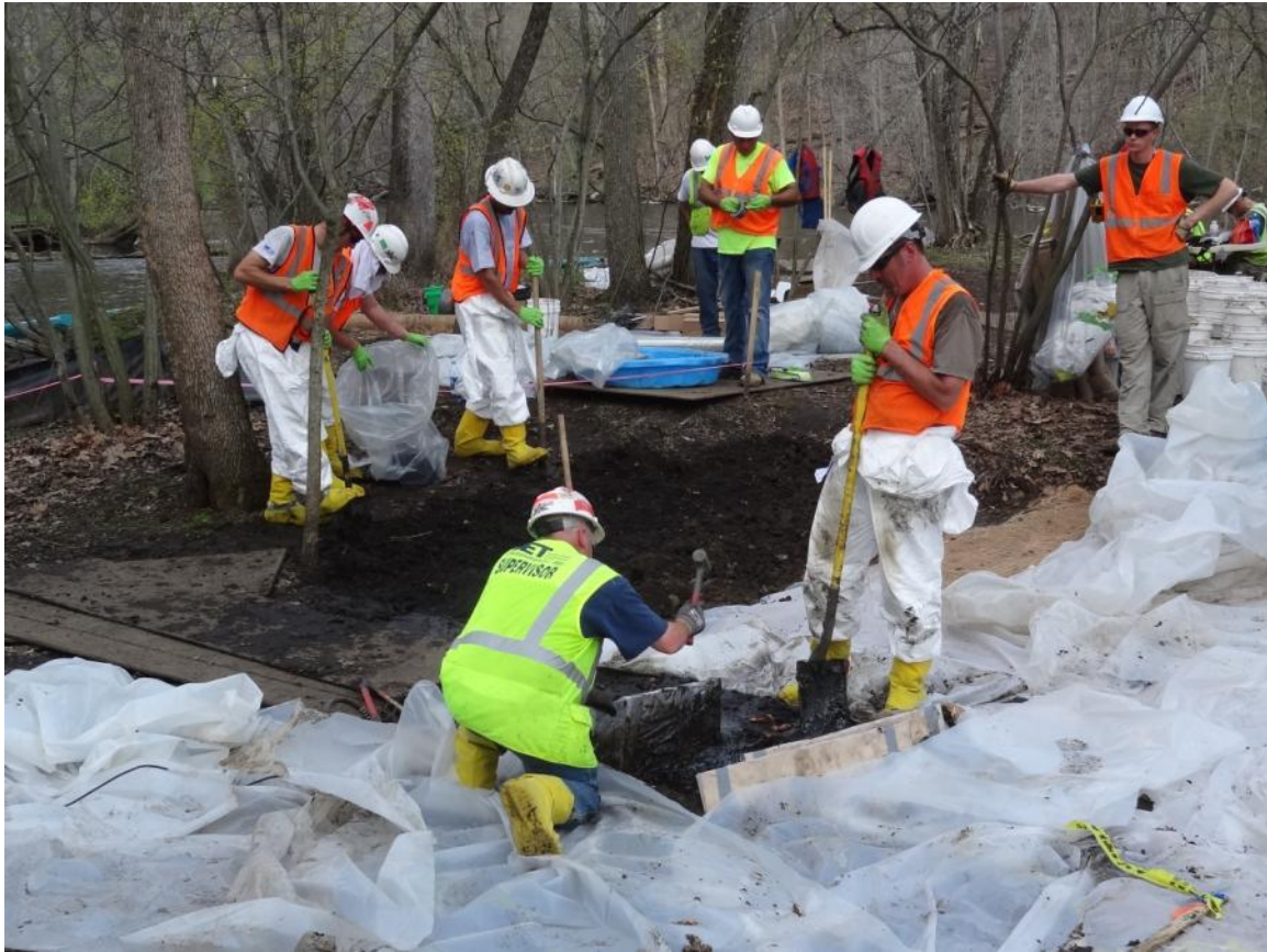
15. OB8.97 I scrape work continued.
