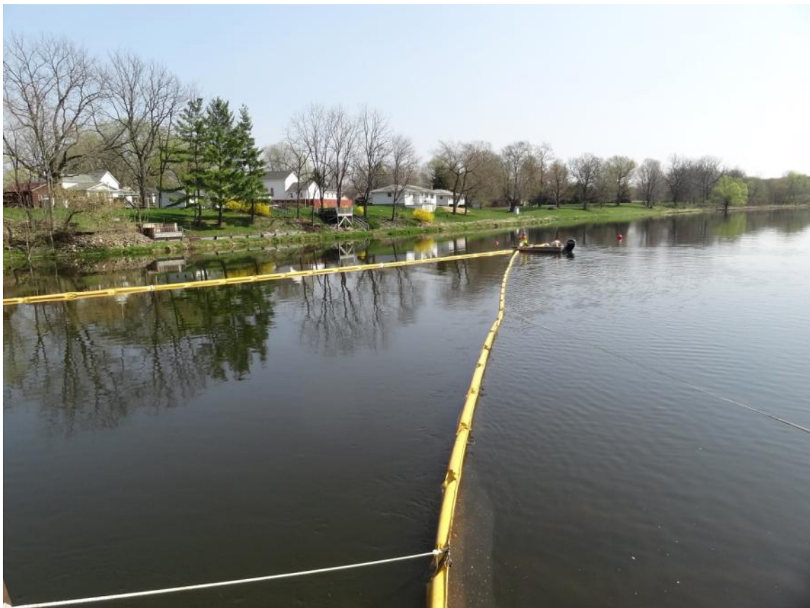
6. Ceresco Dam SWAT crew observed deploying boom.
