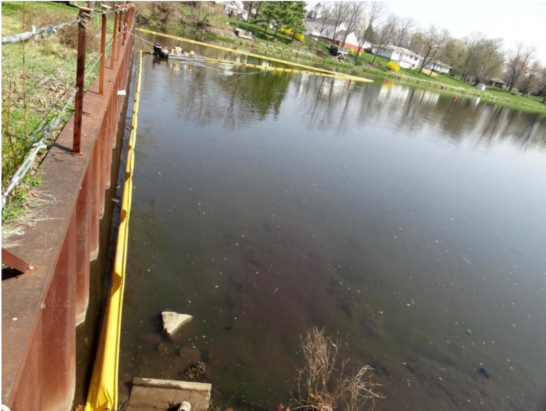
5. Ceresco Dam SWAT crew observed deploying boom.
