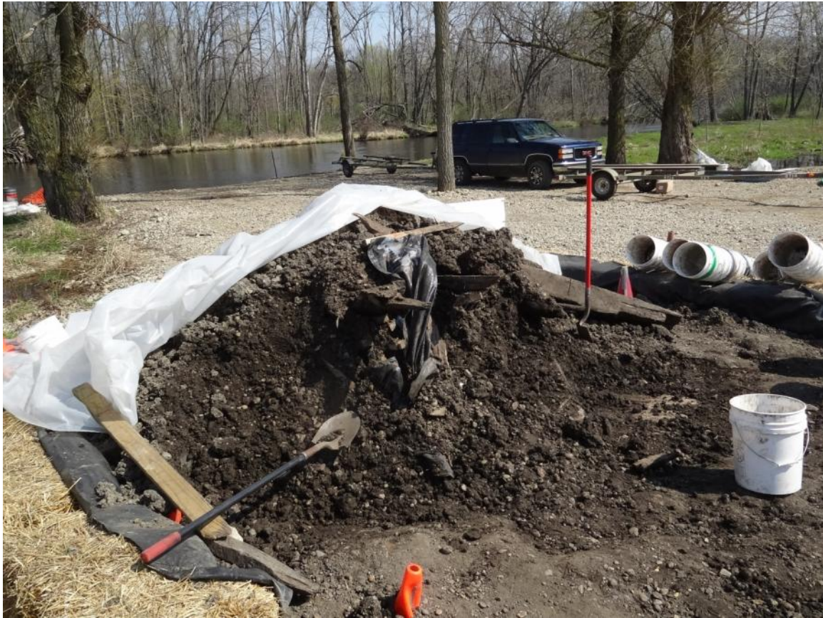
9. OB10.37RDB backfill being utilized.
