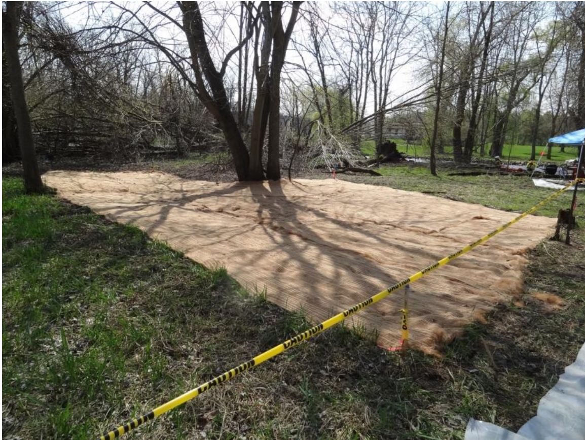
13. OB10.37 RDB restoration of scrape area.
