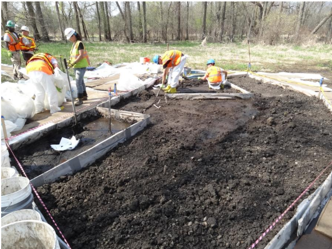
12. OB10.37 RDB scrape work continued.
