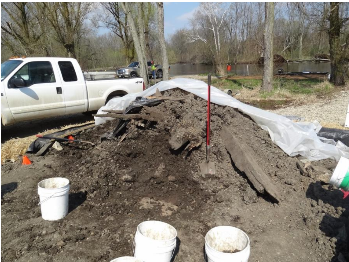
10. OB10.37RDB backfill being utilized.
