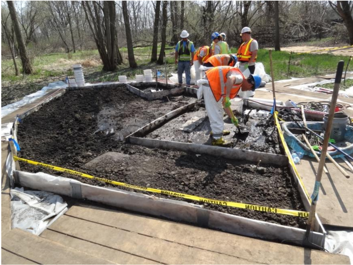
11. OB10.37 RDB scrape work continued.
