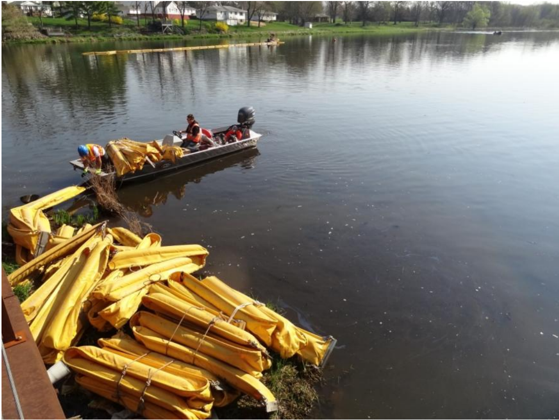
3. Ceresco Dam SWAT crew observed deploying boom.
