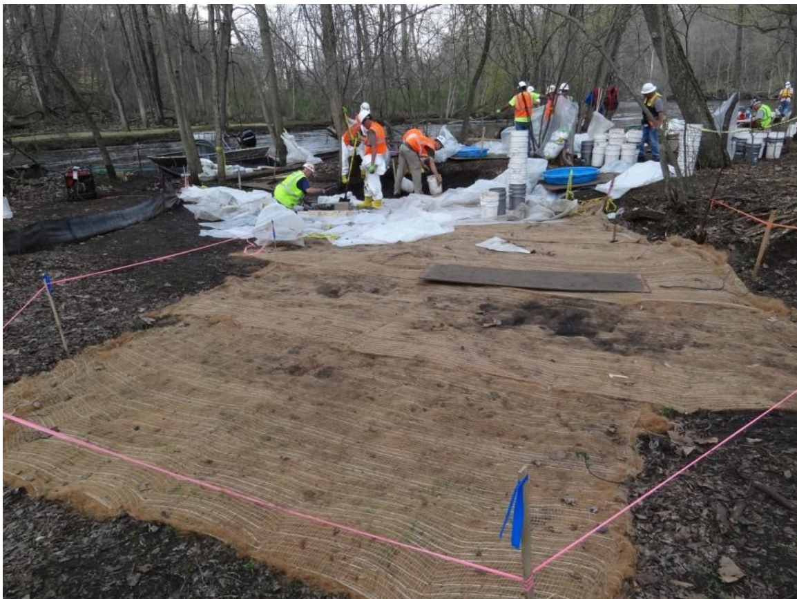
14. OB8.97 I scrape work continued.
