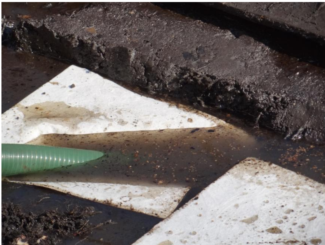
19. Scrape at OB 8.97 dewatering.
