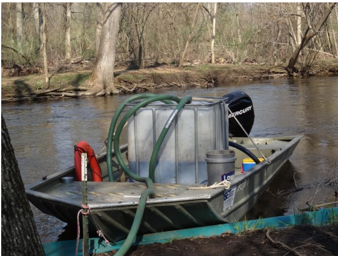
20. Scrape at OB 8.97 dewatering into tote on boat.
