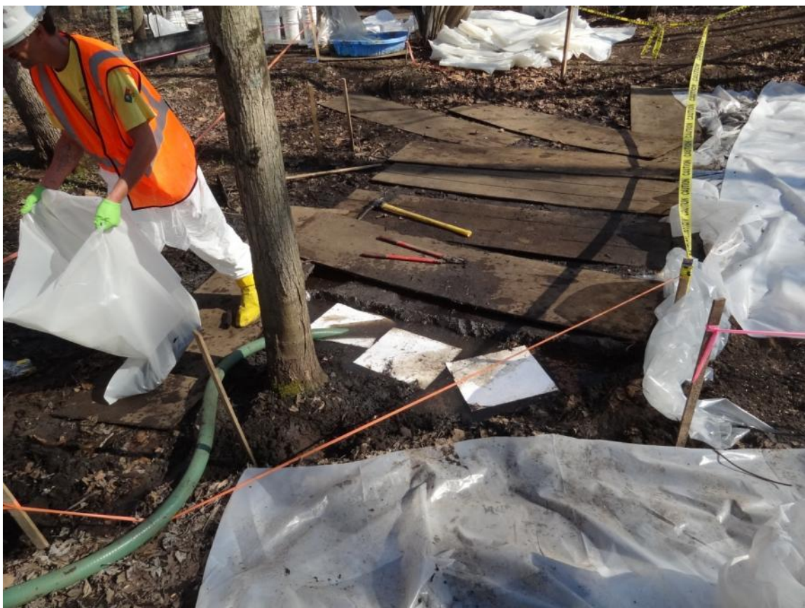
18. Scrape at OB 8.97 dewatering.
