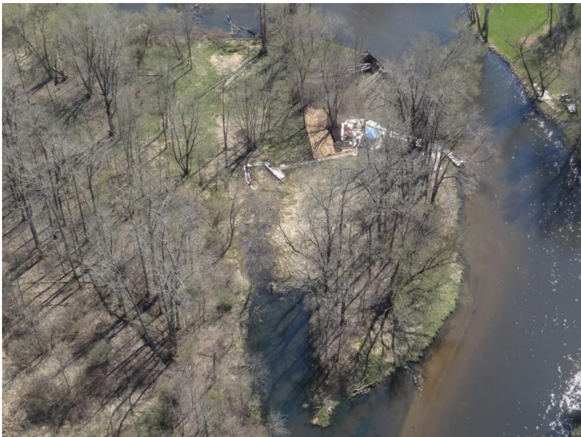
22. Scrape work at OB10.37 continues.
