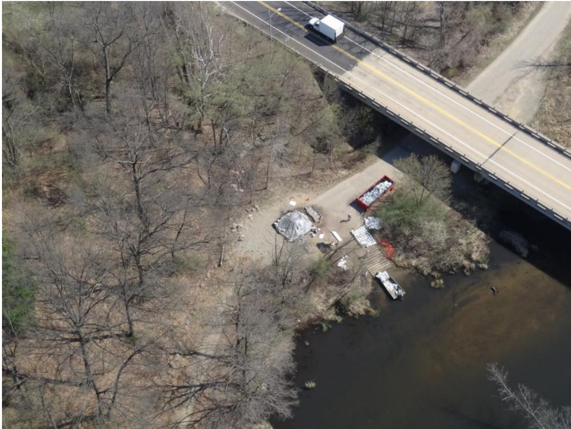
21. Historic Bridge Park soil staging area for the OB8.97.
