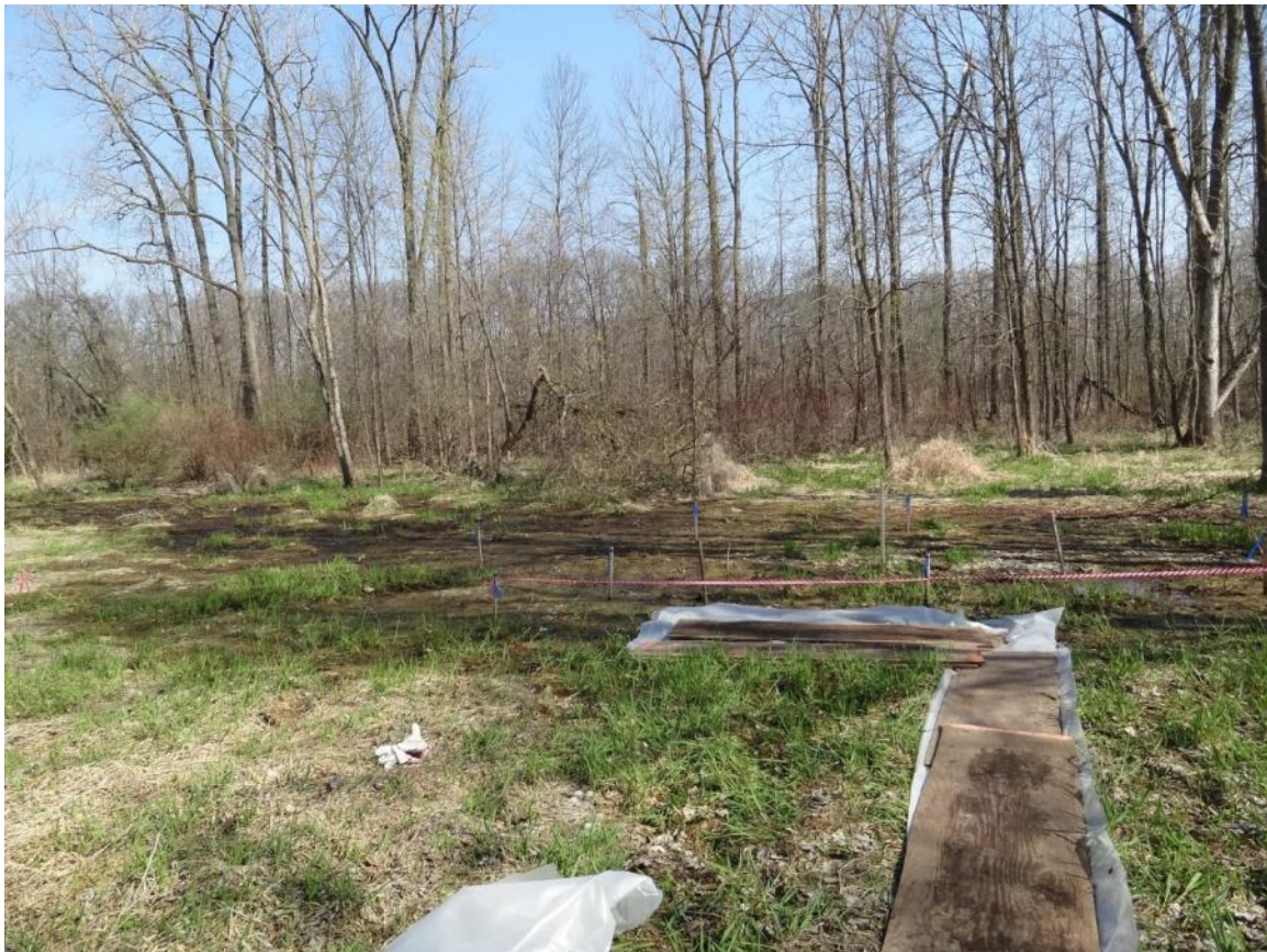
24. Scrape work at OB10.37 RDB continues.
