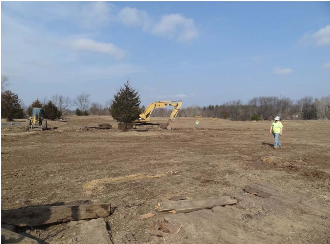
4. Crews removing last of timber mats at Former Turbidity Control System location.
