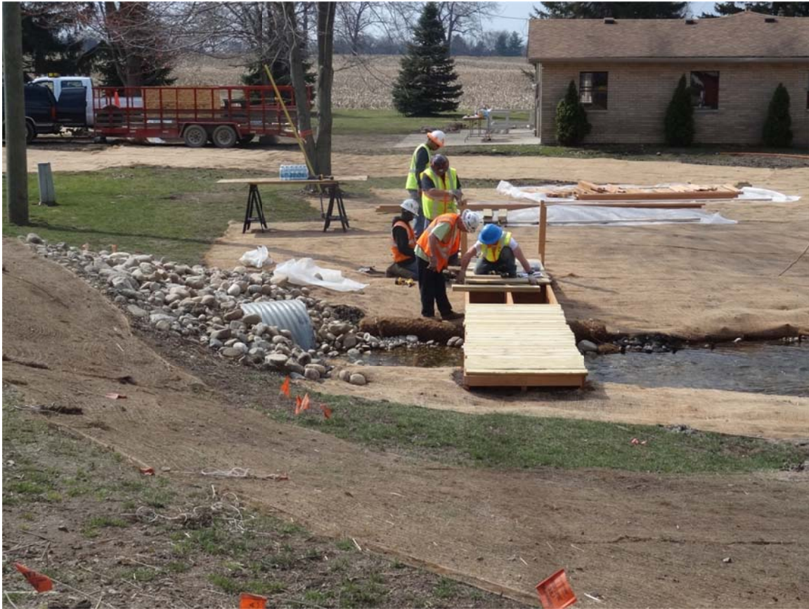
11. Confluence, crews installing new bridge across Talmadge Creek in afternoon.
