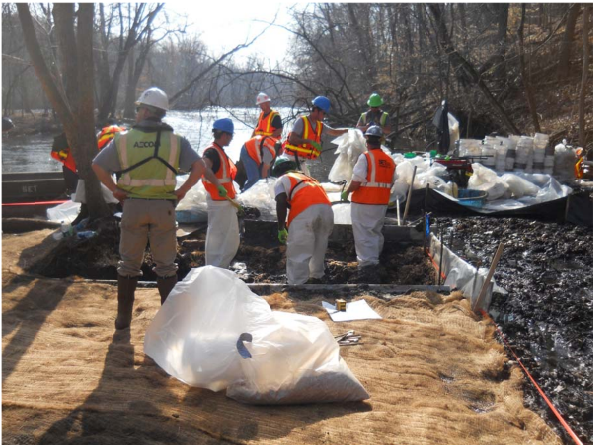
14. OB 9.10 LDB, scrape work continues.
