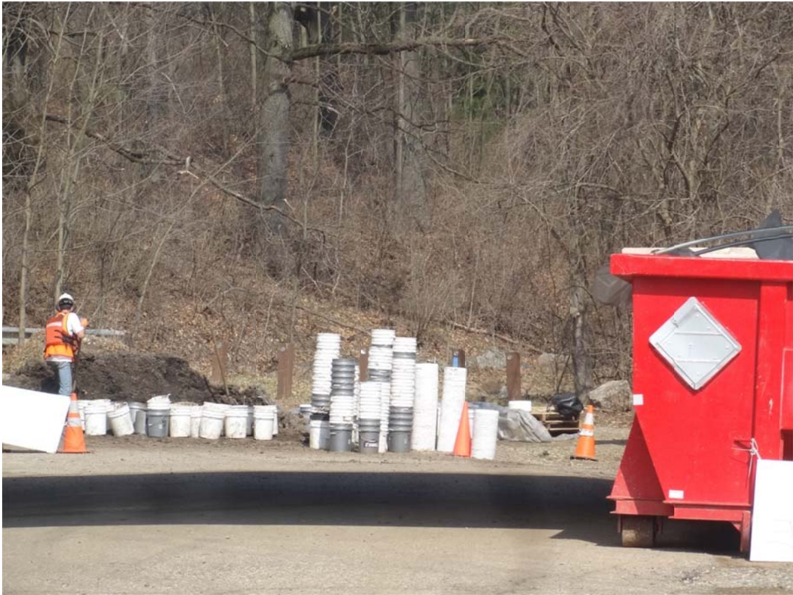
17. Historic Bridge Park, soil/water loading area for soils scraped from OB 9.10 LDB.
