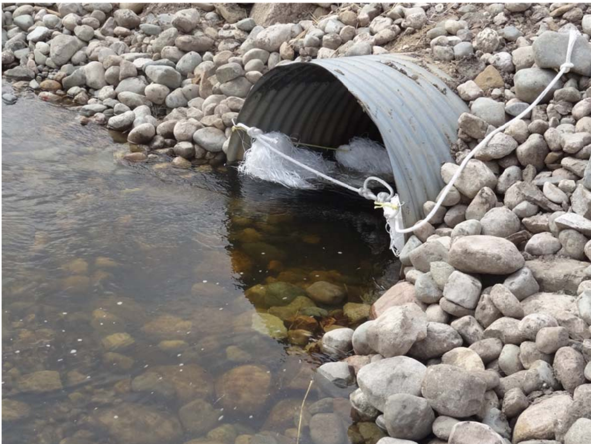
12. Confluence, snare boom installed in culvert on south side of A Drive.
