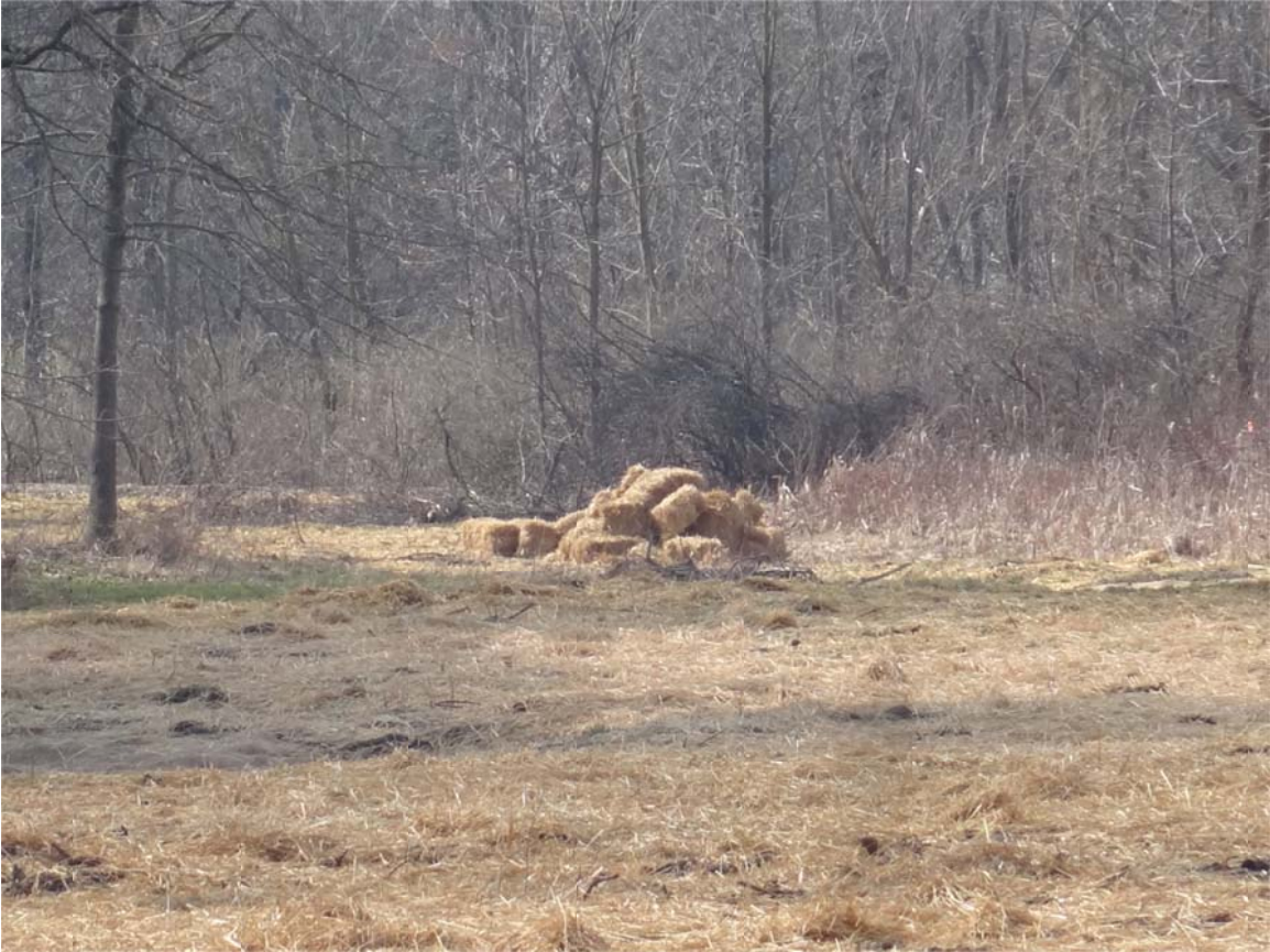
7. Talmadge Creek: additional straw bales staged on south side of creek.
