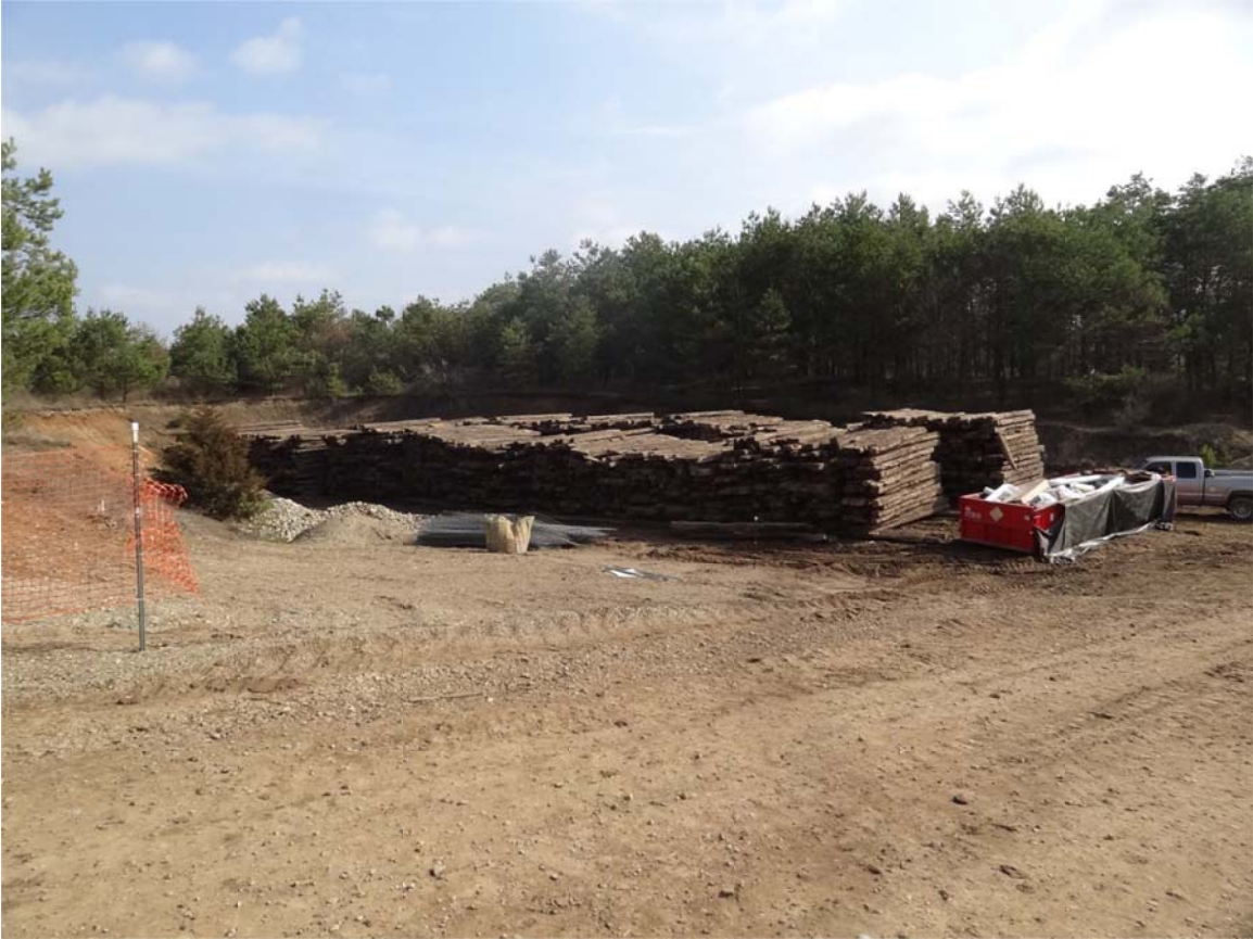
3. Timber mats staged east of former Turbidity Control Structure location.
