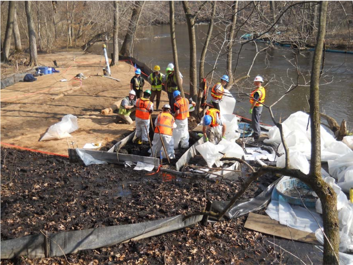
15. OB 9.10 LDB, scrape work continues.
