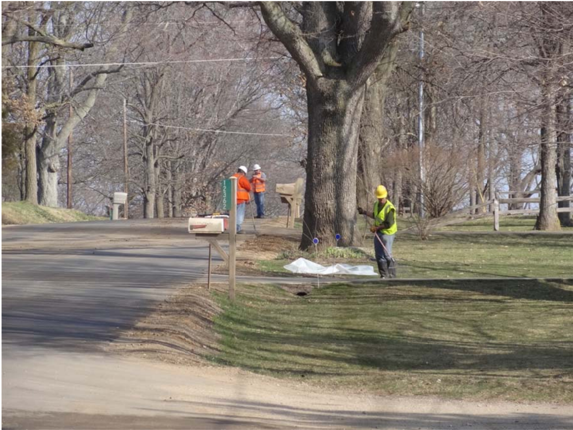
1. Crews conducting roadside/mailbox cleanup along residences on 15-1/2 Mile Road.
