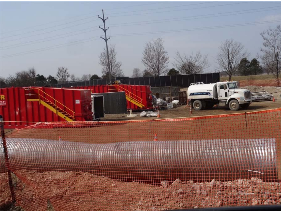
20. Frac Tank City southern decon pad, crews cleaning a frac tank.
