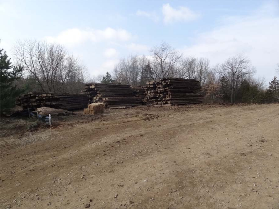
5. Timber mats staged south of former Turbidity Control System.
