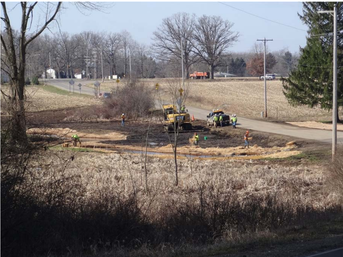
6. Restoration work south of A Drive, upstream from Confluence.
