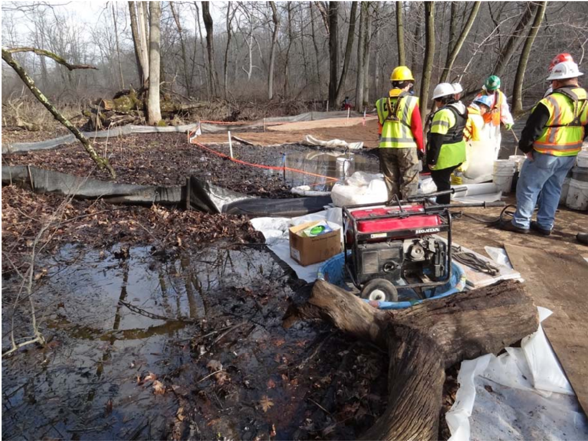
15. OB 9.10 LDB, scrape work continues.
