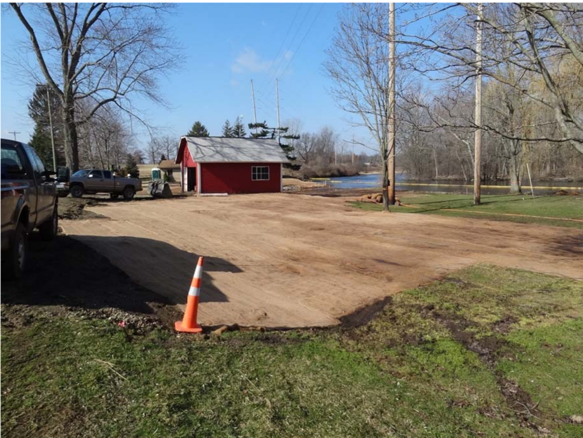
10. Confluence, former soil mixing box location.
