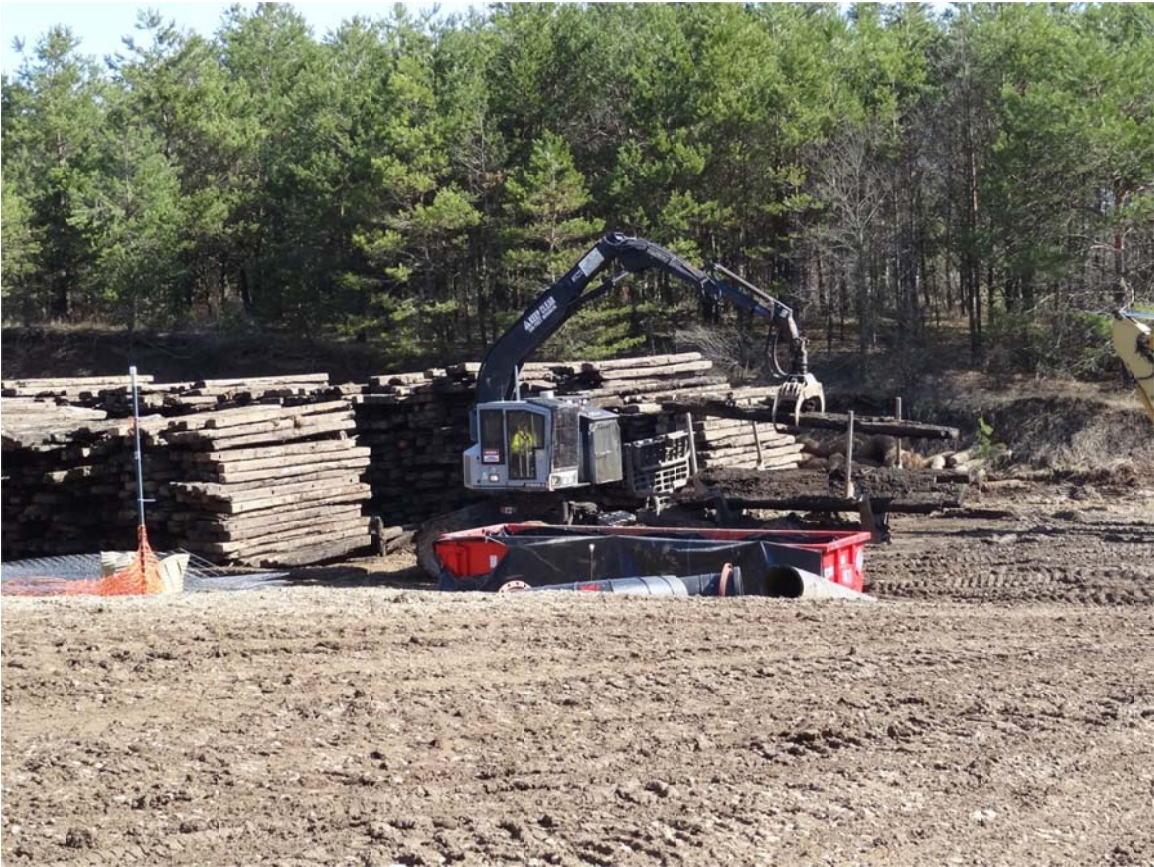
3. Crews continue mat removal and staging at former Turbidity Control Structure location.
