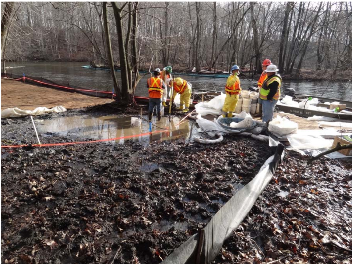
14. OB 9.10 LDB, scrape work continues.
