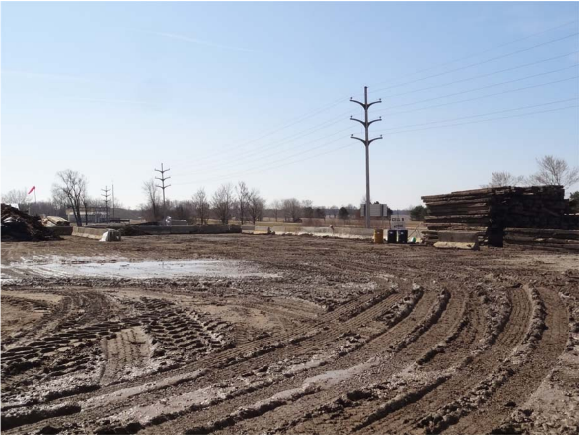
21. Frac Tank City Cell B, no material or activity observed.
