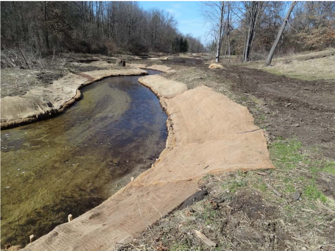
2. Talmadge Creek, restoration along creek west of 15-1/2 Mile Road.
