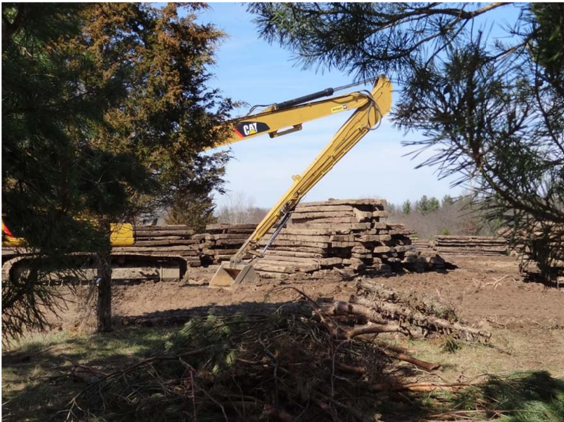
4. Stacked mats at former Turbidity Control Structure location.
