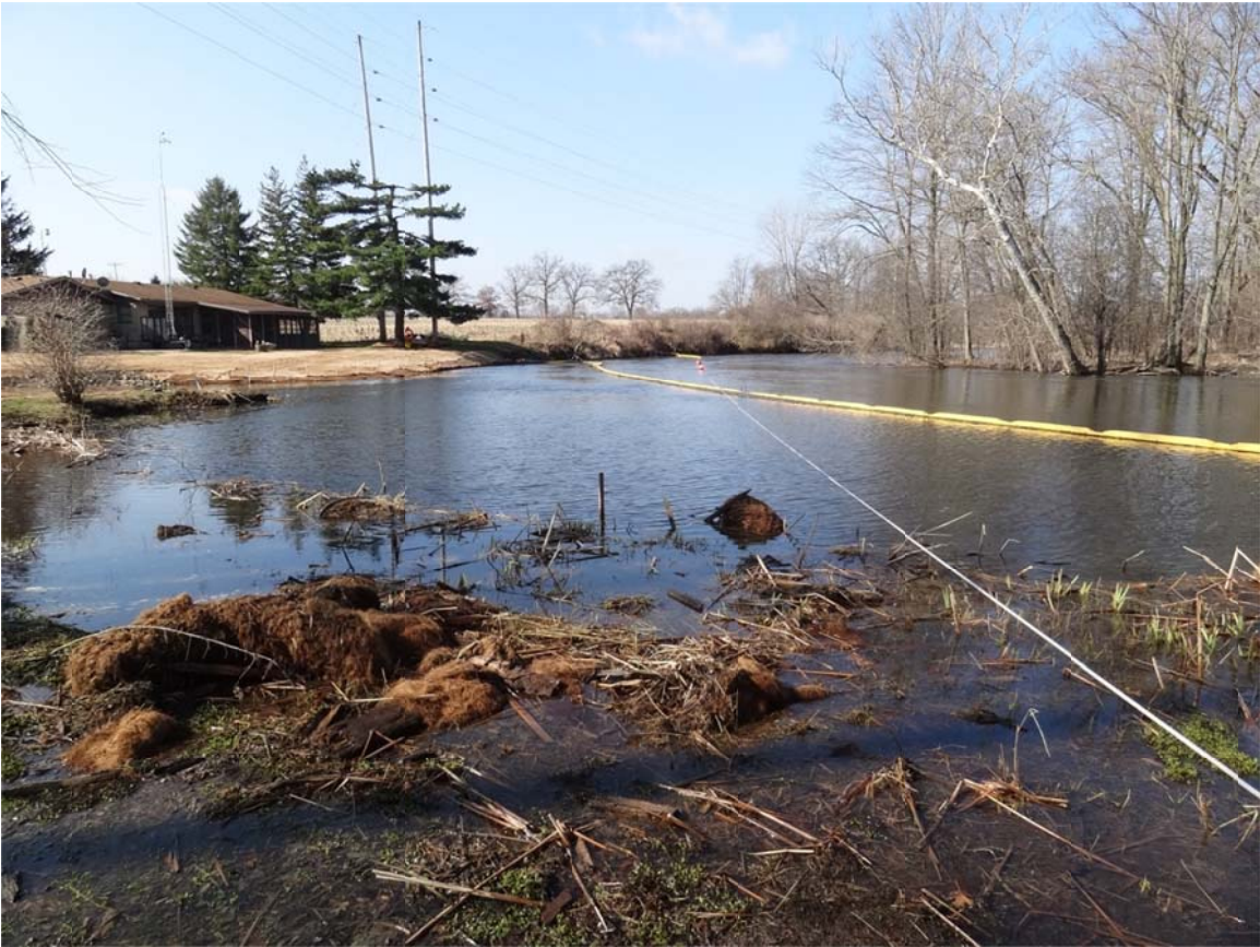
9. Confluence, restoration work complete.
