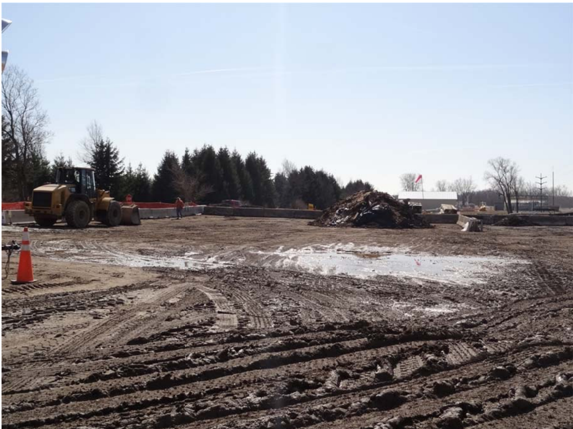
20. Frac Tank City cell A, one soil pile present.
