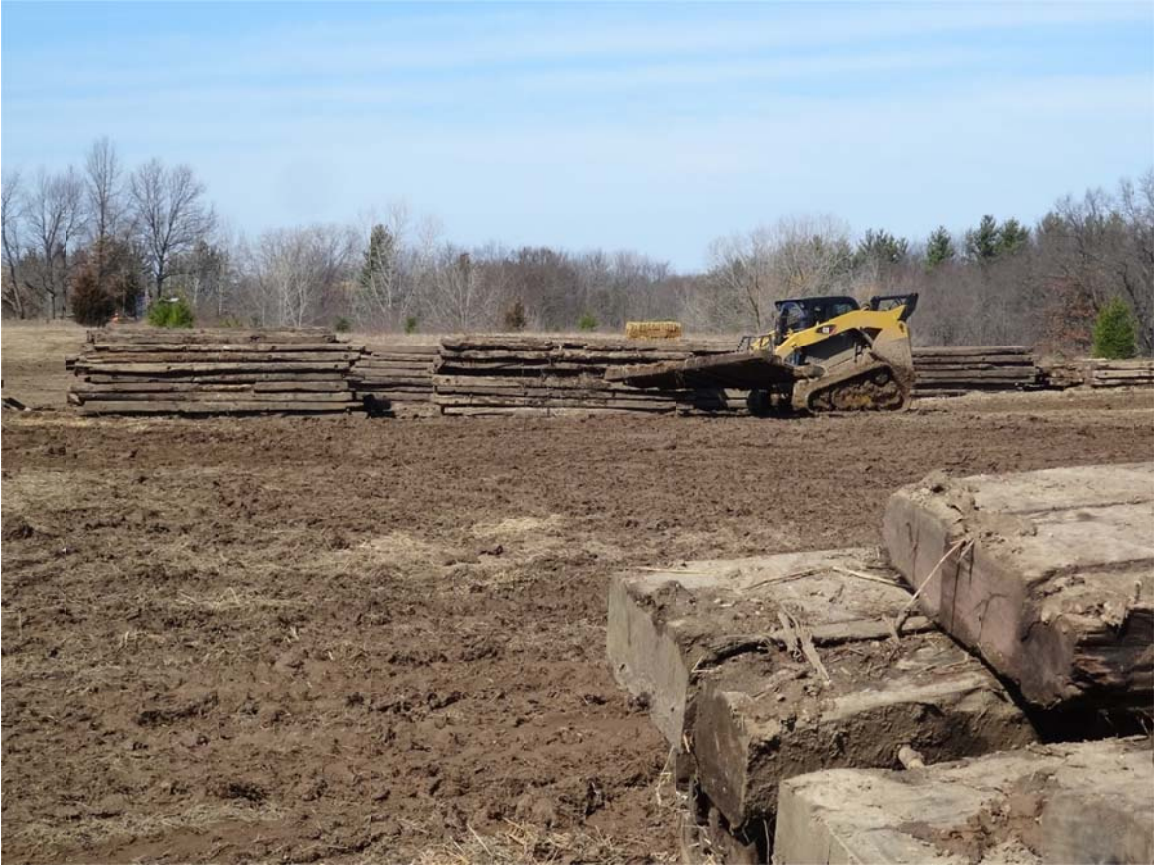
5. Crews stacking mats at Former Turbidity Control System location.
