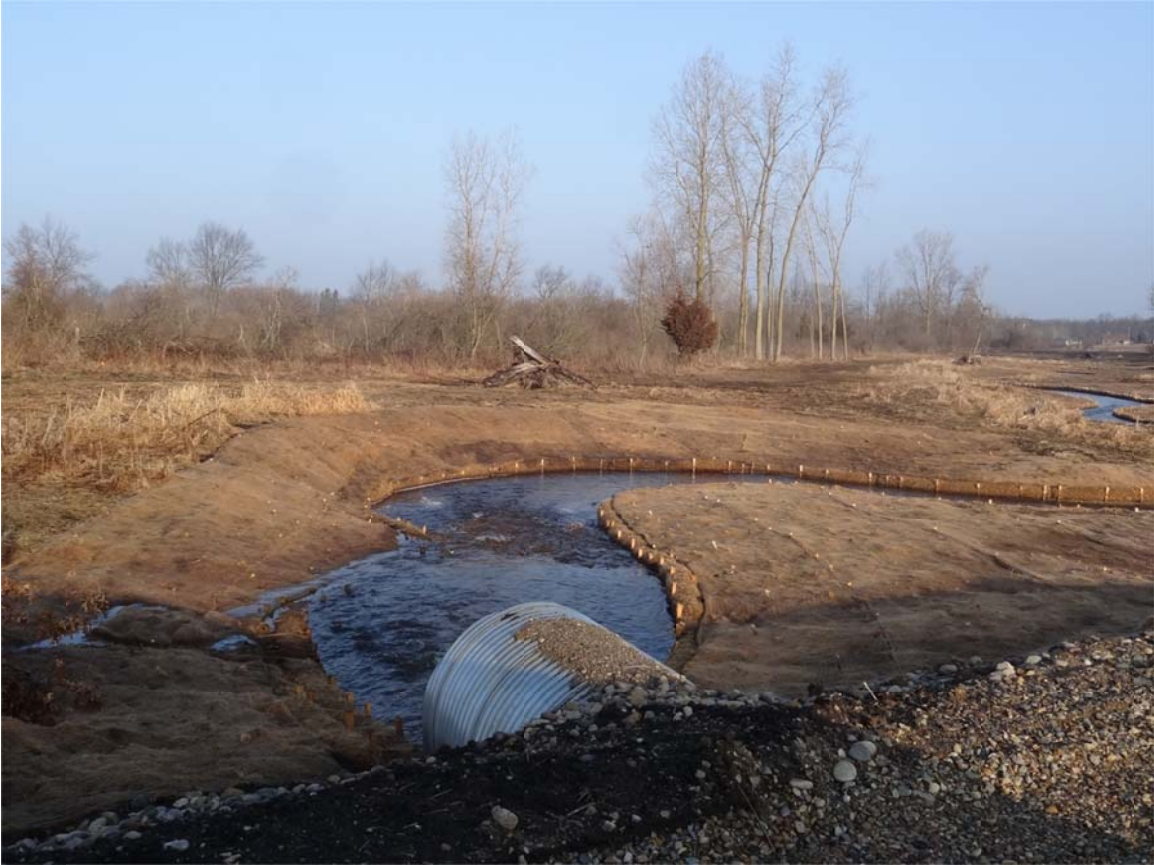
1. Talmadge Creek near MP 1.0, looking northwest.
