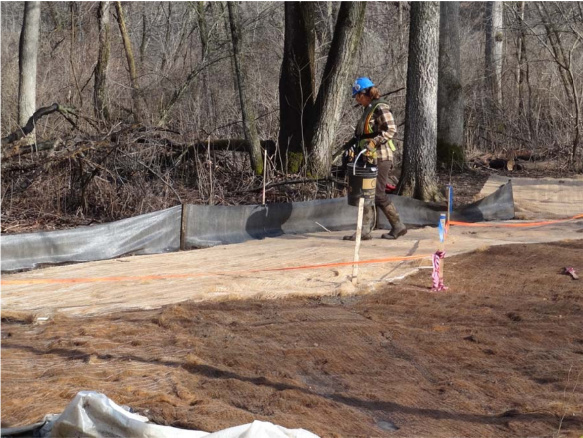
17. OB 9.10 LDB, restoration work.
