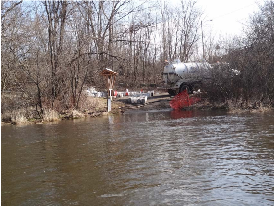
19. Historic Bridge Park, soil/water loading area for soils scraped from OB 9.10 LDB.
