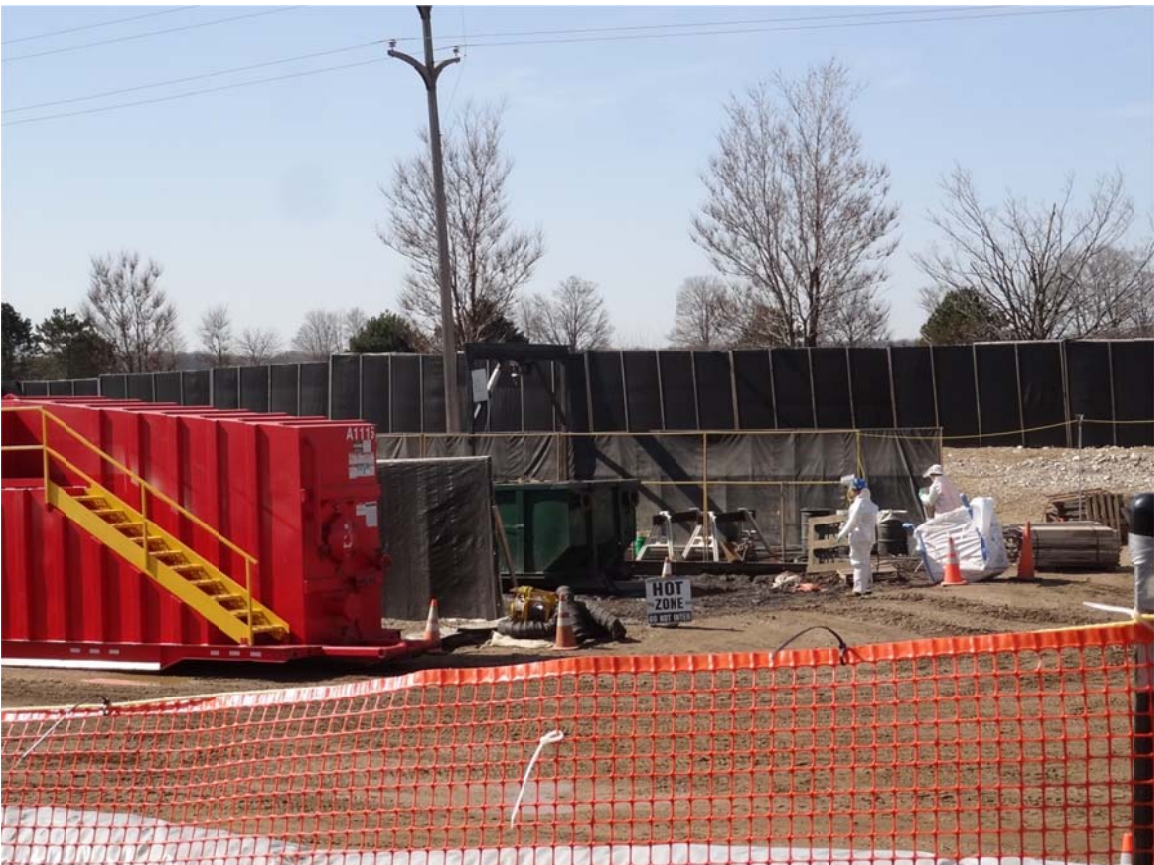
22. Frac Tank City southern decon pad, crews cleaning sheet pile panels and equipment.
