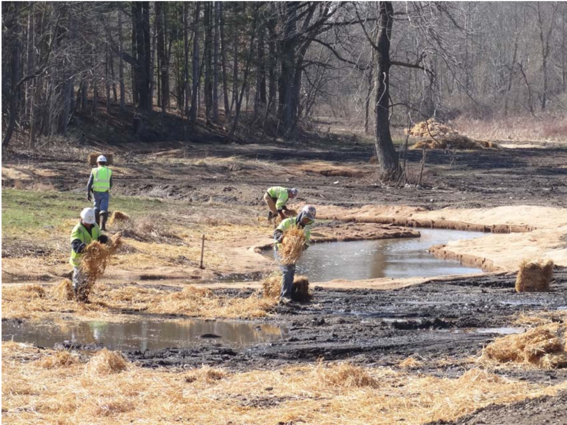
7. Talmadge Creek: crews spreading straw south of A Drive at Confluence.
