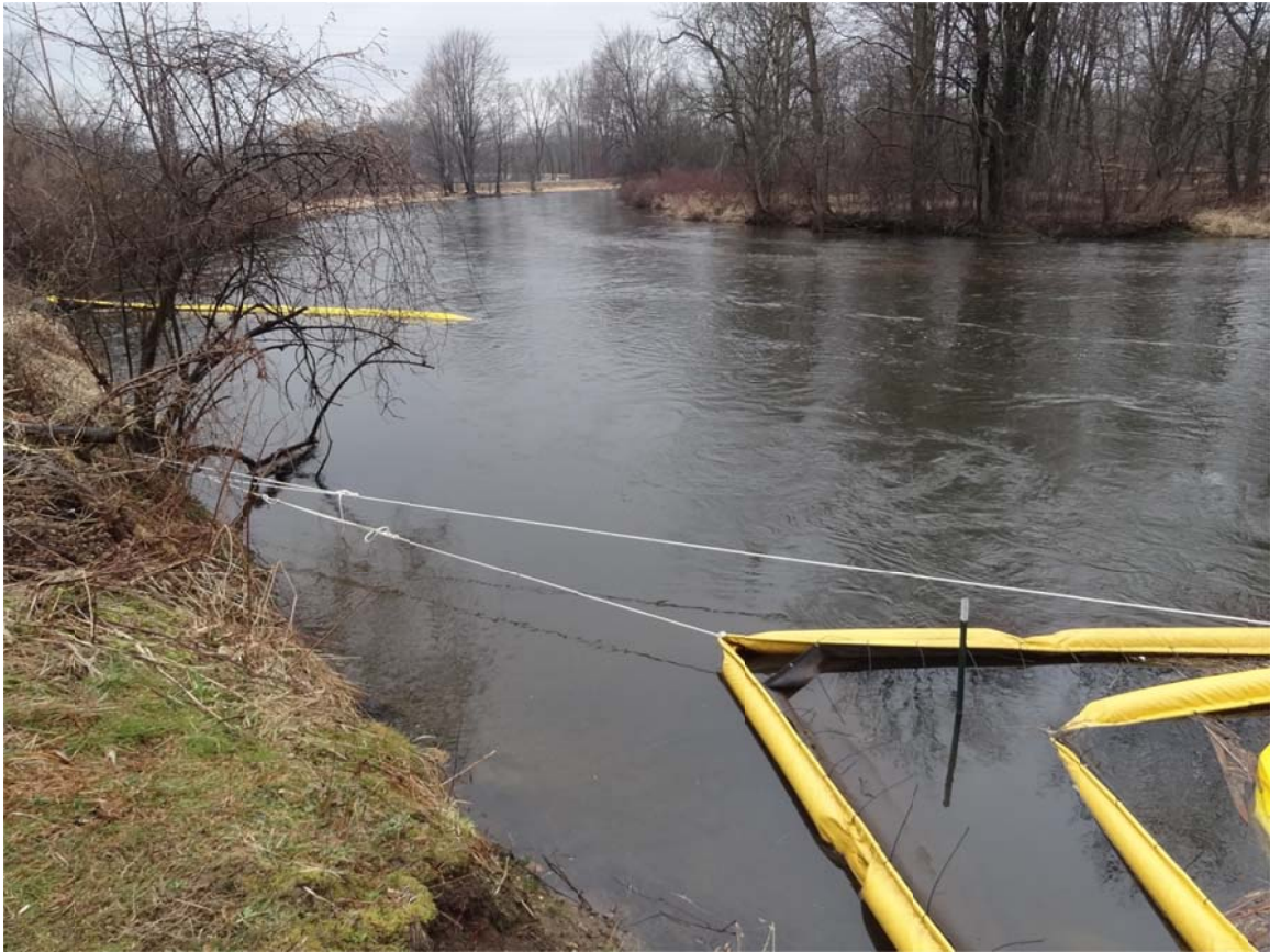
15. Confluence: containment boom in place at Talmadge Creek discharge.
