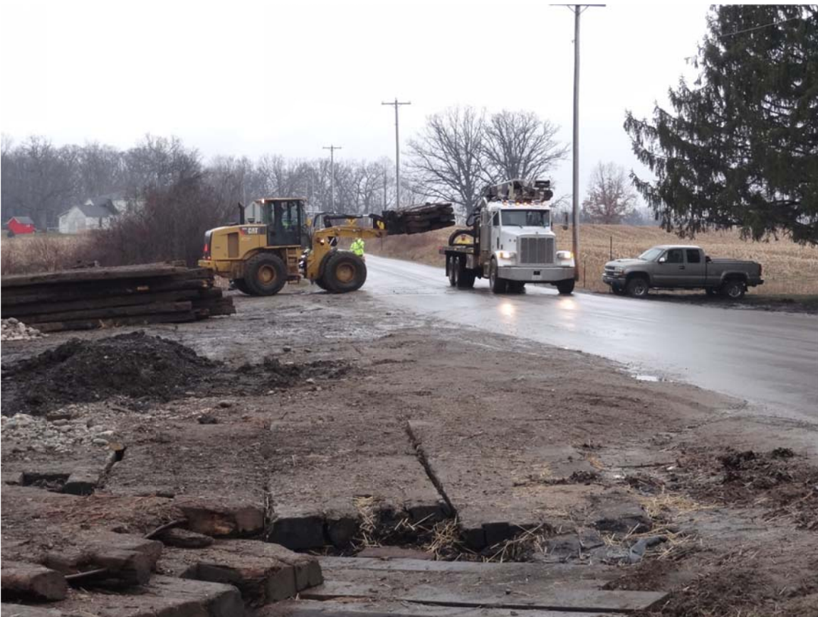
8. Talmadge Creek: crews loading mats onto truck on A Drive at Confluence.
