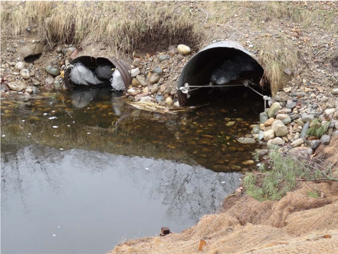
1. Talmadge Creek, sweeper boom installed in culvert on east side of 15-1/2 Mile Road.
