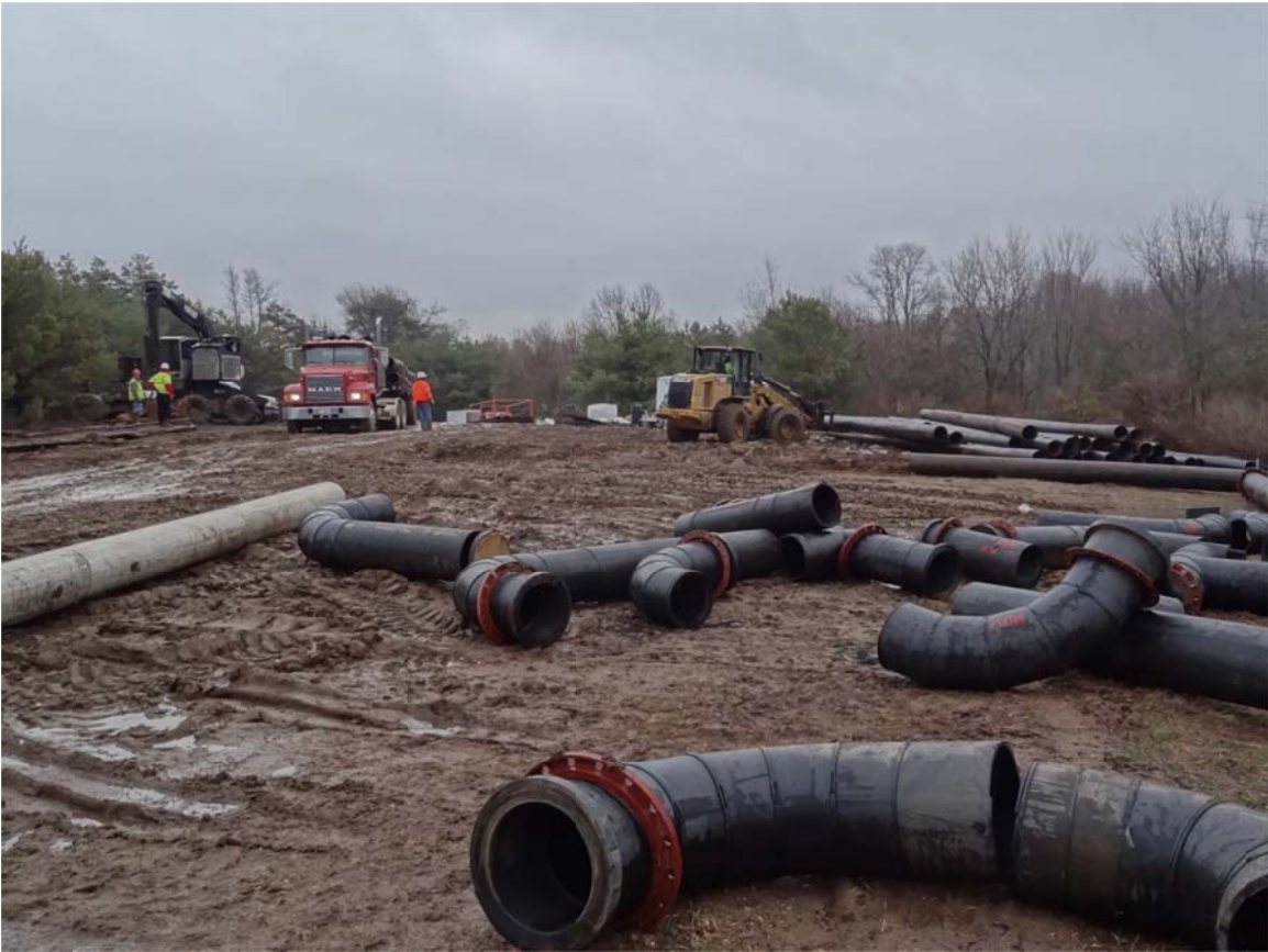
5. Crews loading Turbidity Control System piping onto trucks near 15-1/2 Mile Road.
