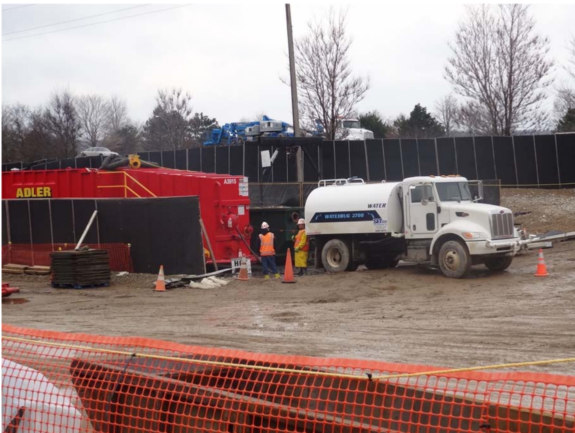
22. Frac Tank City southern decon pad, crews cleaning a frac tank and roll-off box.
