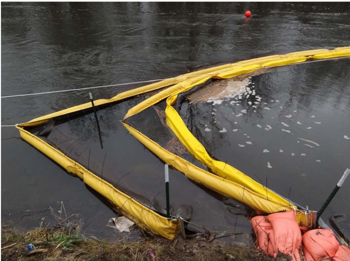
16. Confluence: minor debris observed within containment boom.
