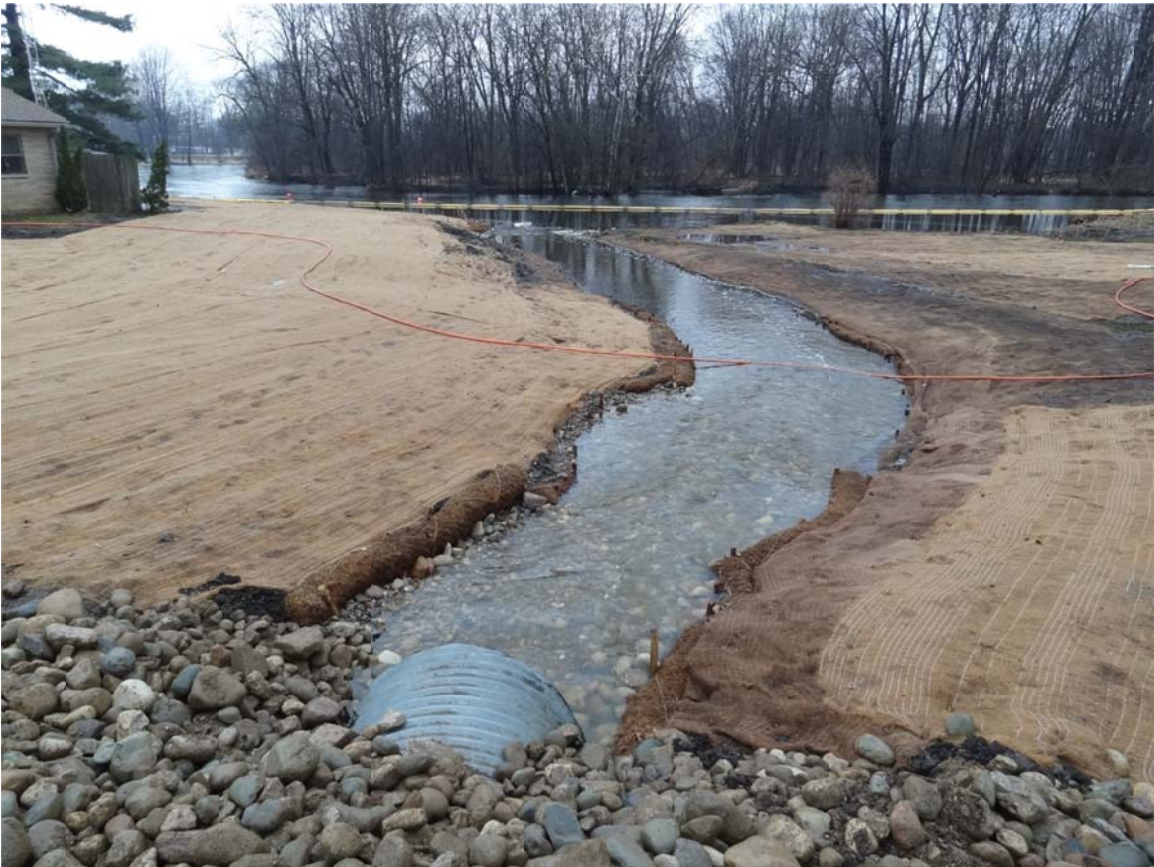
9. Talmadge Creek: restoration work continues at Confluence.
