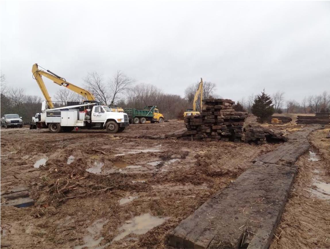
3. Crews continue mat removal at former Turbidity Control Structure location.
