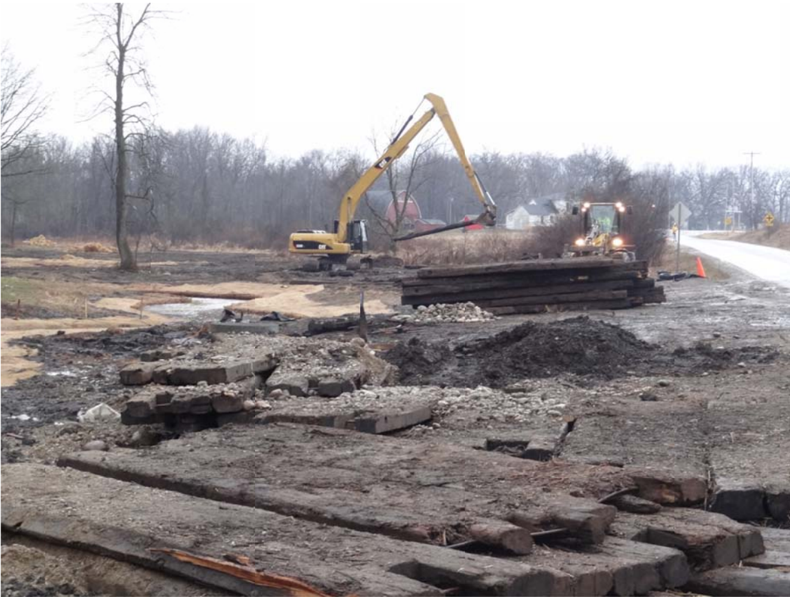
7. Mat road removal continues south of A Drive, upstream from Confluence.
