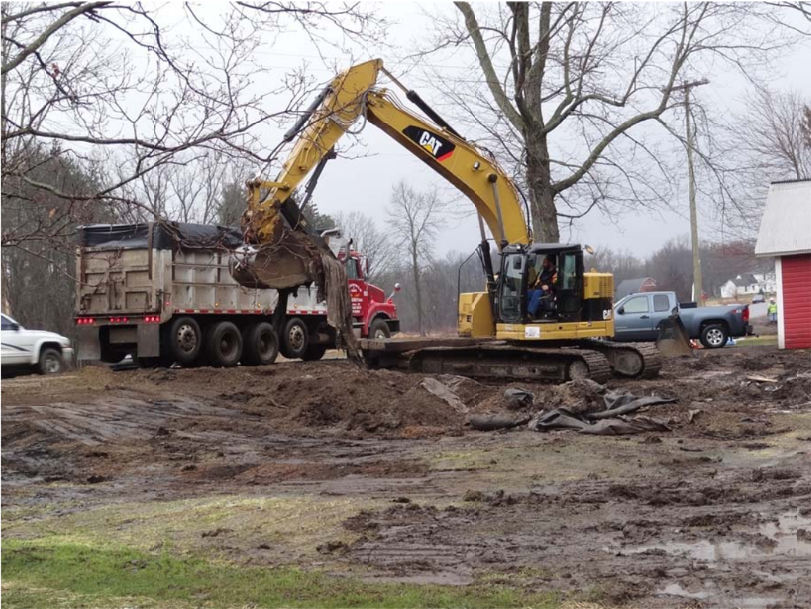
11. Confluence, crews excavating former soil mixing box location.
