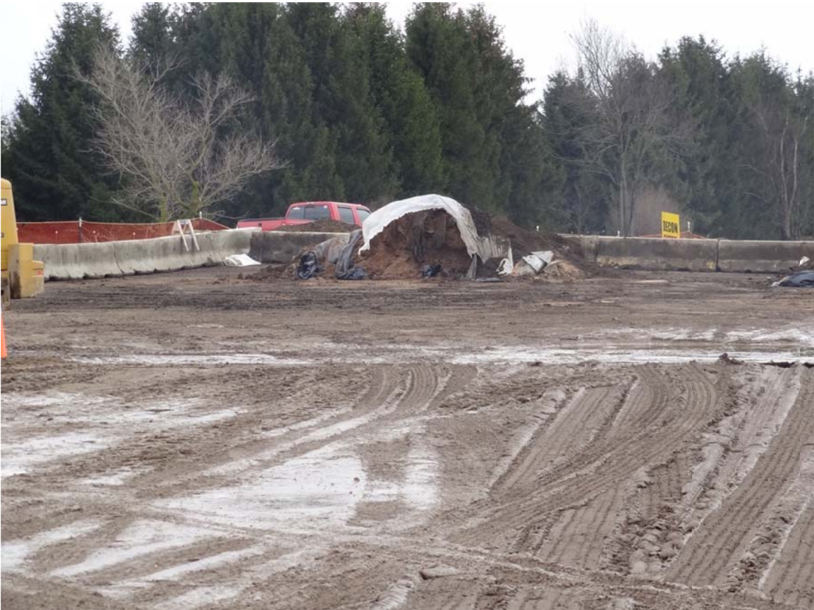
20. Frac Tank City Cell A, only two small piles of soil present in cell.
