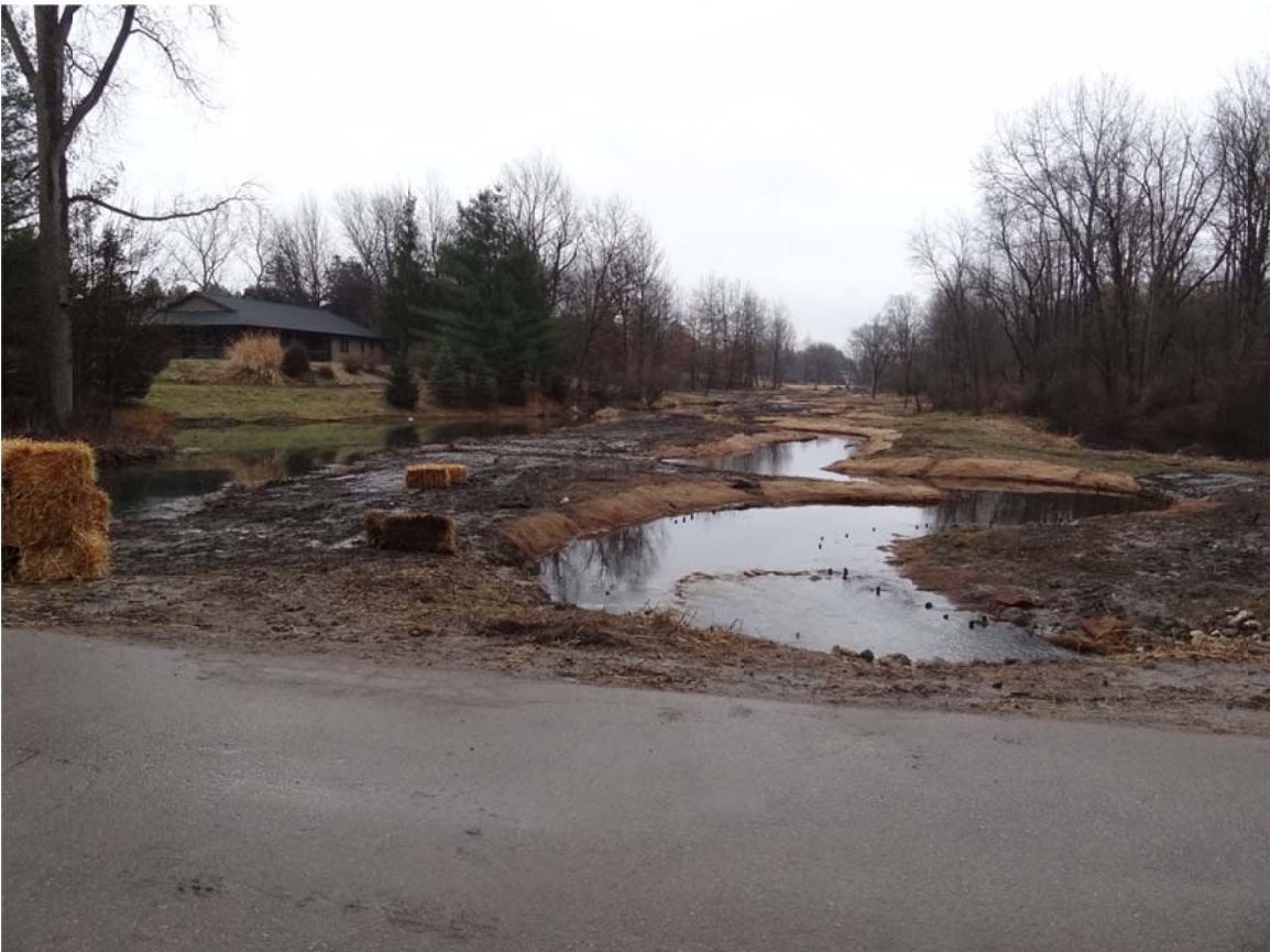
6. Talmadge Creek: restoration work near MP1.5.
