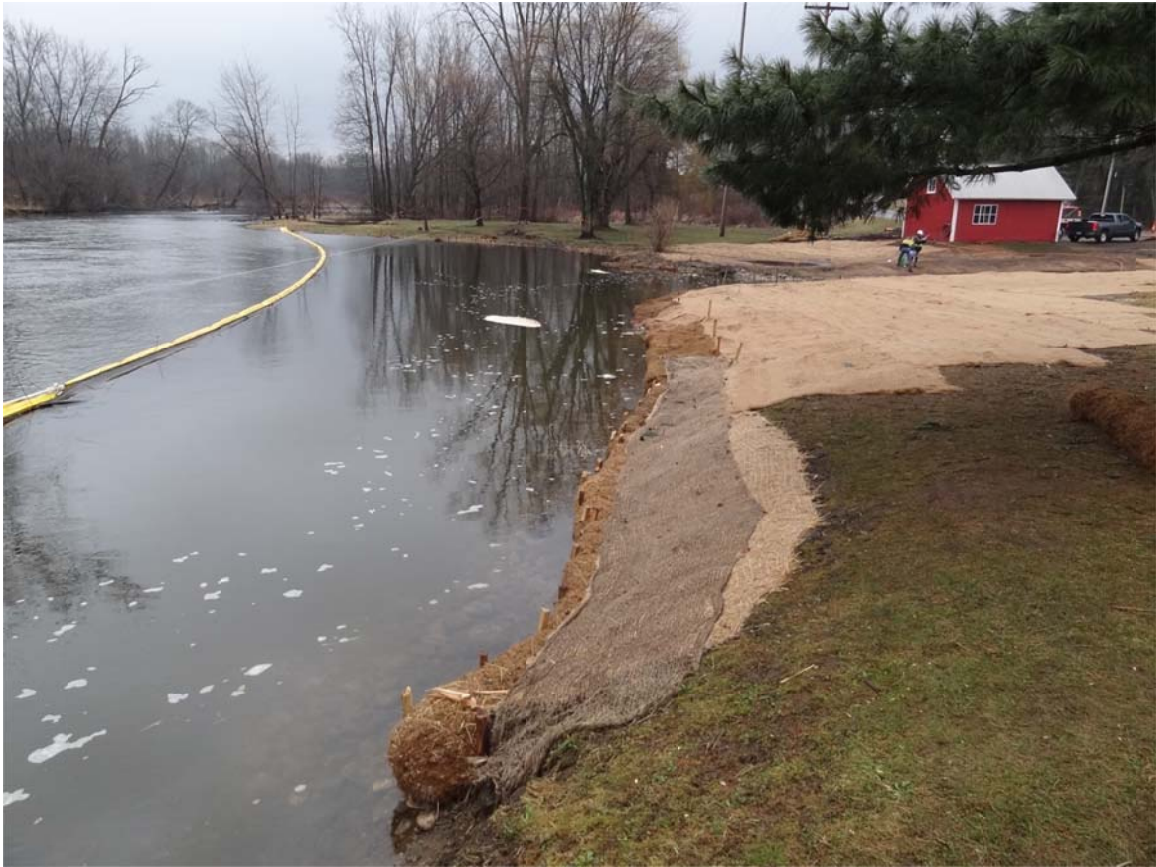
17. Confluence: restoration work along river shoreline.
