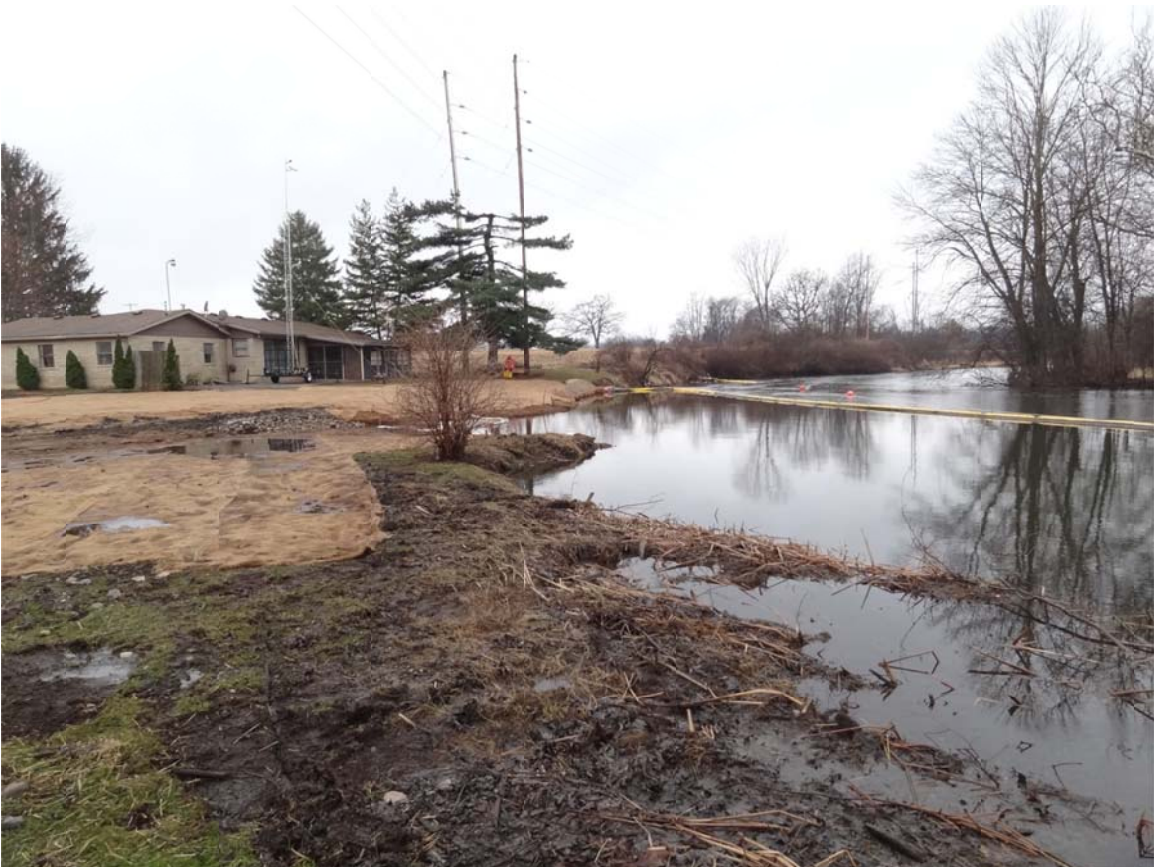
10. Confluence, restoration work almost complete.
