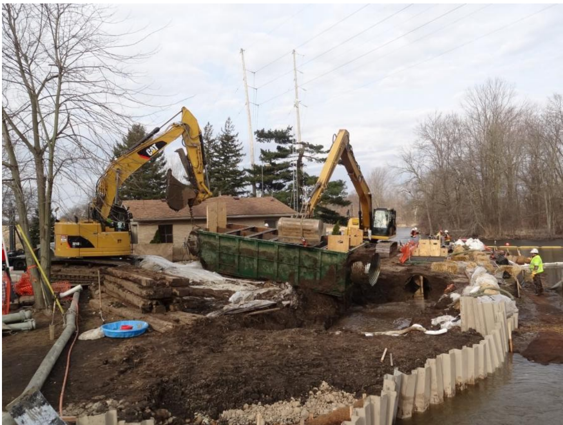
19. Confluence: observed the removal of the first diversion box.
