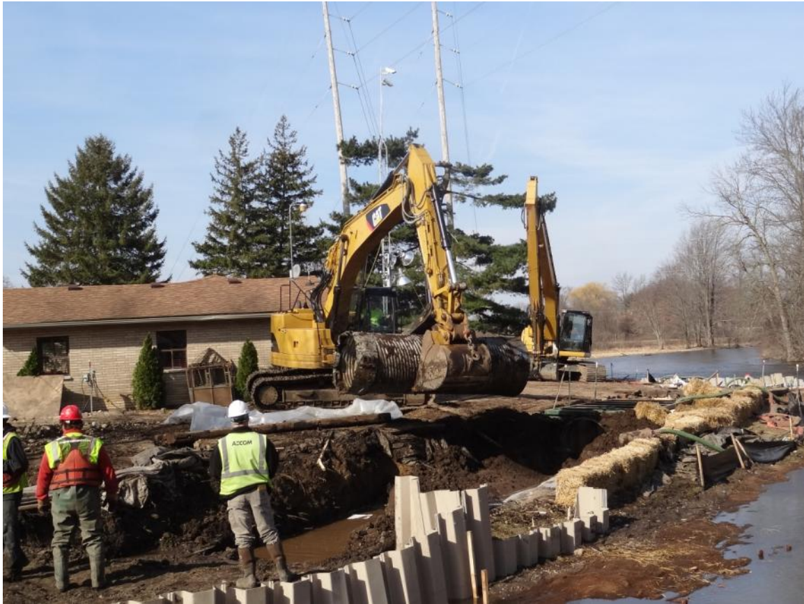
23. Confluence: observed removal of the diversion structure culvert that connected the two boxes.
