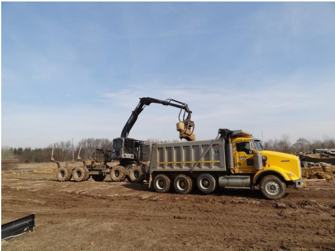
4. Turbidity Control Structure observed being demobilized.
