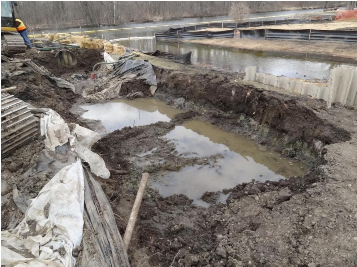
26. Confluence: removal of the diversion structure.
