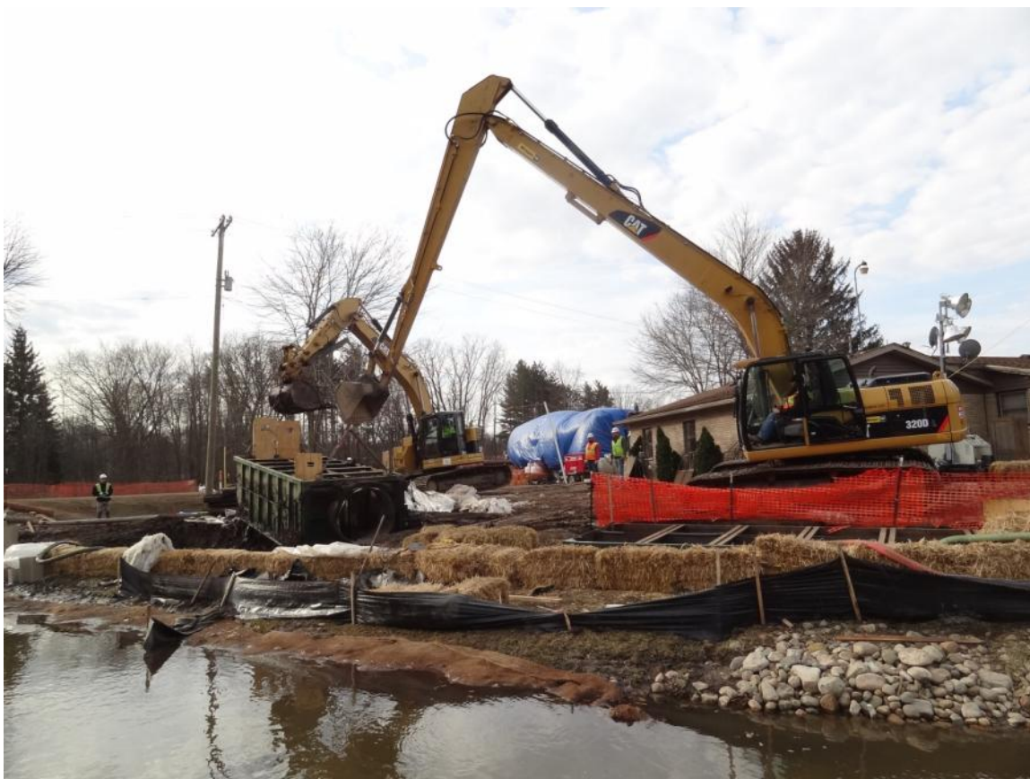
18. Confluence: observed the removal of the first diversion box.
