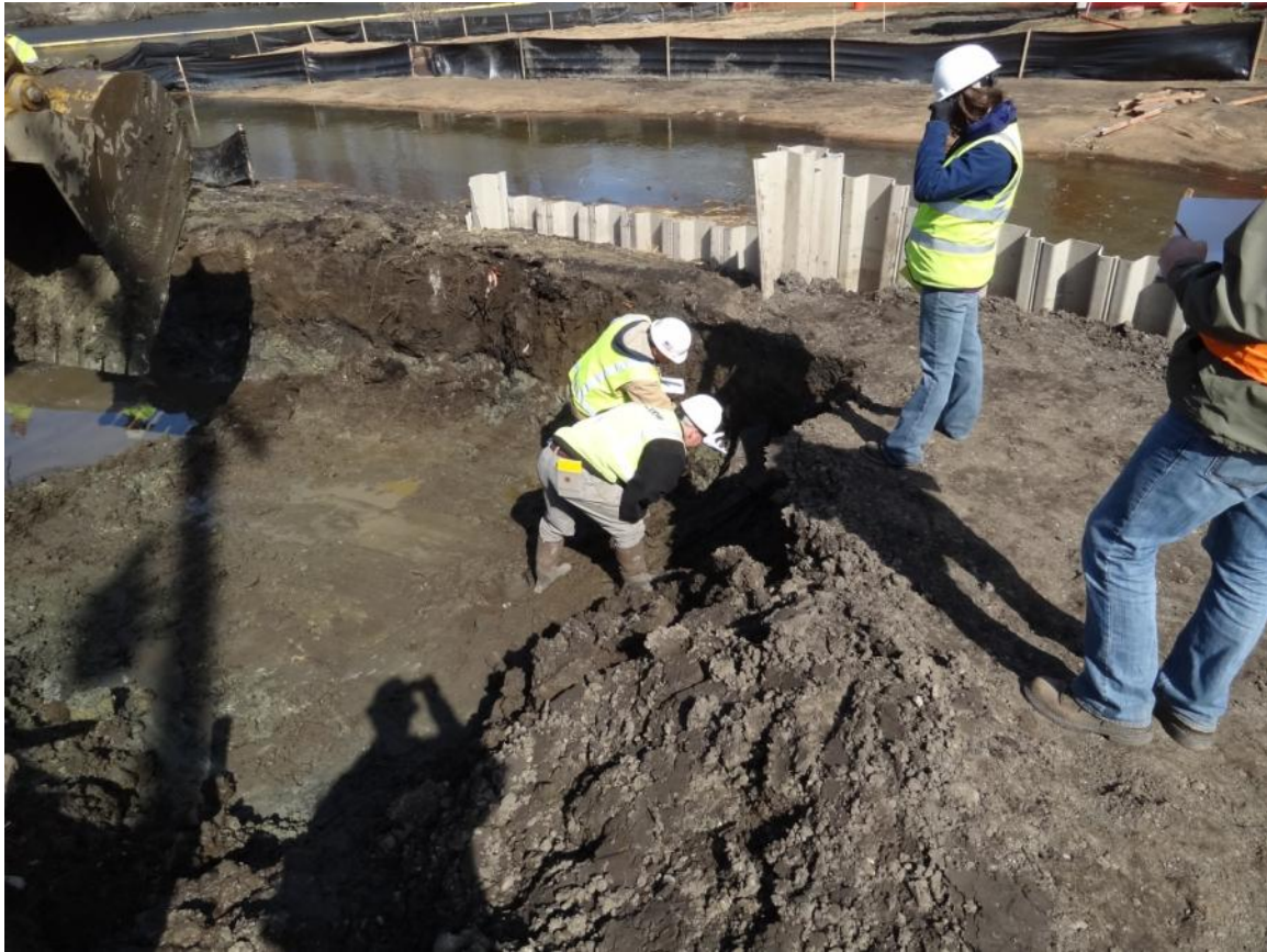
27. Confluence: during the removal of the diversion structure crews cleared the excavation prior to sampling.
