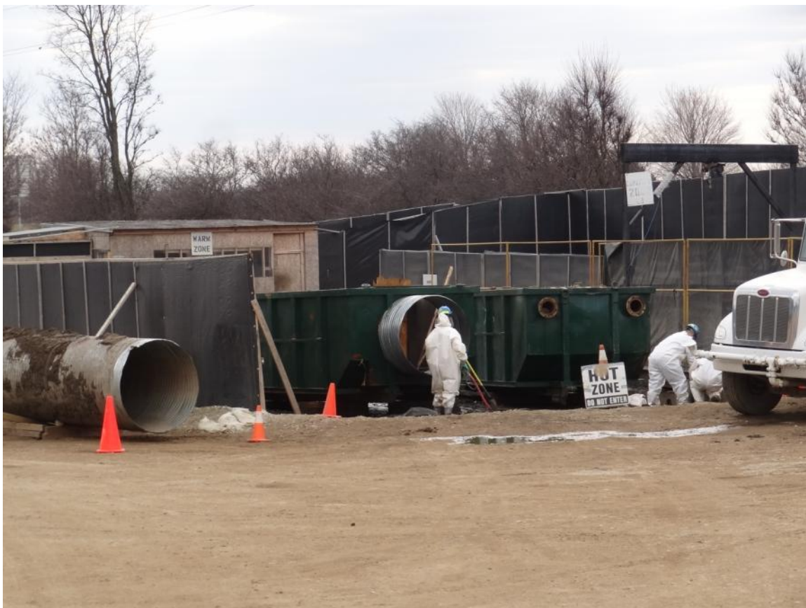
37. . Frac-City observed crews decontaminating diversion box.
