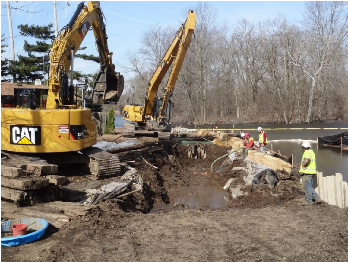
25. Confluence: observed removal of the diversion structure.
