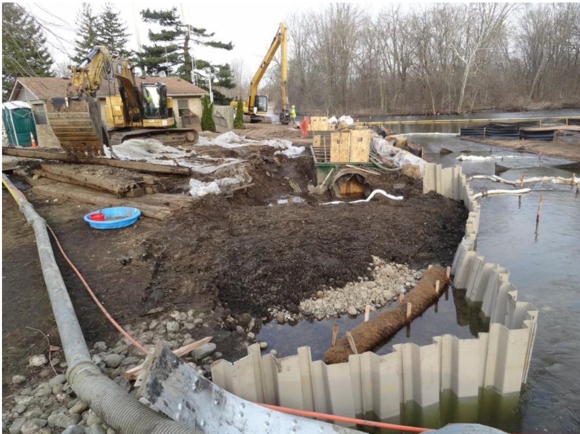
16. Confluence: observed backfill and excavation work around first diversion box.
