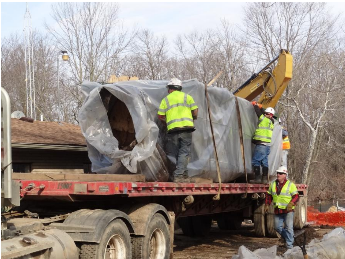
22. Confluence: observed the removal of the first diversion box.
