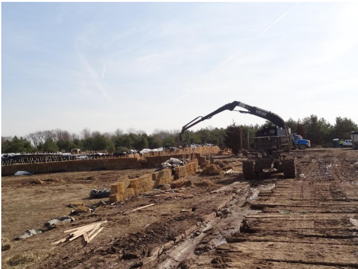
2. Turbidity Control Structure observed being demobilized.
