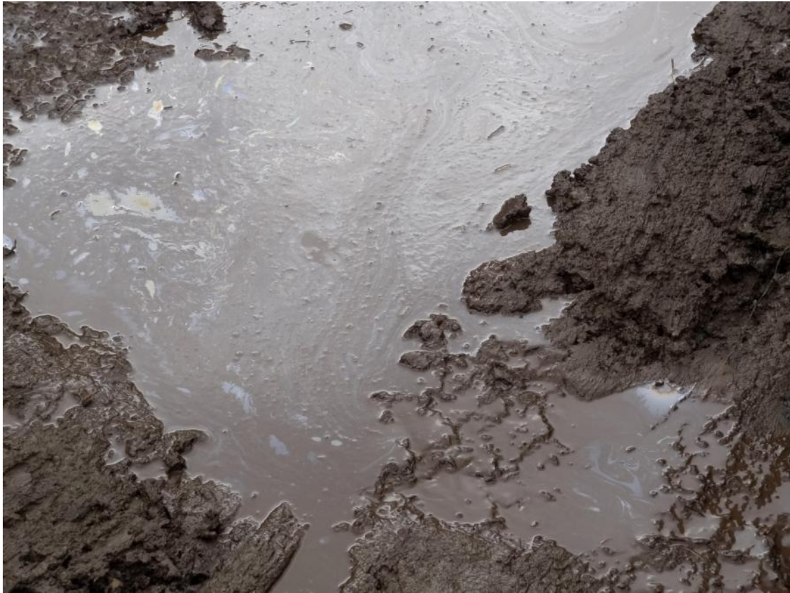
33. Confluence: sheen observed during excavation and removal of the diversion structure.
