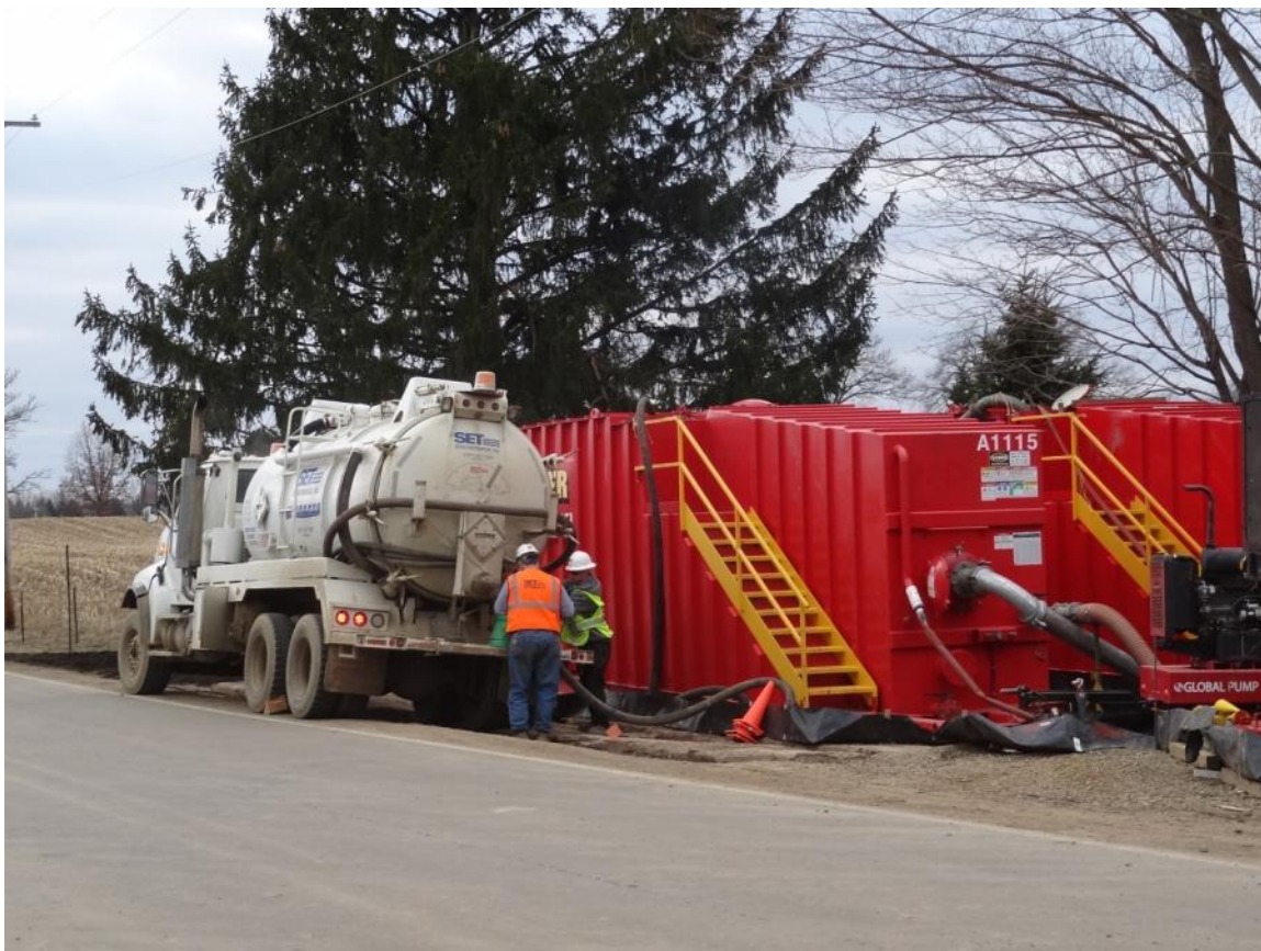
35. Confluence: Vac-truck observed at Frac-Tanks.
