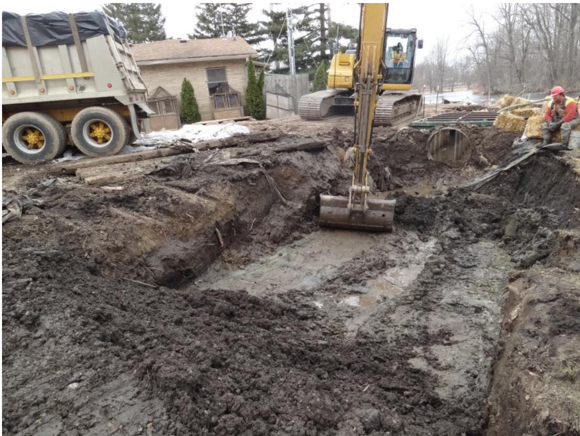
32. Confluence: excavation and removal of the diversion structure.
