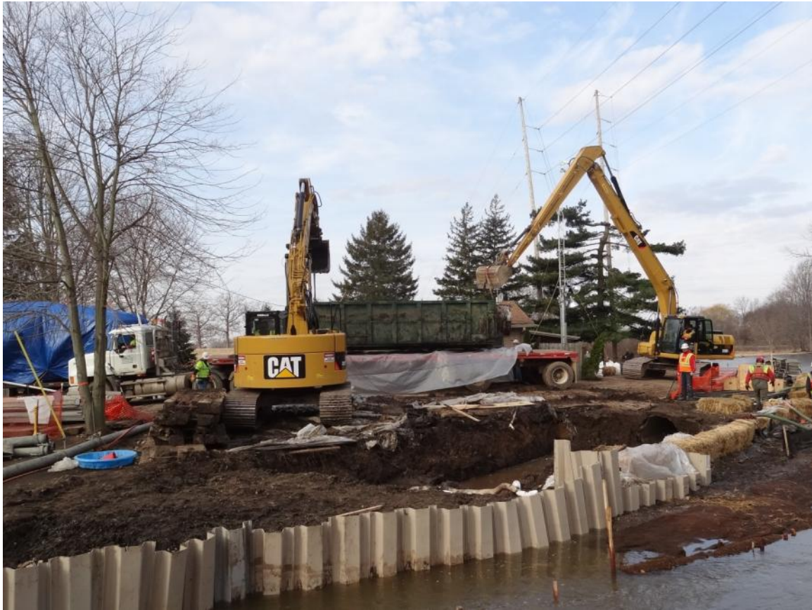
21. Confluence: observed removal of the diversion structure.
