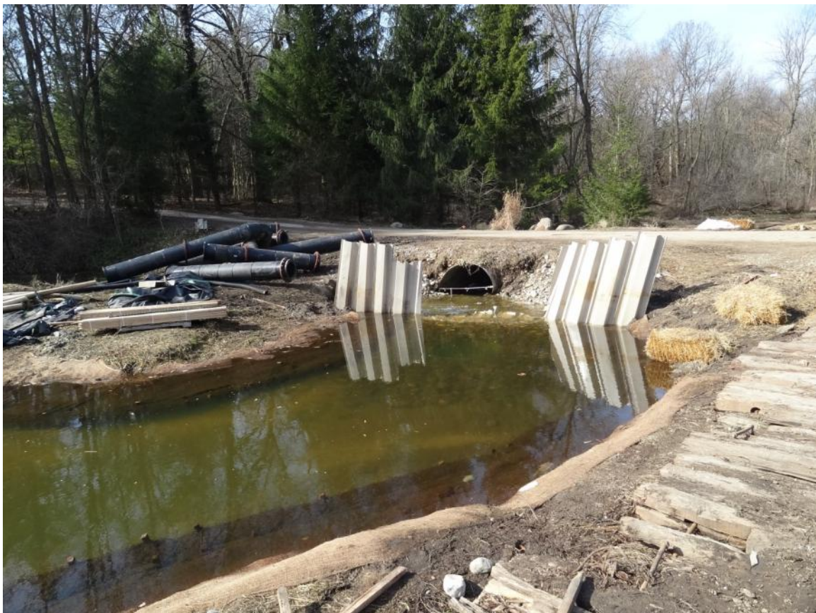
6. Talmadge Creek: weir structure near MP1.6.
