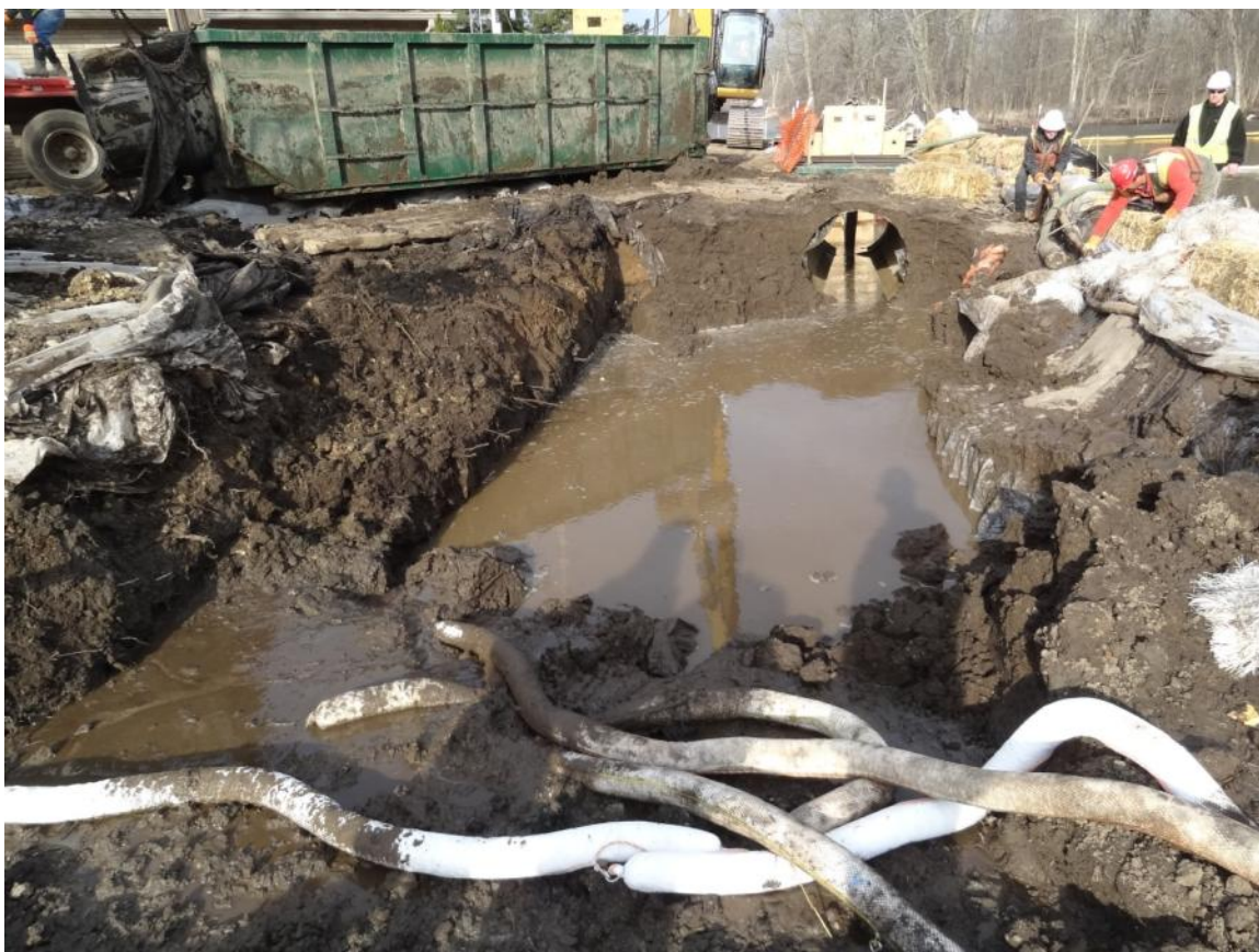
20. Confluence: observed the removal of the first diversion box.
