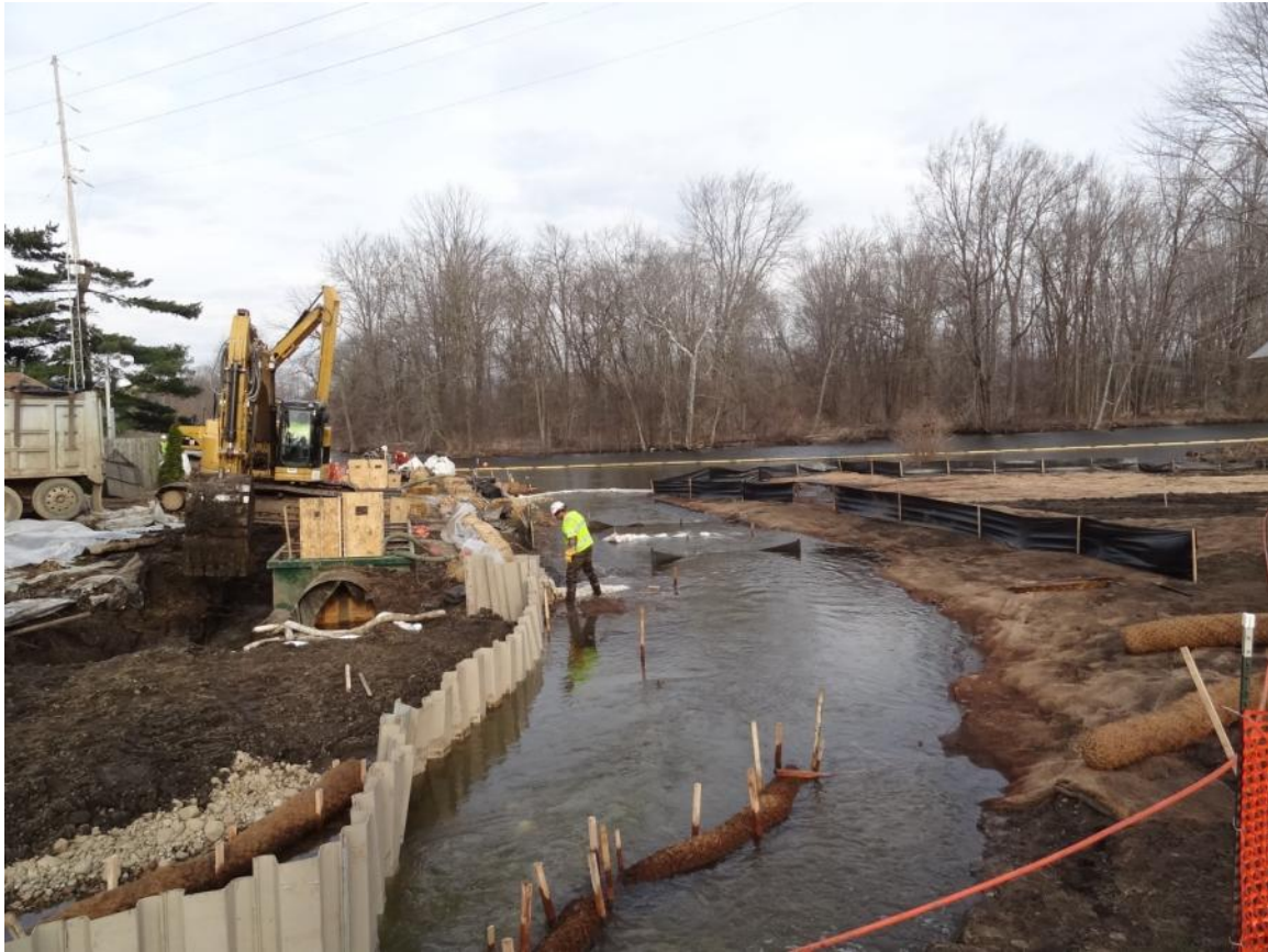
15. Confluence: observed crew removing snare boom and sediment curtain from creek portion of Confluence.
