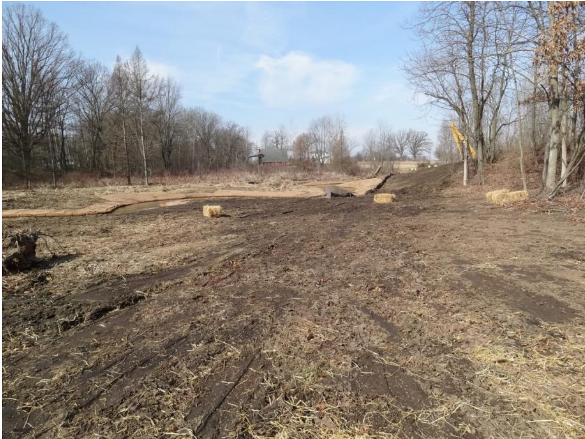
7. Talmadge Creek: timber mats removed and restoration work near MP1.75.
