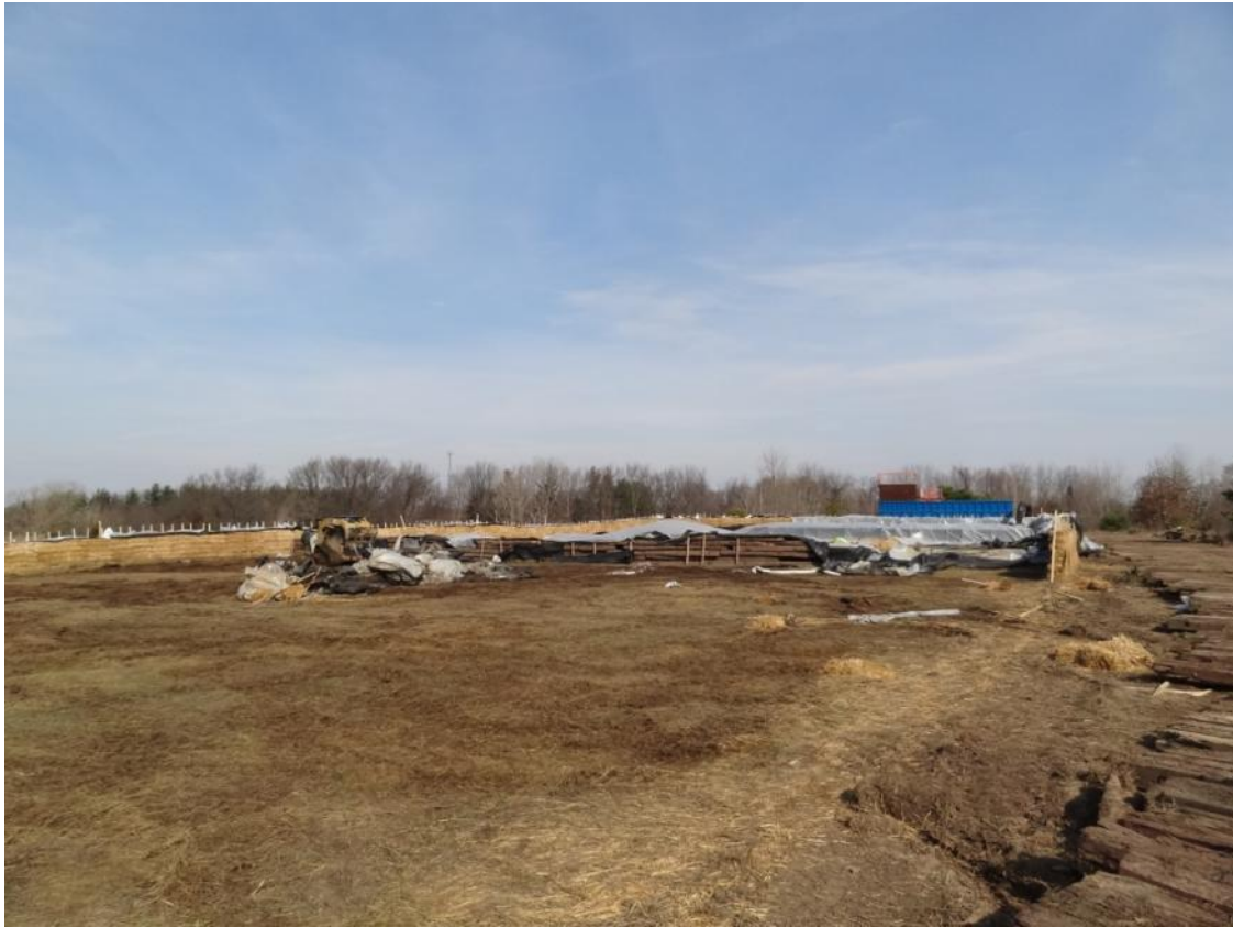
3. Turbidity Control Structure observed being demobilized.
