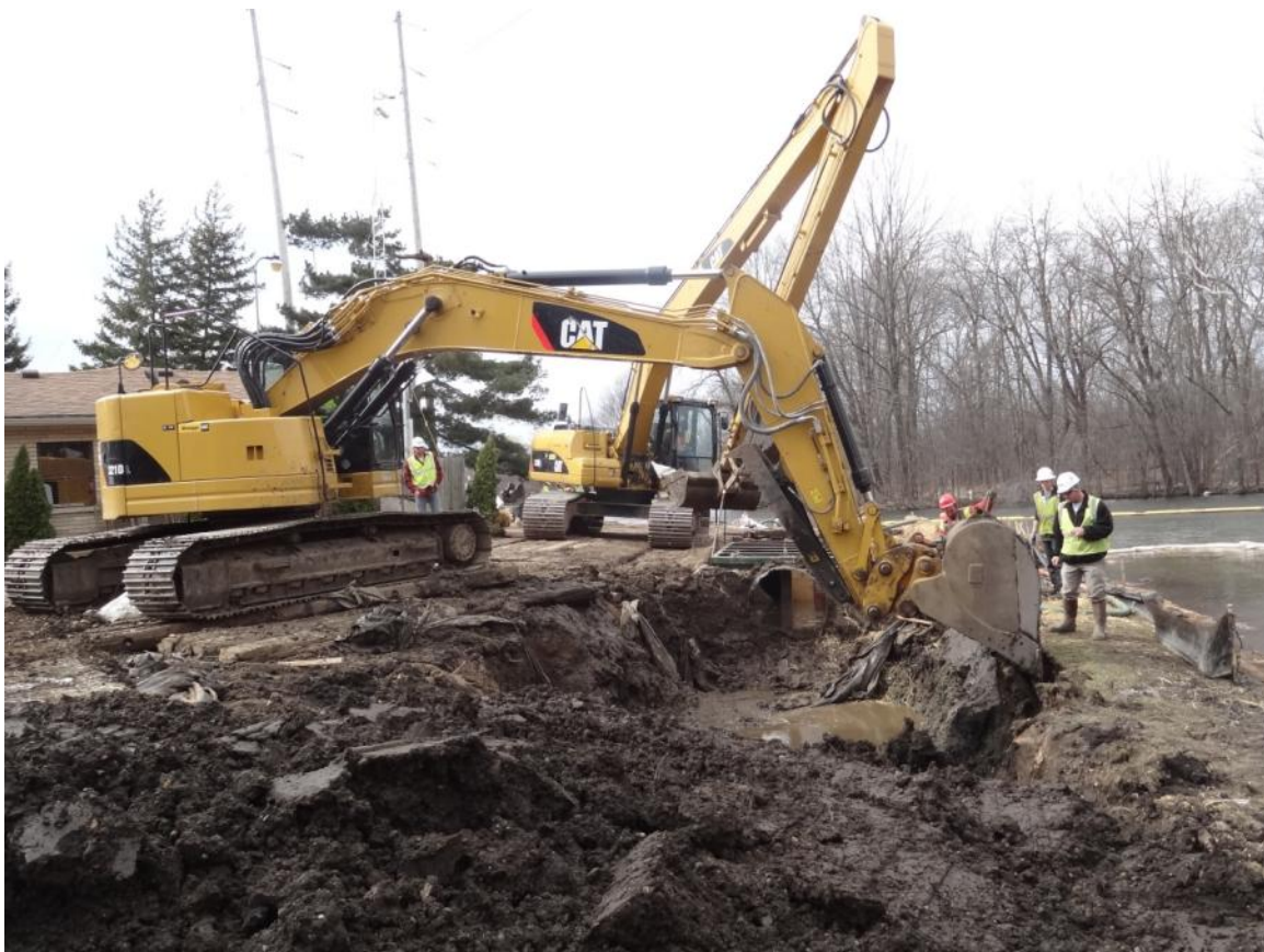
30. Confluence: excavation and removal of the diversion structure.
