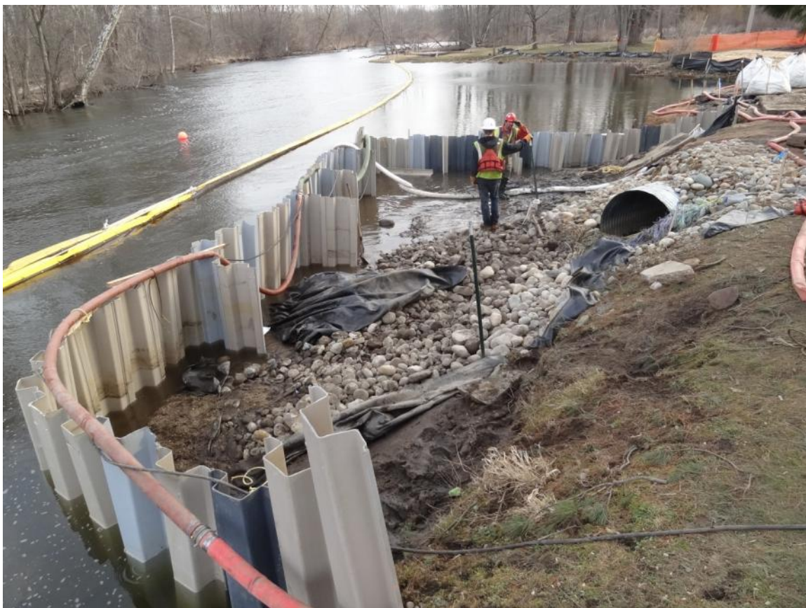
13. Confluence diversion outfall dewatered.
