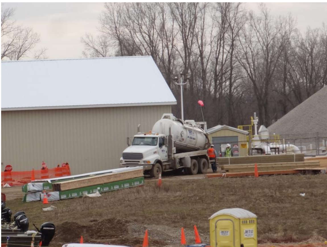
36. Frac-City offloading at pole barn.
