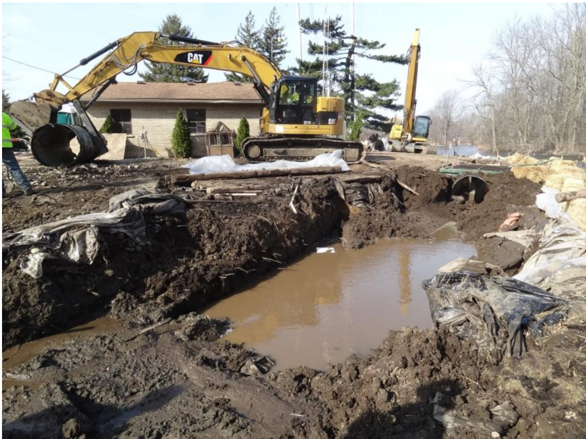
24. Confluence: observed removal of the diversion structure culvert that connected the two boxes.
