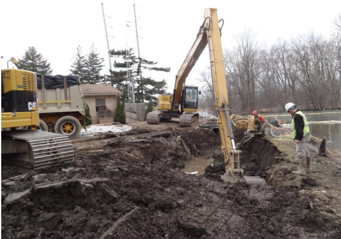
31. Confluence: excavation and removal of the diversion structure.
