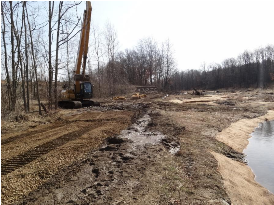
8. Talmadge Creek: timber mats removed and restoration work near MP1.75.
