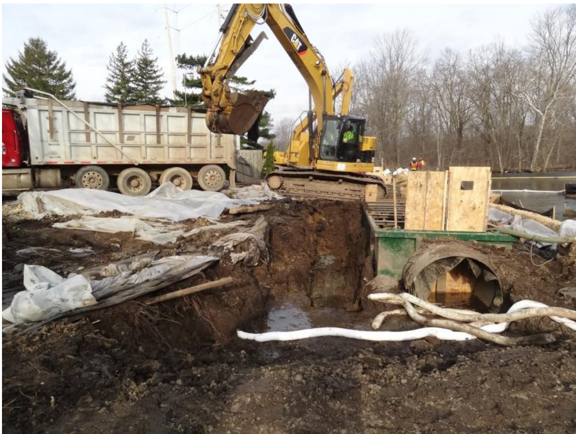
17. Confluence: observed excavation around the first diversion box.
