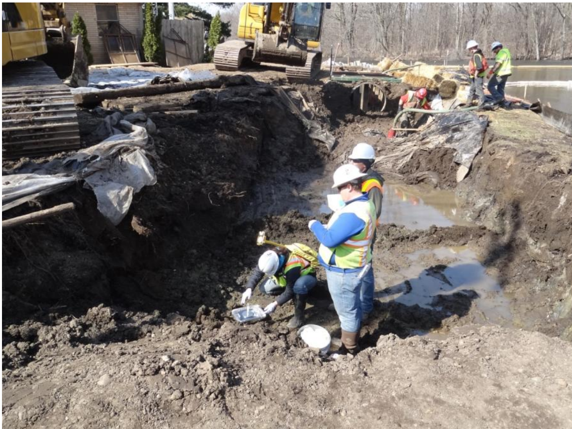
28. Confluence: observed sampling of the excavation prior to restoration.
