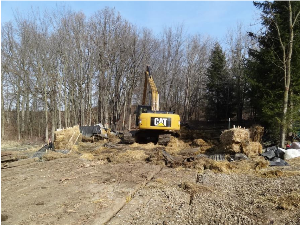
5. Talmadge Creek: demobilizing of bypass discharge near MP1.6.
