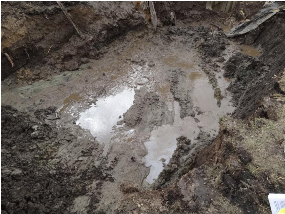
34. Confluence: excavation and removal of the diversion structure.
