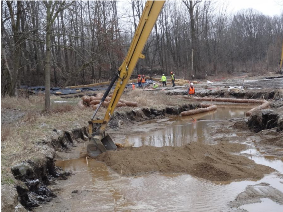
11. Talmadge Creek restoration work near MP1.85.
