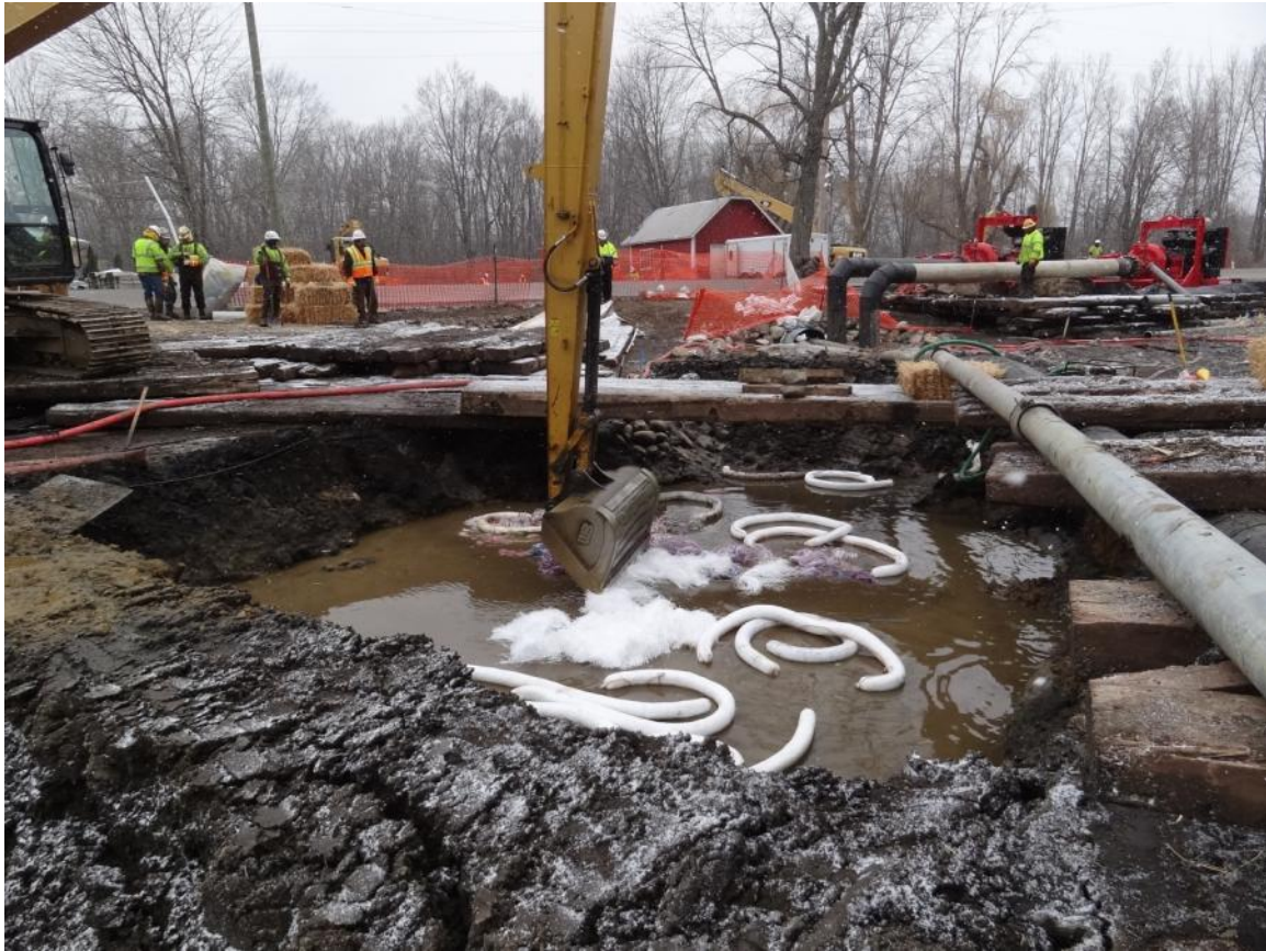
15. Talmadge Creek excavation work near A Drive.
