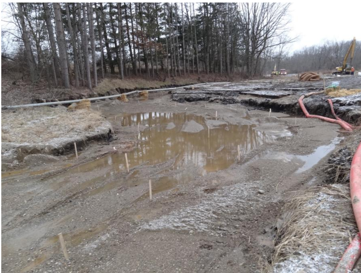
10. Talmadge Creek restoration work near MP1.85.
