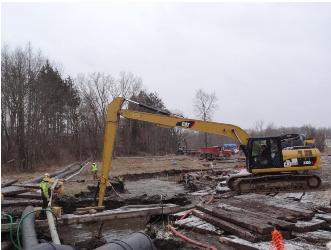
14. Talmadge Creek excavation work near A Drive.
