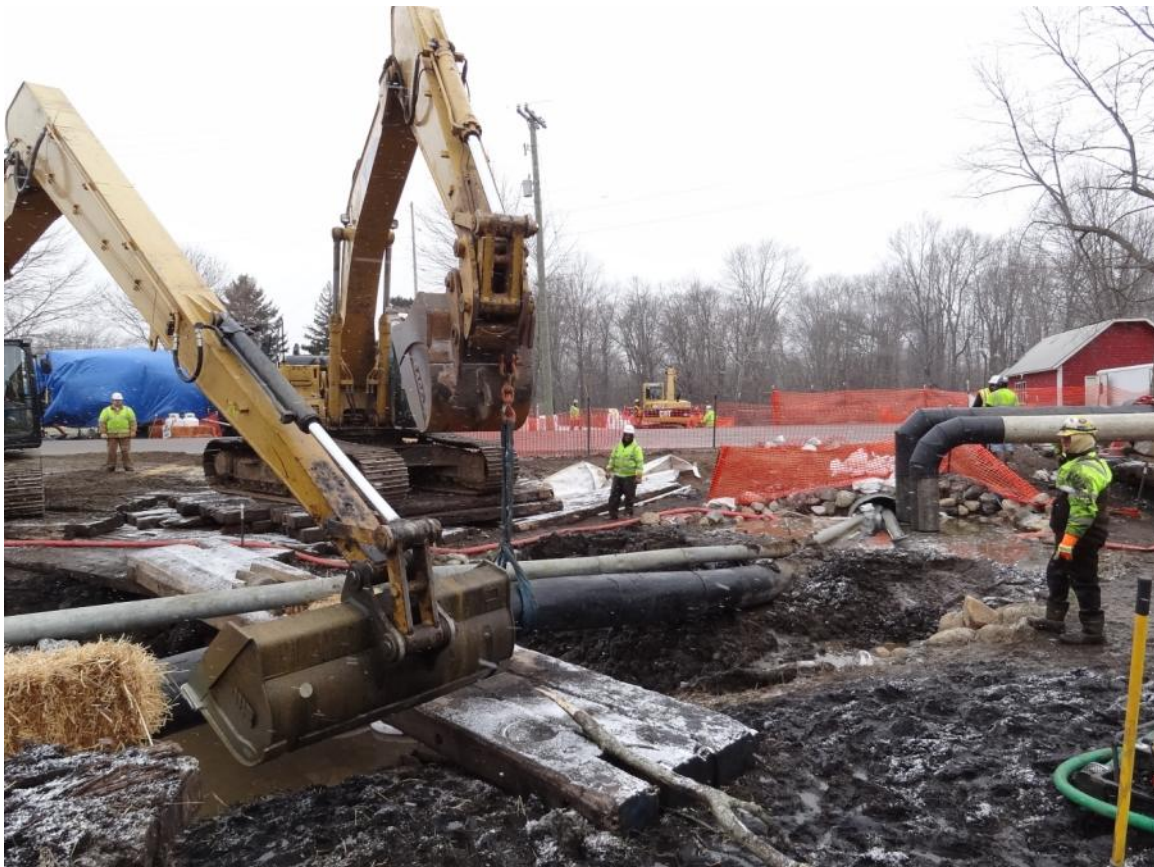
16. Talmadge Creek: observed site prep for excavation work near A Drive.
