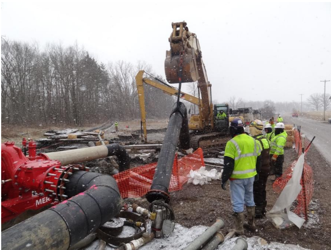
17. Talmadge Creek near A Drive: observed pump being modified.
