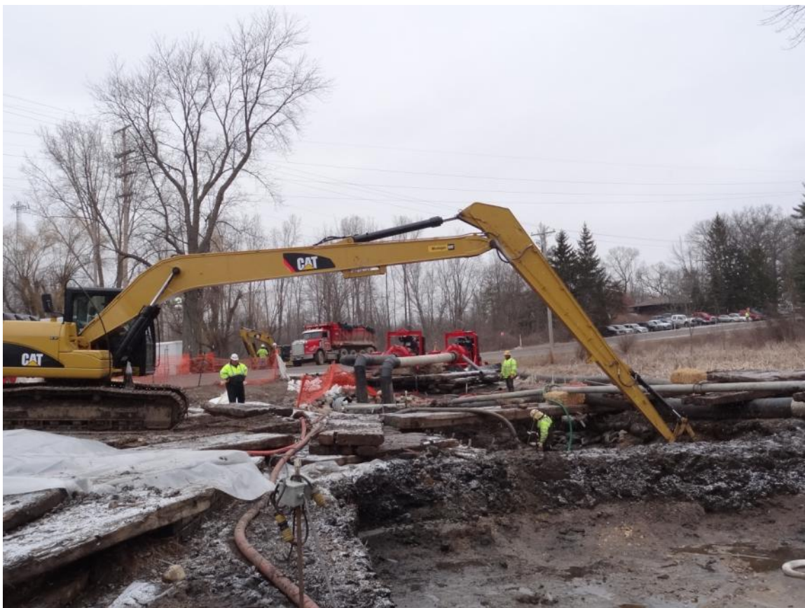
13. Talmadge Creek excavation work near A Drive.
