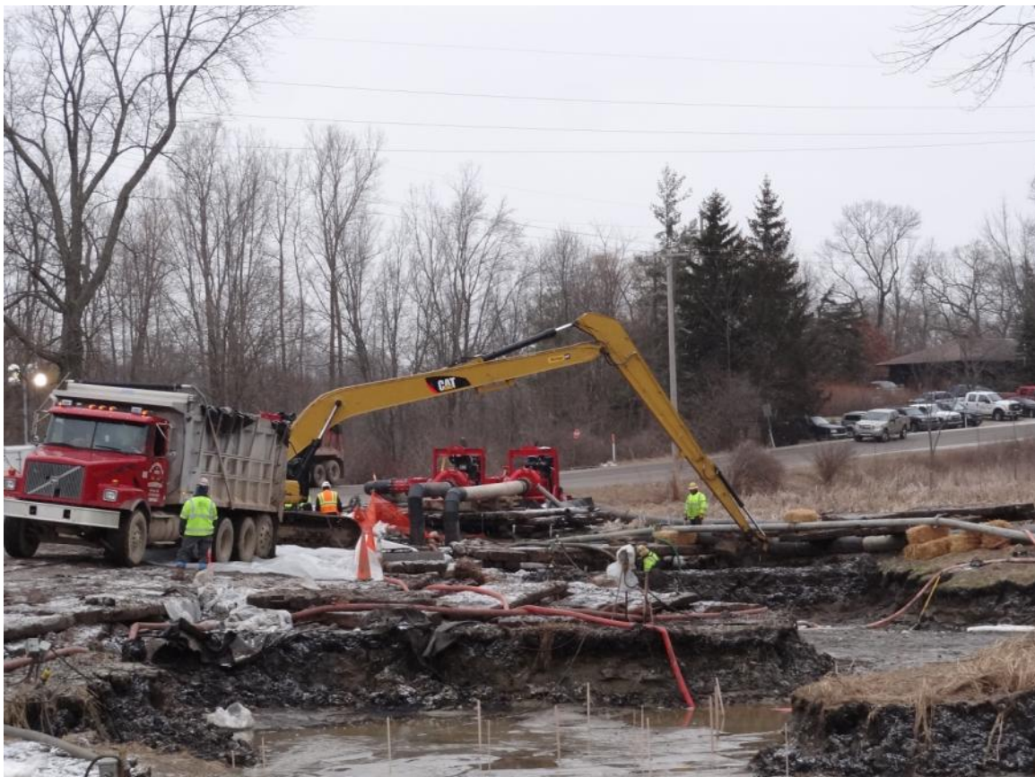
12. Talmadge Creek excavation work near A Drive.
