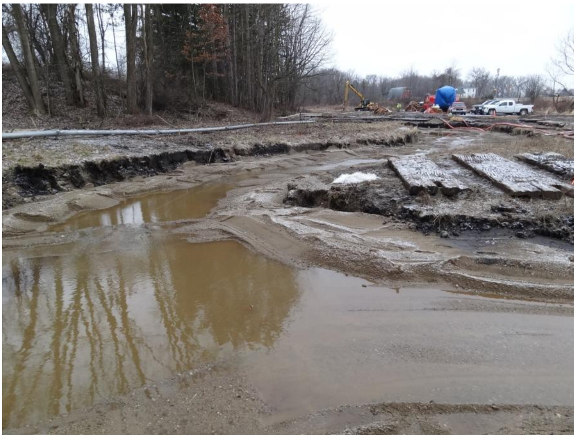
9. Talmadge Creek restoration work near MP1.85.
