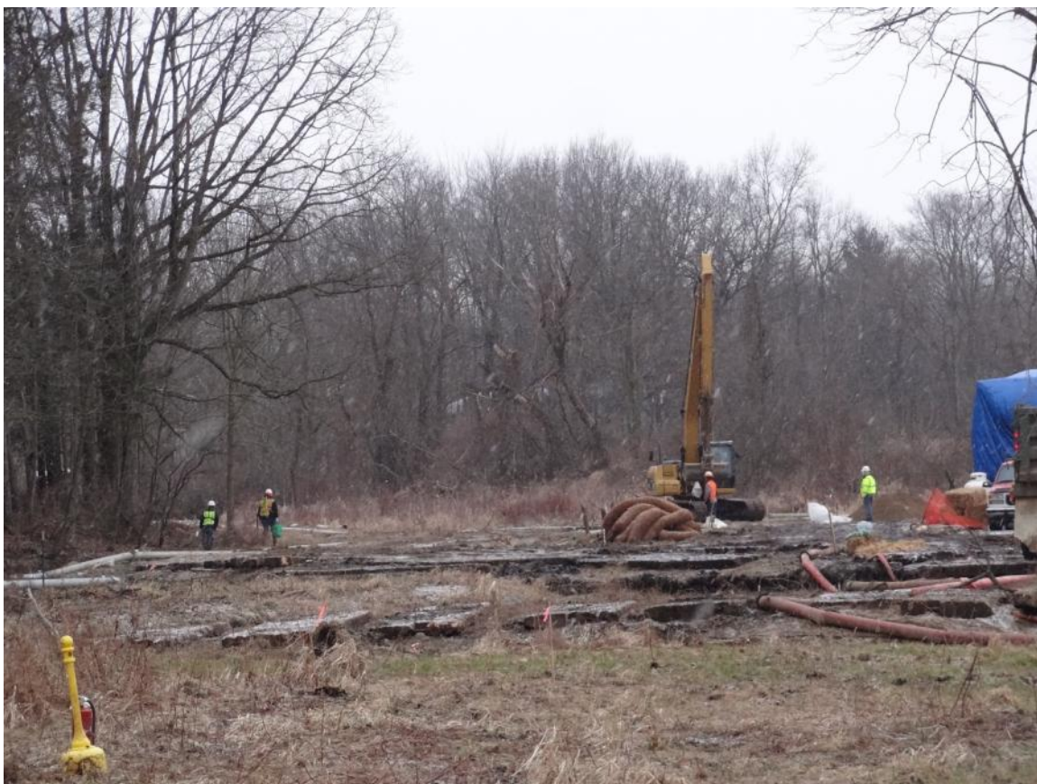
8. Talmadge Creek restoration work near MP1.85.
