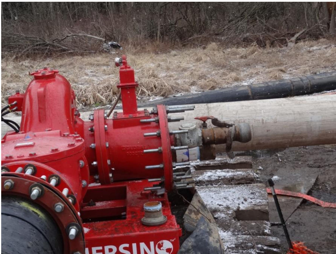
18. Talmadge Creek near A Drive: observed pump being modified.
