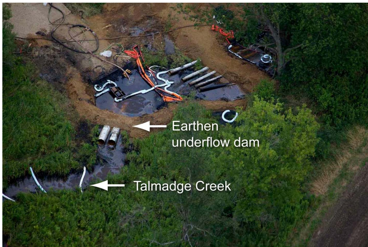
Figure 10. Underflow dam on Talmadge Creek on July 30, 2010.
