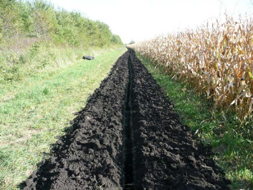
View of lateral distribution line in buffer
