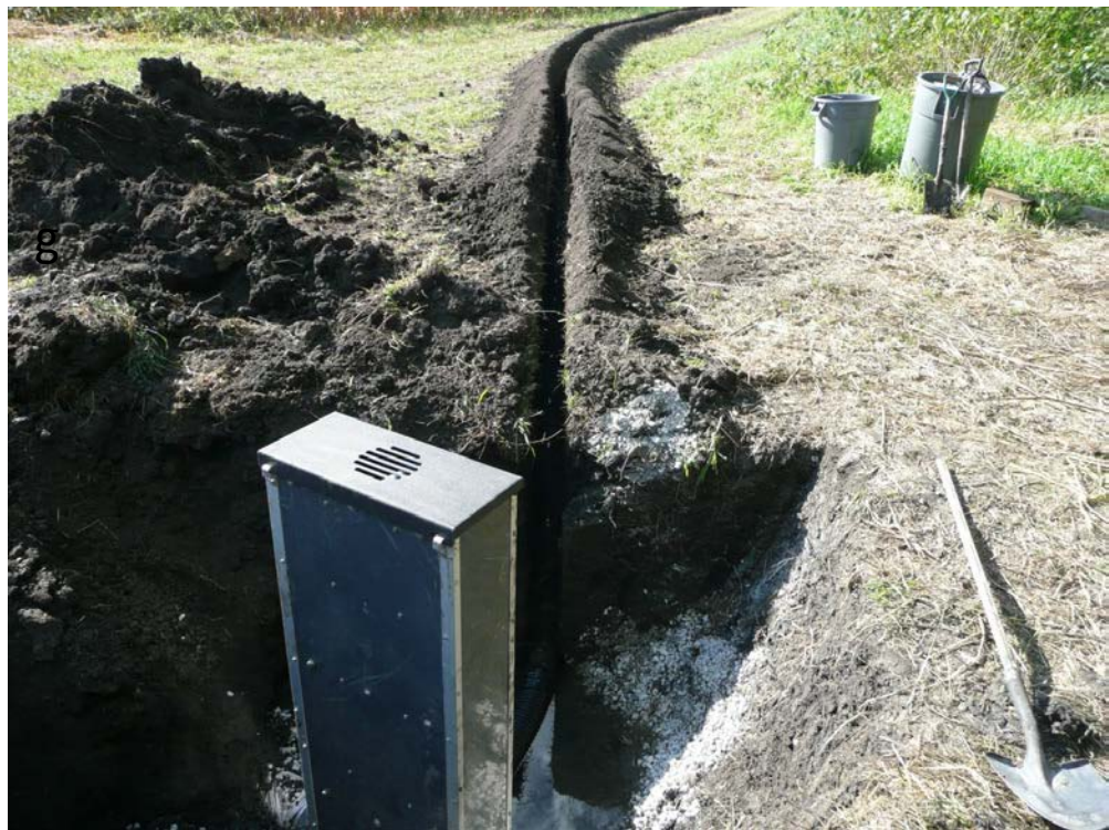
View of control structure installation
