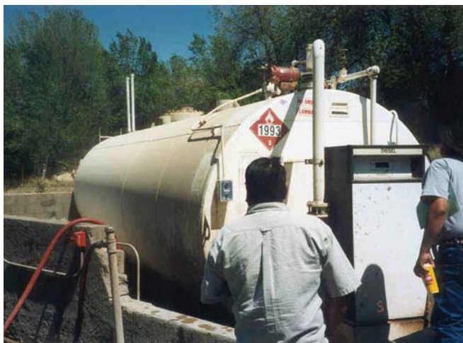
Upper left: Good example of secondary containment.
