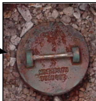
Closeup Of Extractor Port
