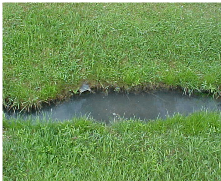
Septic drainage: Preston, KY
