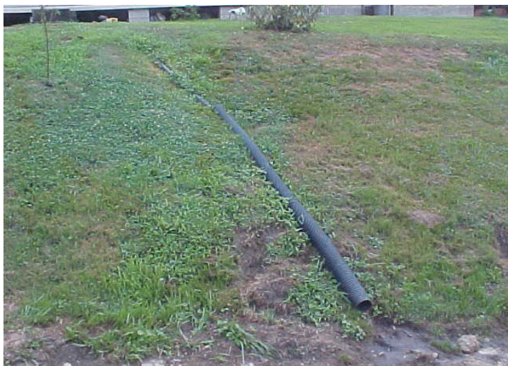
Straight Pipe: Martin County, KY
