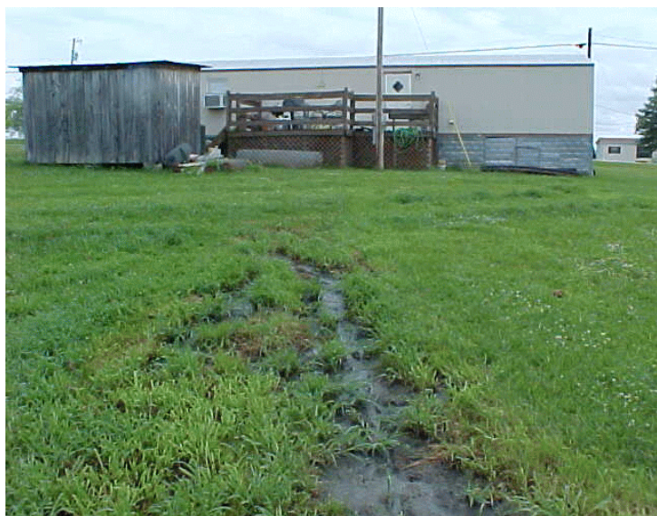
Failed Septic System: Preston, KY
