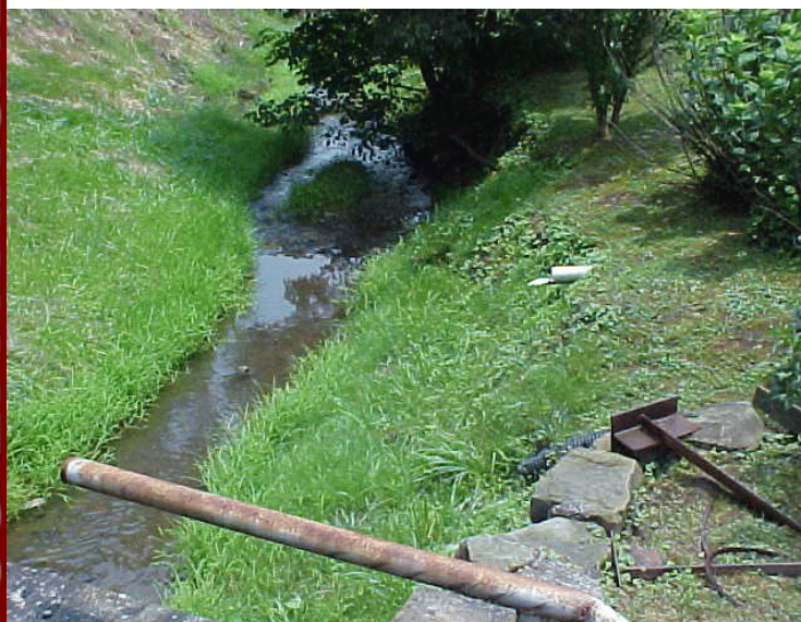
Straight Pipe Discharge: Kermit, West Virginia
