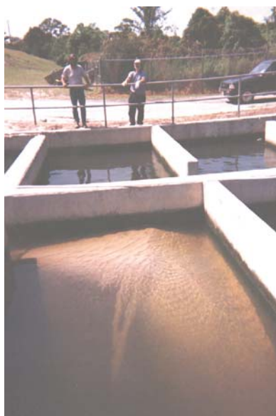
Sand Accumulation in Chlorine Contact Chamber
