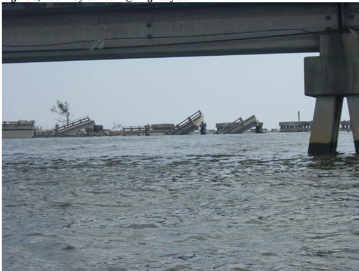
Figure 8, Back Bay of Biloxi @ Highway 90
