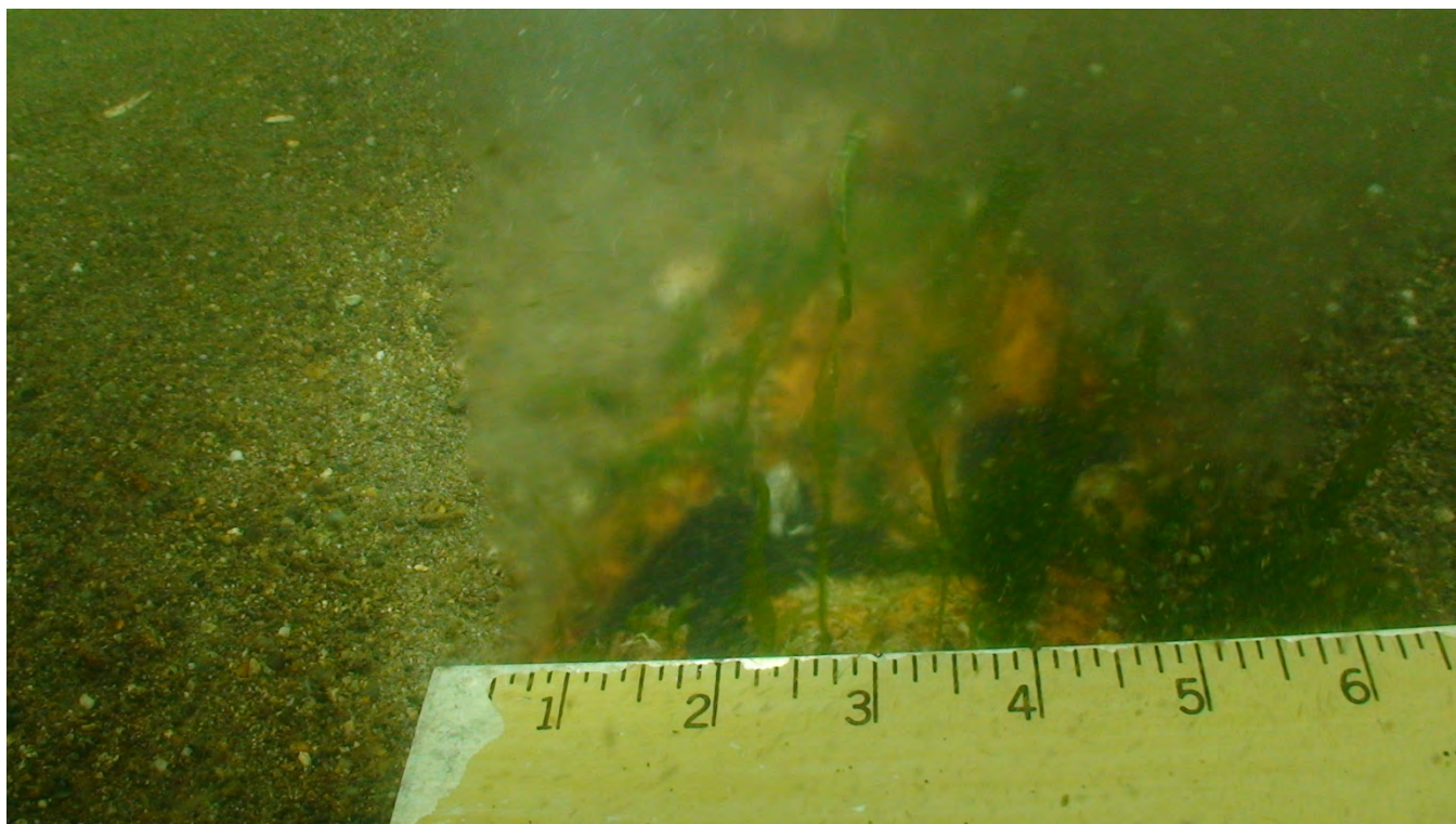
Documenting outfall leakage. Note the freshwater diffracts ambient light differently than the saltwater.
