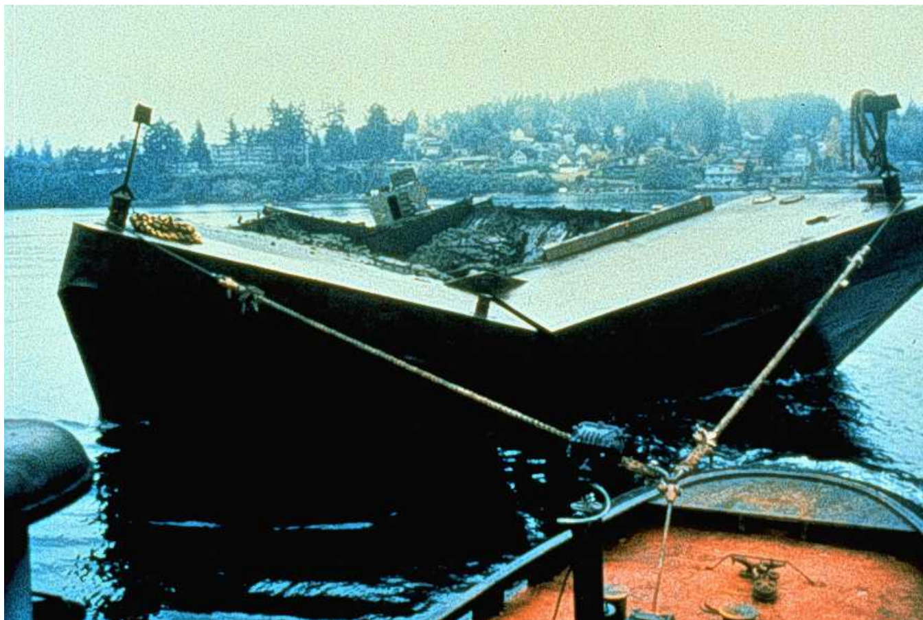
Bottom dump barge placing cap material.
