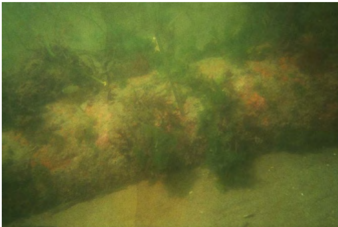
View of algal growth along the treatment plant outfall
