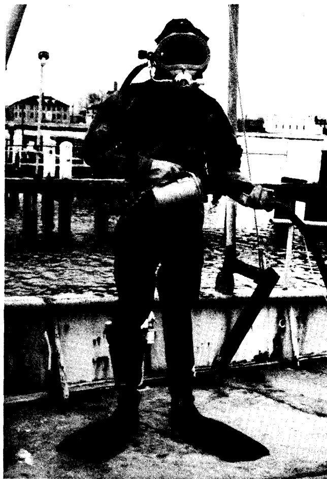
Figure 2. Kirby-Morgan band mask and Viking variable volume suit.
