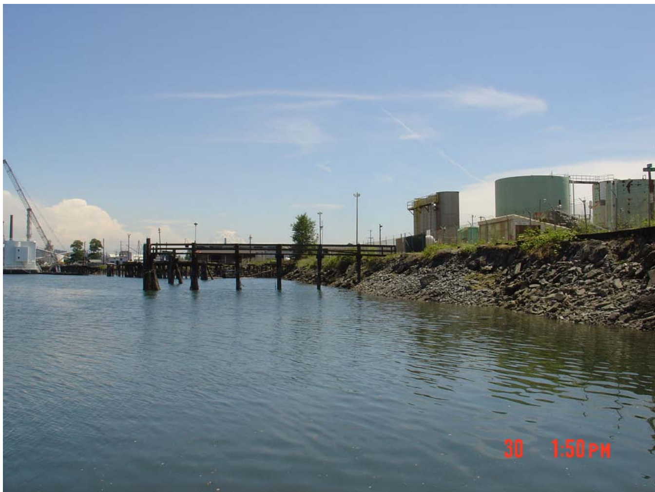
Typical finger pier, rip rapped shoreline, and facility tanks
