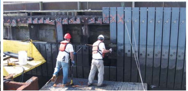
Hydro-Marine workers removing the existing timber fender.
