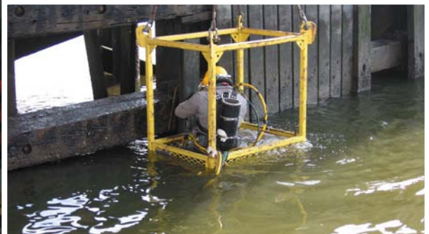
Diver performing underwater work utilizing a man lift.
