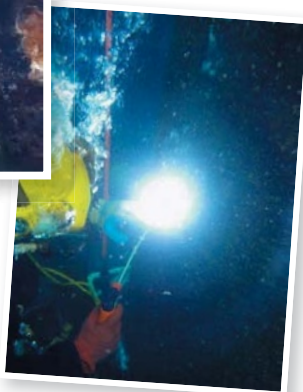
Underwater Jacket Leg Welding Honduras.
