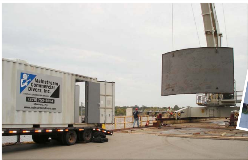
Setting stop logs at a power plant, decompression chamber in conex shown.
