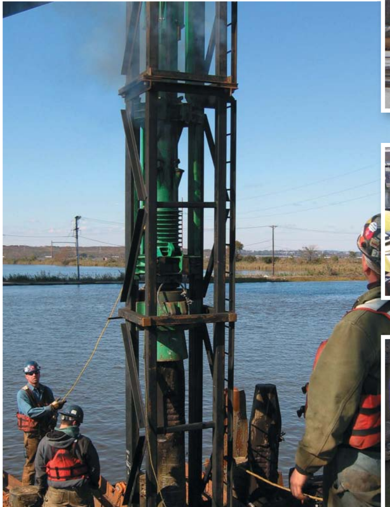
Installation of pile dolphins.
