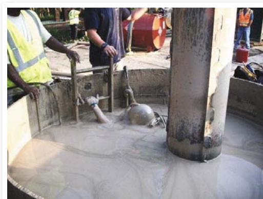
Out of the Mire – An emergency dive to retrieve a 72" drill bit stuck in a 90' deep Caisson filled with drilling mud. Photo taken by Mike Aiken, Owner – American Inshore Divers Corp.
