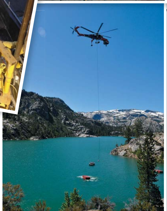
No road into reservoir. All barges and equipment had to be flown in with heavy lift helicopter, CA.
