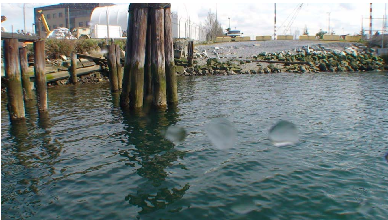
View facing east of a recreational shore access area, just south of the south dock structure.
