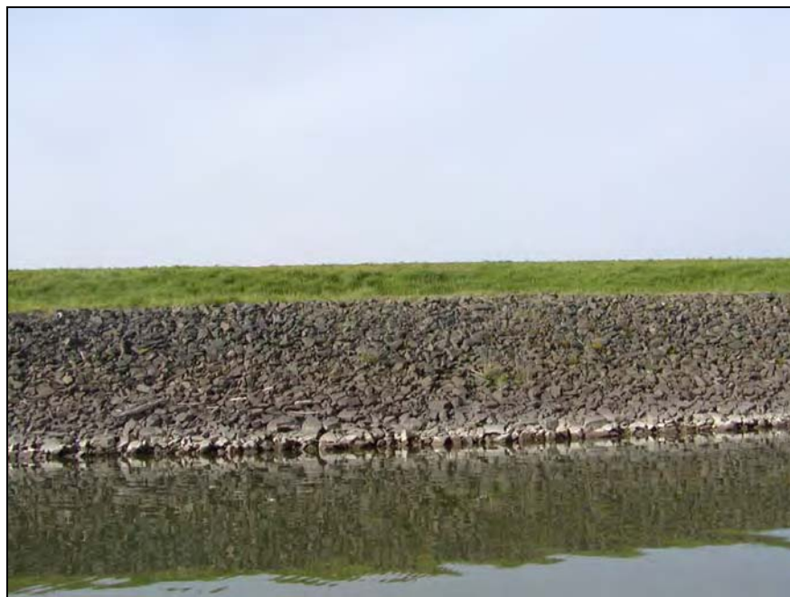
Photo 42. Approximately 0.91 nautical miles downstream from ODEQ GPS Location. Samples DMD-SD-16, DMD-SD-17, DMD-SD-18, and DMD-SD-28. Facing S. 0900 hours. April 26, 2007.
