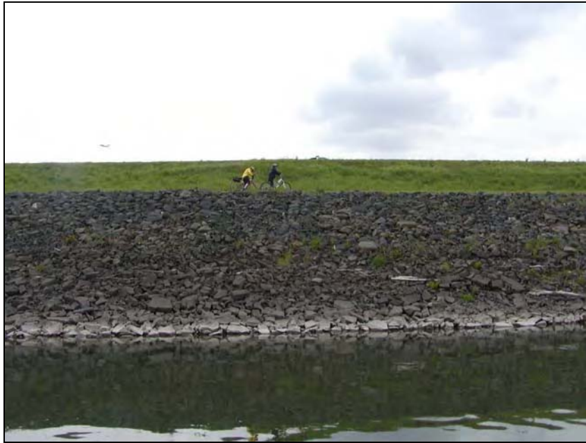
Photo 55. Approximately 0.62 nautical miles downstream from ODEQ GPS Location showing bikers on the bike path. Samples DMD-SD-25 and DMD-SD-26. Facing S. 1410 hours. April 26, 2007.
